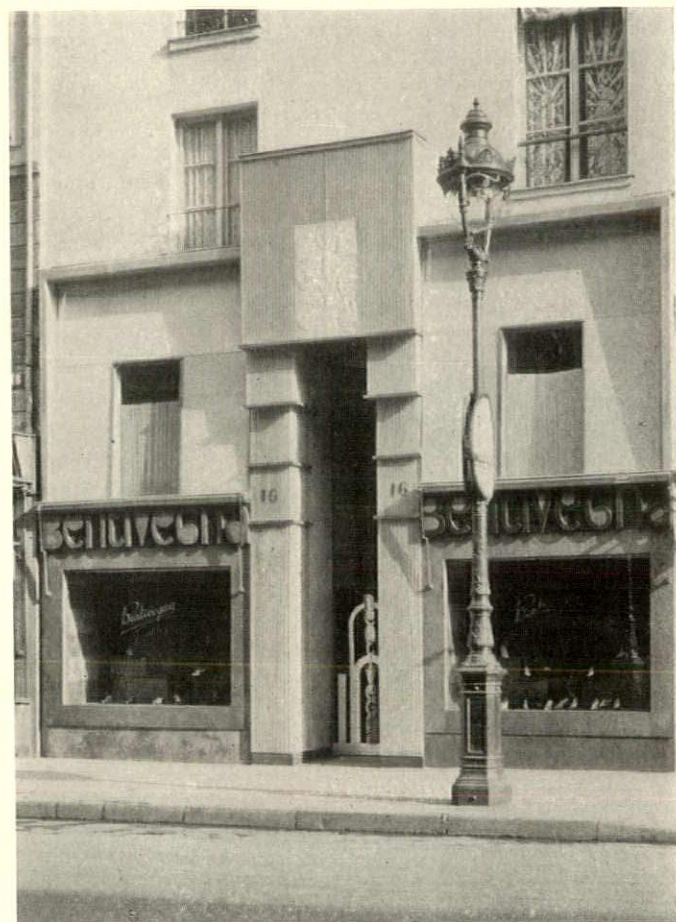
Rue de Faubourg Saint-Honoré. (Maurice Bizet, architect.) This design comprises a versatile union of: two Paris houses with different floor levels, the requirements of an expensive shoe shop, and a design influence imported from perhaps the vicinity of the Nile. The entrance motif is of Nile-green glass ribbed underneath, with an opaque glass panel above the entrance. The show windows have plain facias of mottled gold finish; the window backs have old-gold background and drapes, with the sides in two shades of wide yellow stripes. The base band and signs are lacquer red
