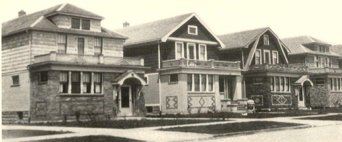
Buffalo, 1931, the second year of the depression. The top story is extended forward to make a full replica of the flat below, but the fact must still be hidden by the draping of a false gambrel-roof effect. The sun-porch appendage is still distinguished by its brick appliqué as the front half of the living-room, tied into the frame half of this room by a fake brick fireplace, on each side of which is the small window over the proverbial book shelves
