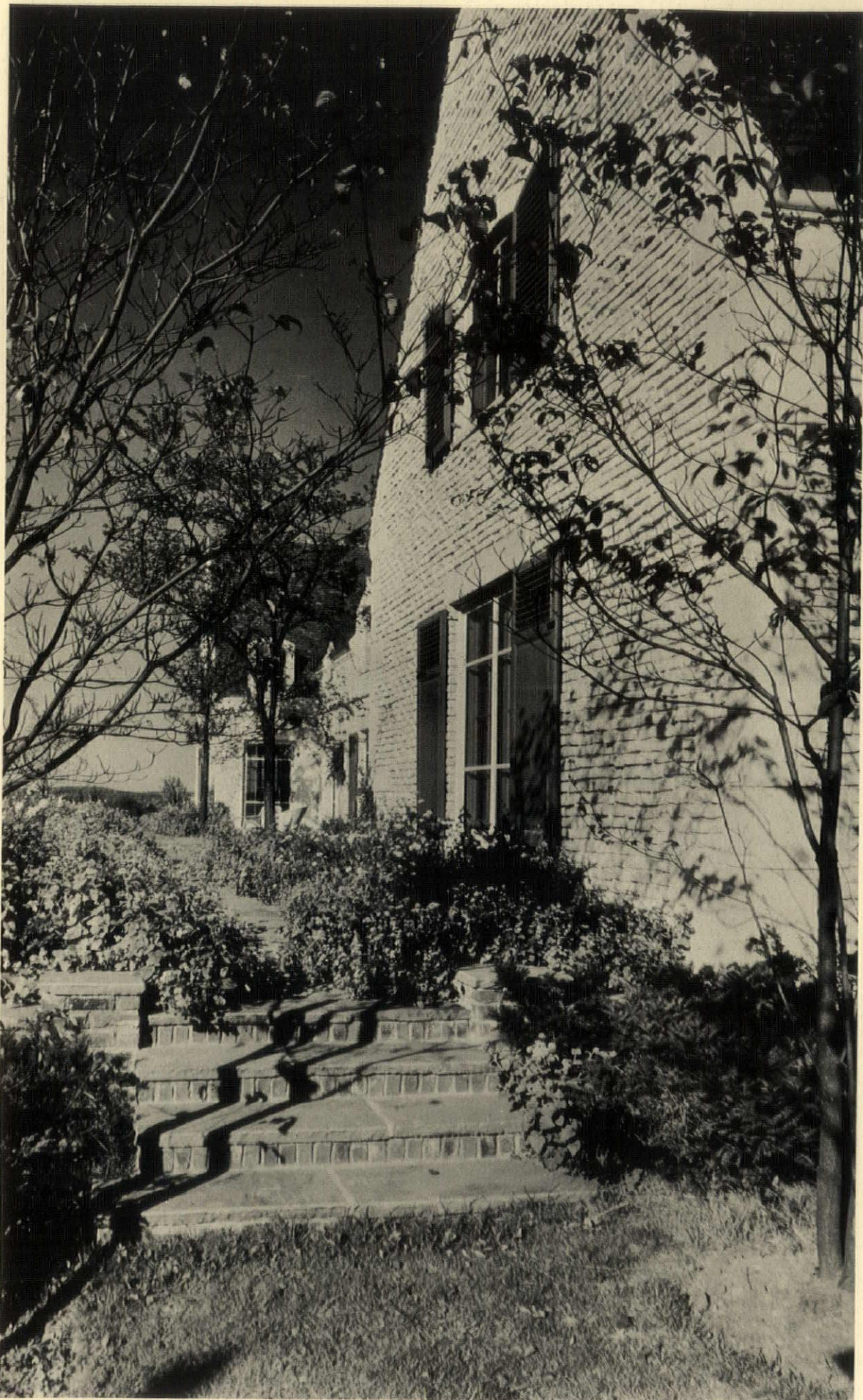
A view taken sharply across the terrace front. For the garden walls, brick capped by flagstone has been used. Shutters are blue-green, woodwork white. Wood casements are used throughout
