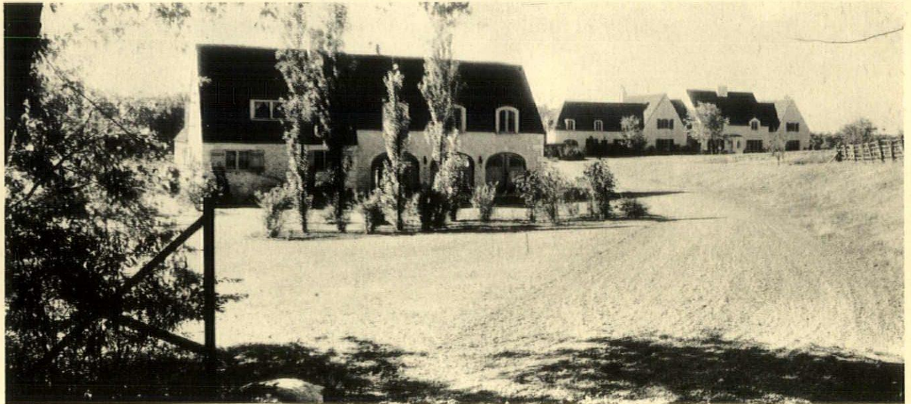
The building in the foreground is the garage, built throughout of the same materials as those used in the house itself
