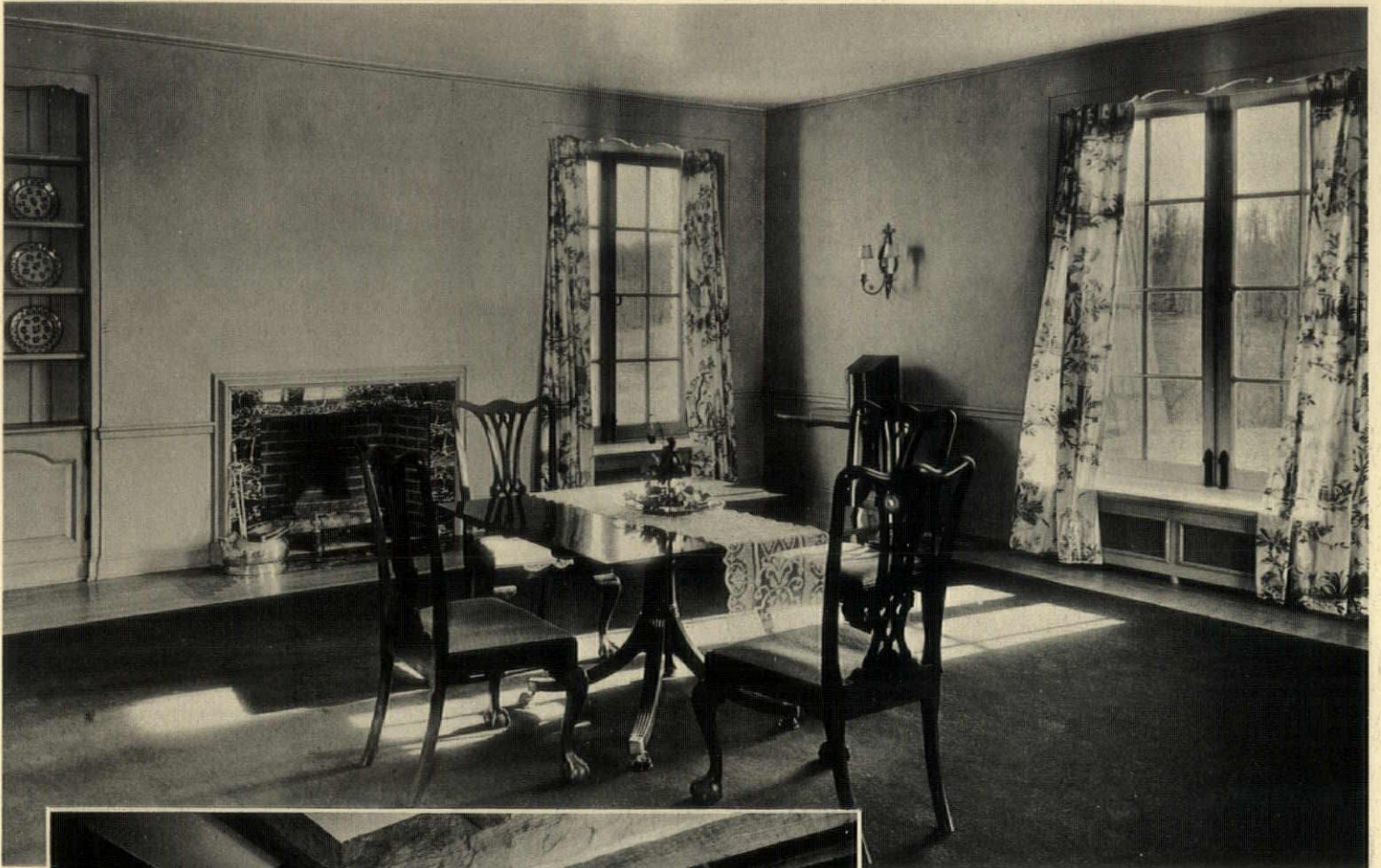
In the dining-room the plaster walls and the woodwork are painted. There is an interesting detail here in the sawn window heads, made to cover the curtain rods. The radiation is concealed under the broad window sills
