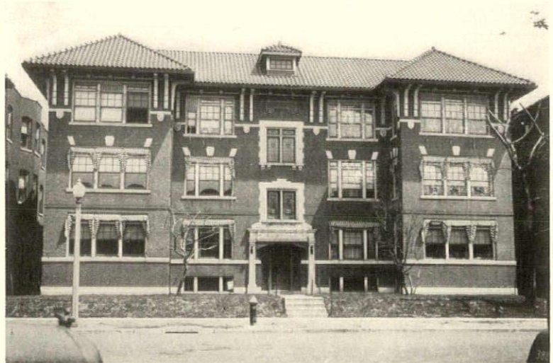
St. Louis, 1925-1930—the expansion of the widened tree-story double flat to the high-rent field, in which an interior court is introduced to form a “U” plan, still with the narrow side yards. Chicago followed suit with about 170,000 dwellings
