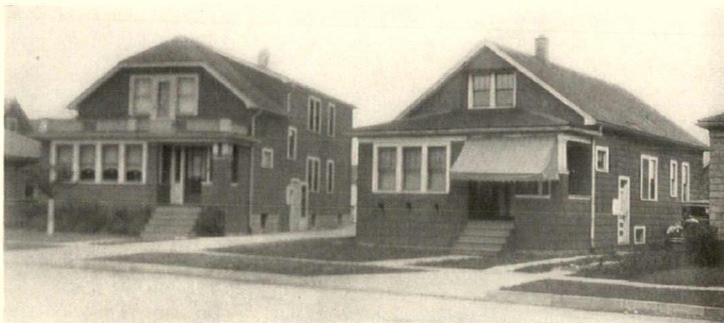
At right, the 1929 Buffalo bungalow. Next door to it is the next step of 1930-31—the "investment bungalow," with an annex on the rear attic for a sub-tenant. The living room of the lower unit is crowded forward into what had started as a sun porch
