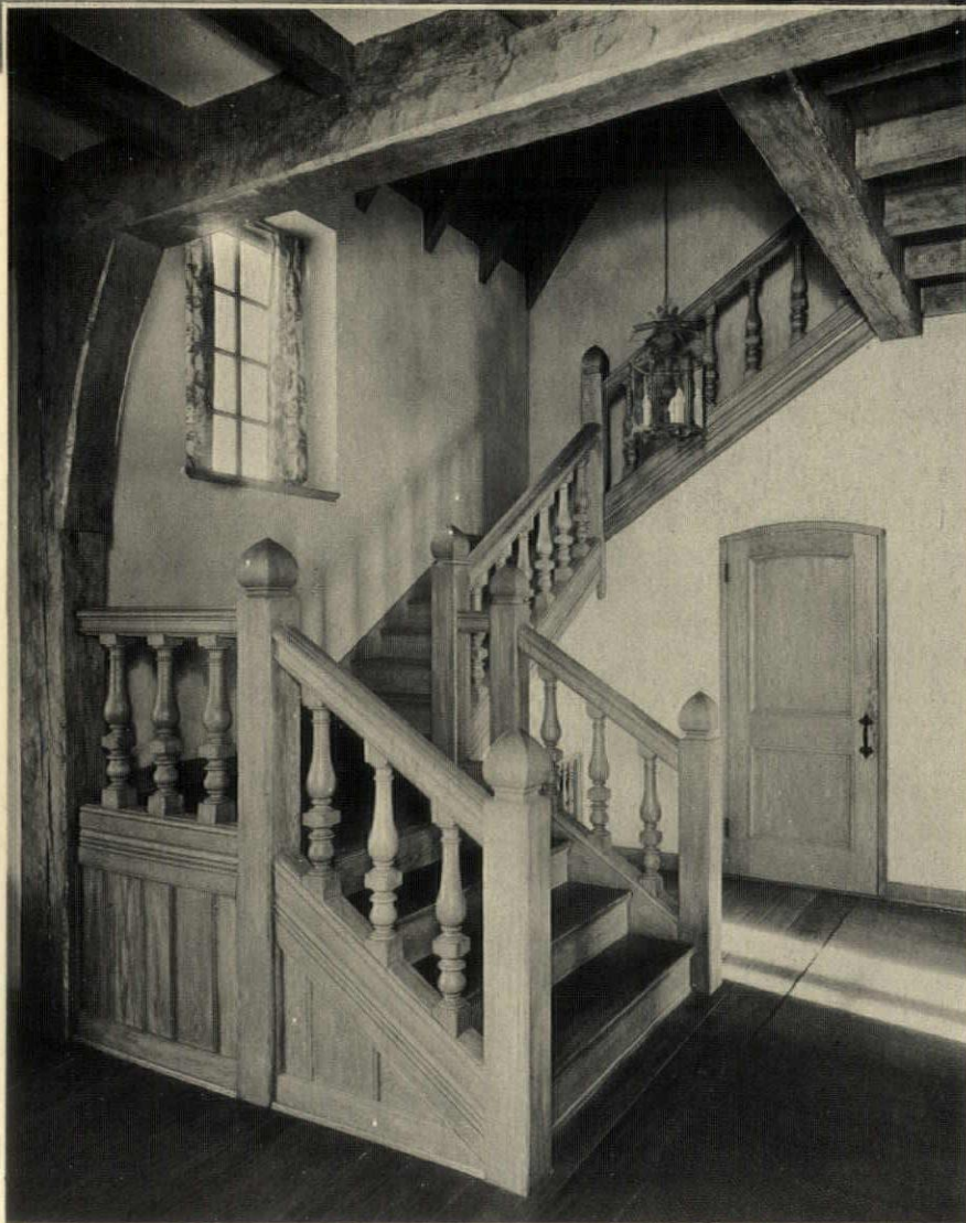
Detail of the main stairway, entirely of oak. The millwork has been given a very light stain as compared with the darker one of the rough-hewn timbering
