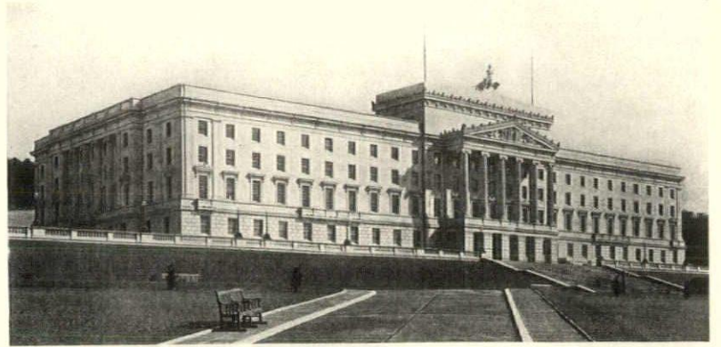
The new Parliament Buildings for Northern Ireland, built of Portland stone on a granite base. Sir Arnold Thornely, architect
