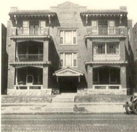
St. Louis, 1915-1925, extended the double two-family dwelling upward to three stories, retaining the tandem layout and adding porches
