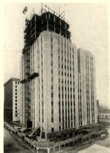
Progress of the work on October 30, 1931
