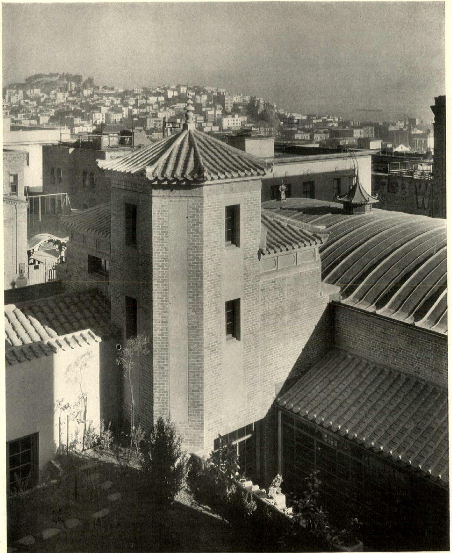
Detail of the east tower and roof composition. The nearer roofs are of handmade tile, the walls of brick and cast stone
