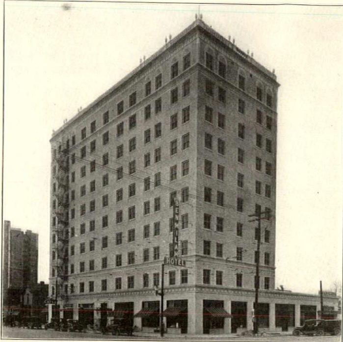
HOTEL BEN MILAM, HOUSTON, TEXAS JAMES RUSKIN BAILEY, ARCHITECT CALKED BY A. M. BOWLES, HOUSTON, TEXAS
