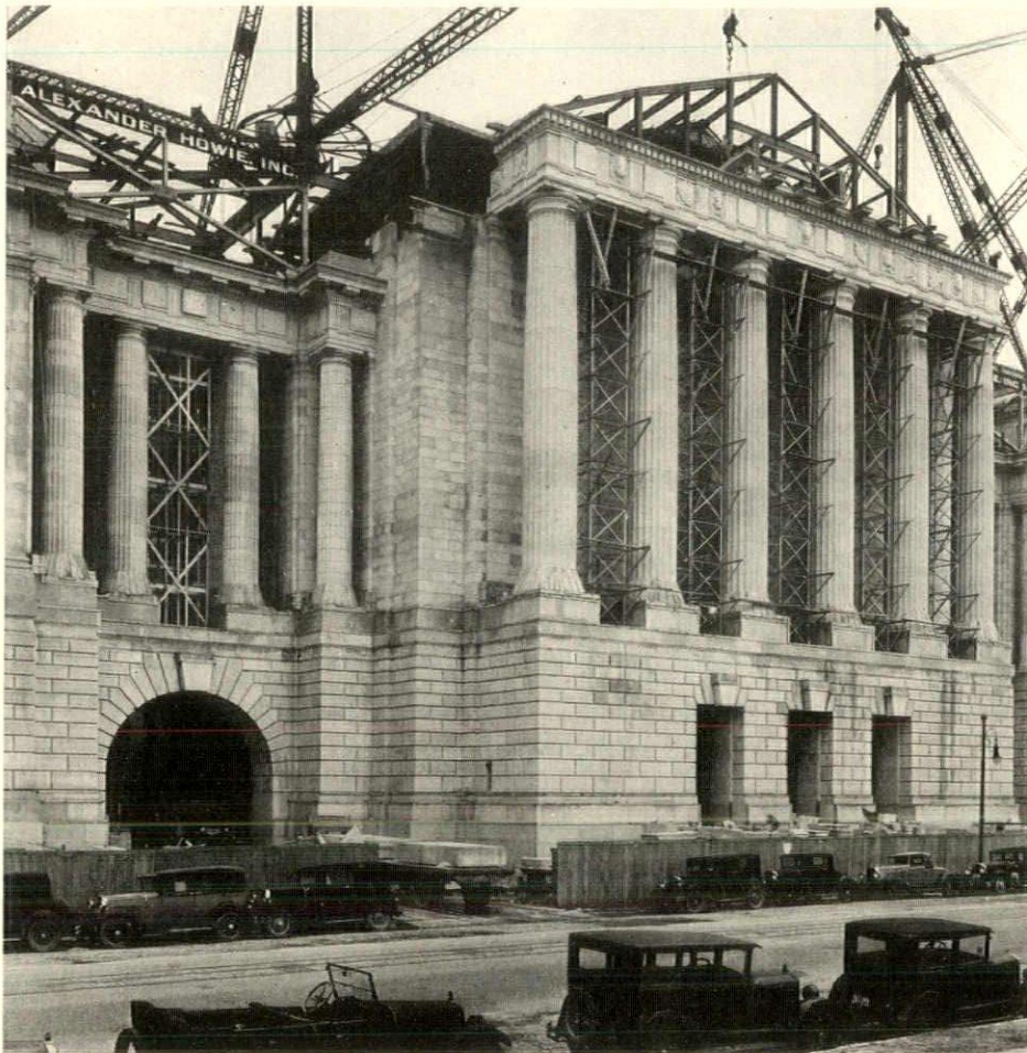
A recent progress photograph of the central portion of the above
