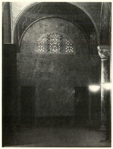
the stone, at right angles to its natural bed. This cutting brings out veins instead of the clouds that appear when such a stone is cut with the grain. The thin slabs between the grilles were sawn about 5% in. thick, then rubbed down to 3% in. and polished. The parts are firmly joined together with a transparent cement.
