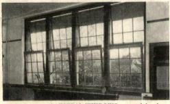
A typical group of AUSTRAL WINDOWS as used in cla rooms; ventilation at center without direct draft.
