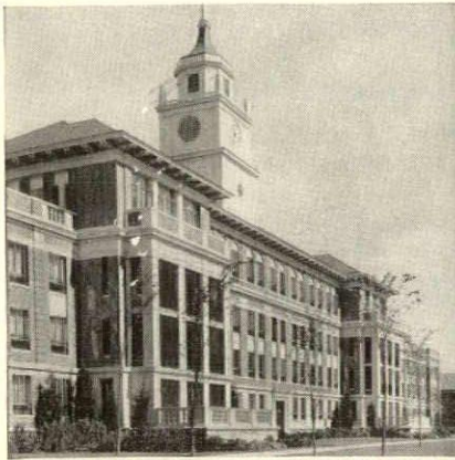
MIDDLESEX COUNTY SANATORIUM, WALTHAM, MASSACHUSETTS. Byers Genuine Wrought Iron specified for concealed waste lines, vents, gas and back air piping; also for heating supply and return lines.
