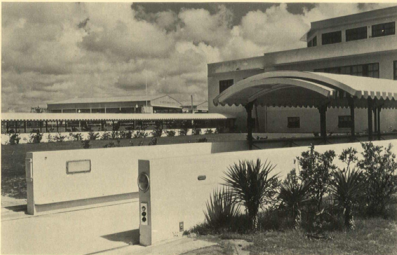
End of a passageway leading to the planes. Note the sliding canopy roof extension
