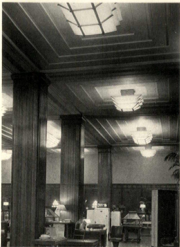
A detail in the showroom of an electric light company in Allentown, Pa.—another example of combination lighting, with the luminaires close to the ceiling
