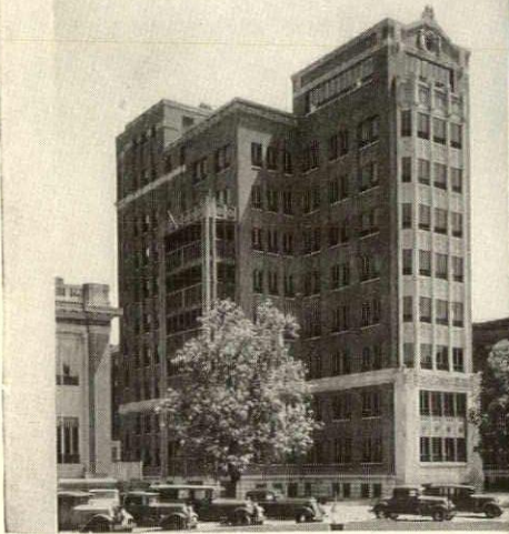
PEDIATRIC BUILDING, BOSTON CITY HOSPITAL. Byers Genuine Wrought Iron specified for concealed waste lines, vents and gas piping; also for heating supply and return lines.
