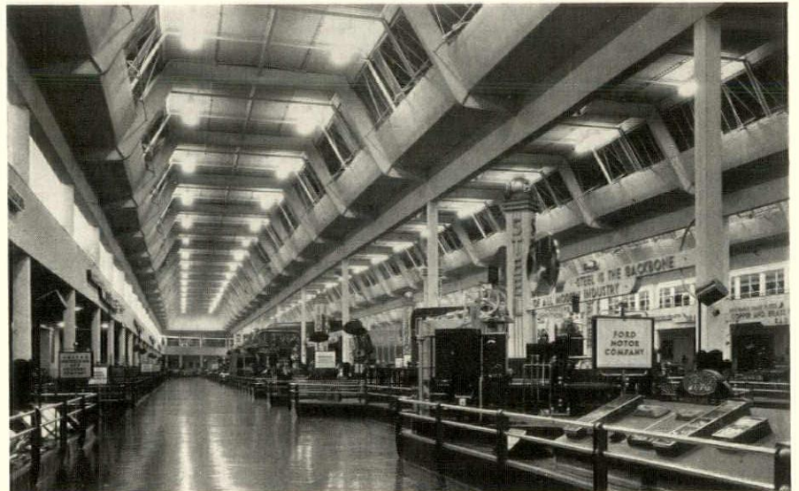
The Ford Motor Company's Building at A Century of Progress Exposition, where an approximation of daylight was produced by high-intensity mercury vapor lamps combined with incandescent lamps. Albert Kahn, Inc., architect
