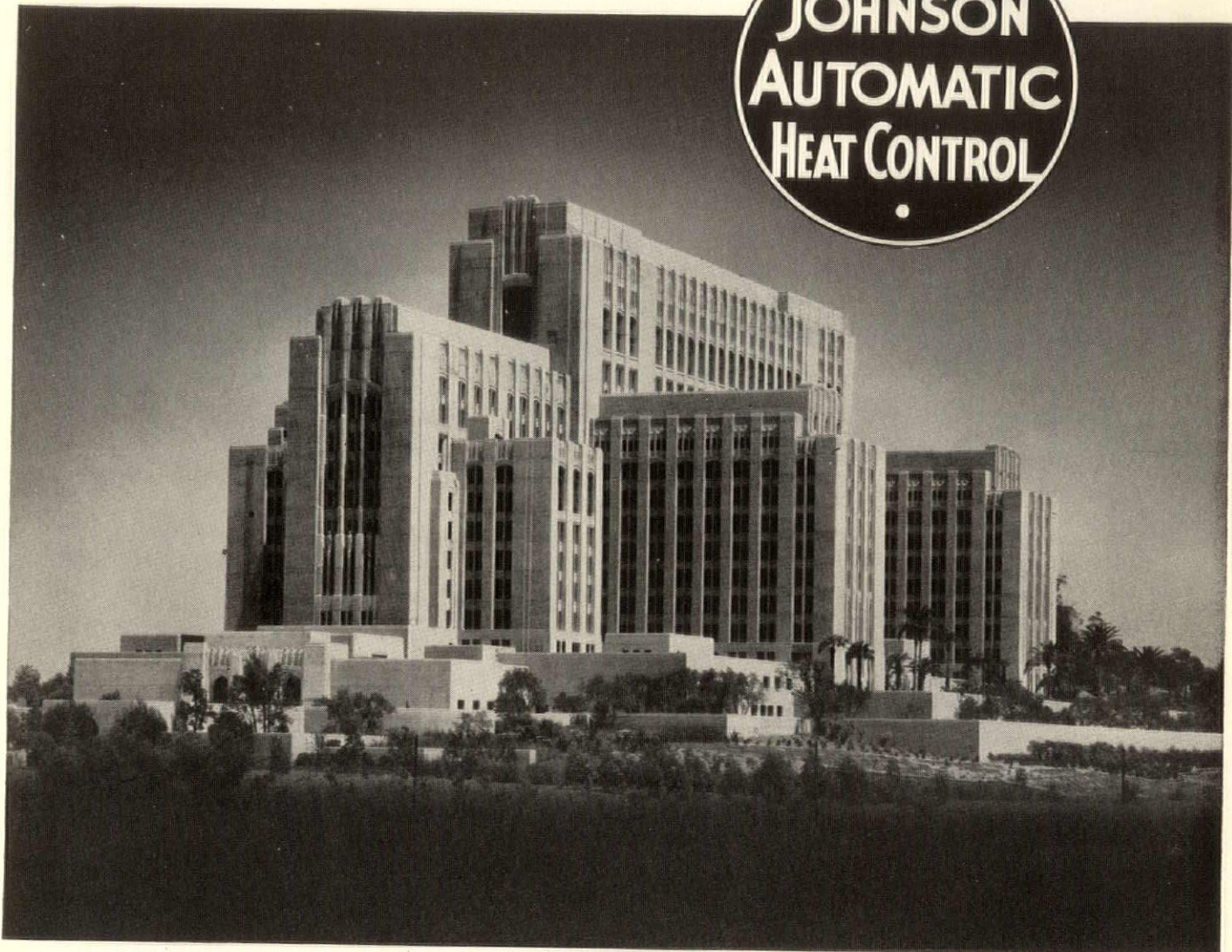
LOS ANGELES COUNTY GENERAL HOSPITAL, LOS ANGELES, CALIF. ALLIED ARCHITECTS, ARCHITECTS; E. L. ELLINGWOOD, CONSULTING ENGINEER, LOS ANGELES
