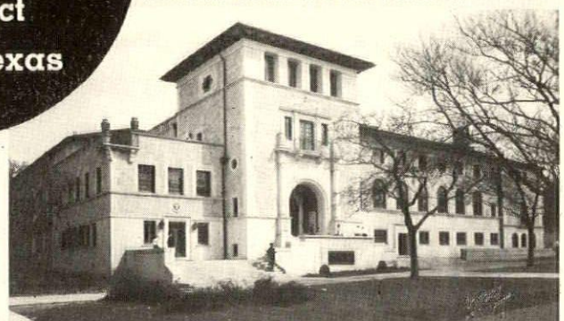
• Student Union Building, University of Texas, at Austin. Genuine wrought iron specified for exposed hot and cold water lines; fire, gas and heating return lines.
