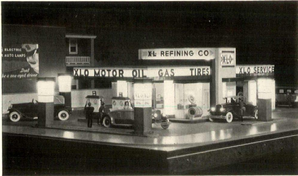
Small-scale model of a gasoline service station, using square pylons with flashed opal glass in metal frames
