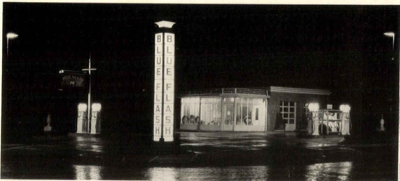
The luminous pylon has been employed effectively in gasoline service-station lighting. This one is lighted by a single vertical row of 100-watt lamps spaced 19½ inches apart. The panels are removable for maintenance
