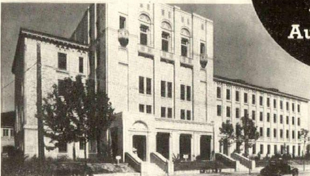
• Hogg Memorial Auditorium, University of Texas, at Austin. Genuine wrought iron specified for exposed hot and cold water lines; fire lines and heating return lines. • Out-Patient Building for the John Sealy Hospital, Galveston. High and low pressure steam lines specified genuine wrought iron.
