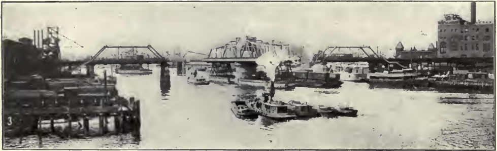
FIG. 11. BRIDGE OVER THE HARLEM RIVER AT SECOND AVE.
