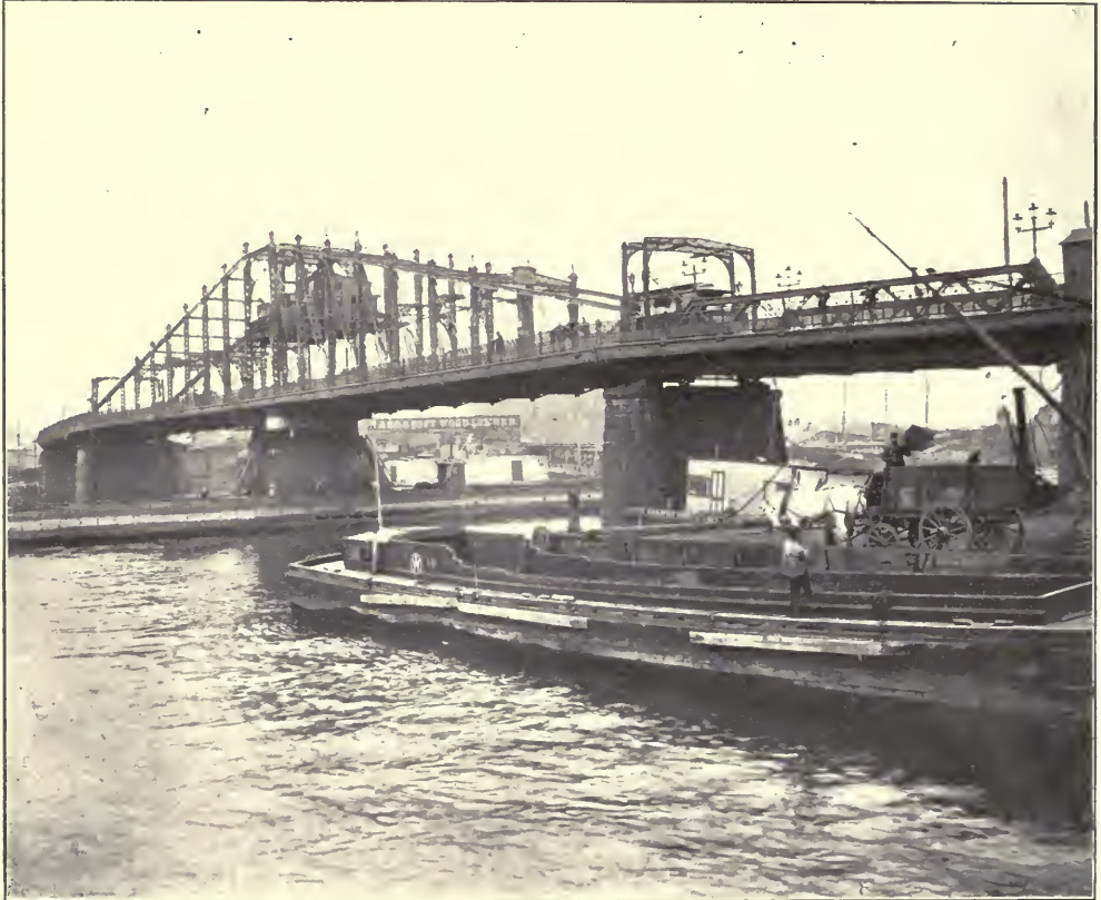
FIG. 3. THE BRIDGE AT MADISON AVE.
