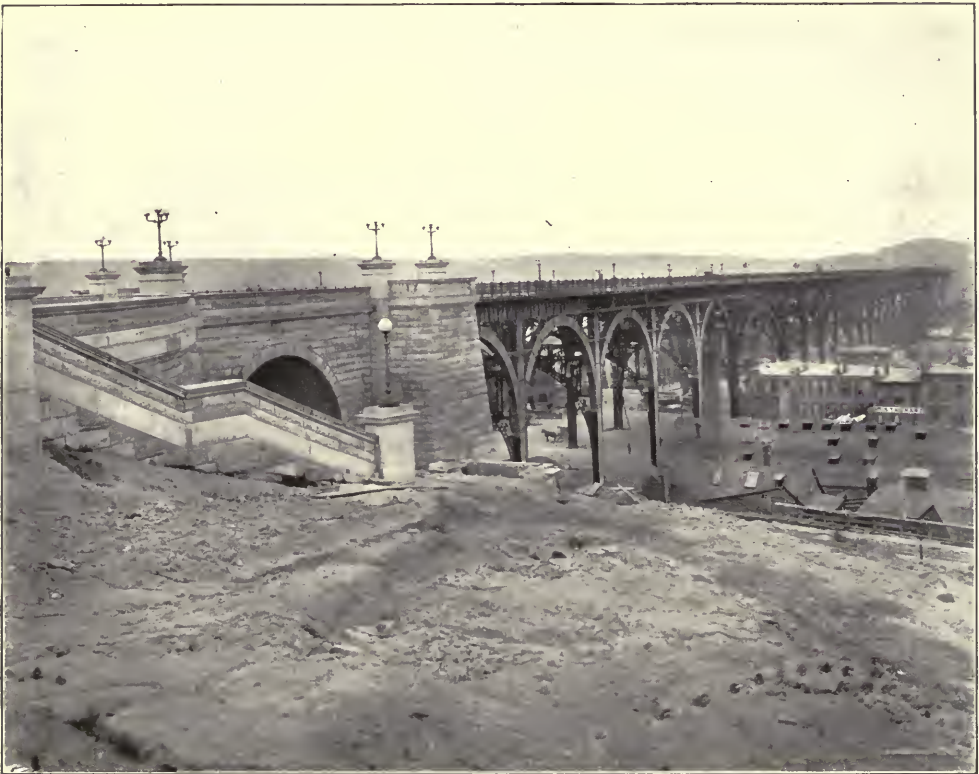
FIG. 8. THE MANHATTAN VALLEY VIADUCT.
