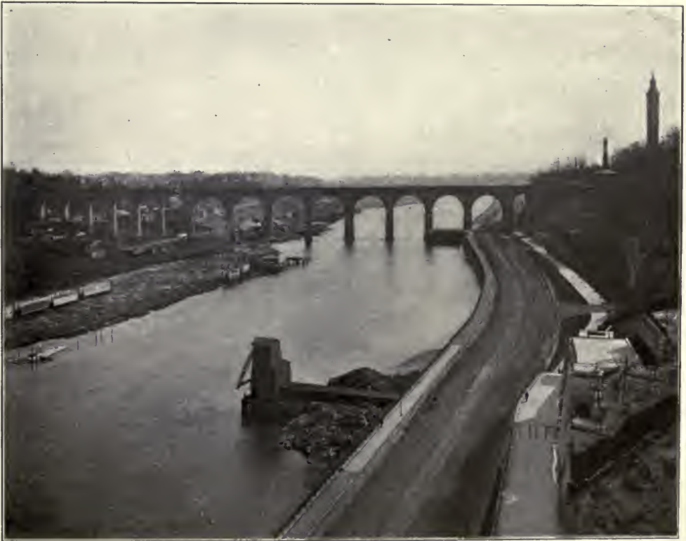
FIG. 7. "HIGH" BRIDGE OVER THE HARLEM RIVER.
