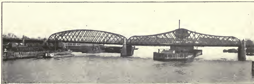
FIG. 5. THE WILLIS AVE. BRIDGE.
