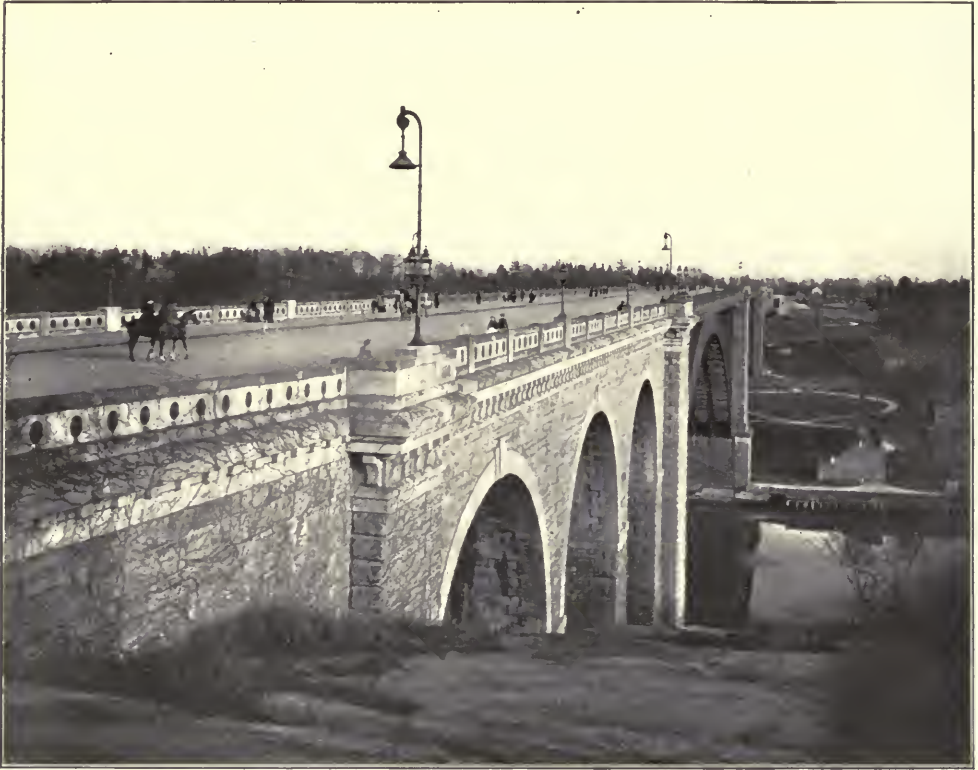
FIG. 17. WASHINGTON BRIDGE FROM THE MANHATTAN SIDE.
