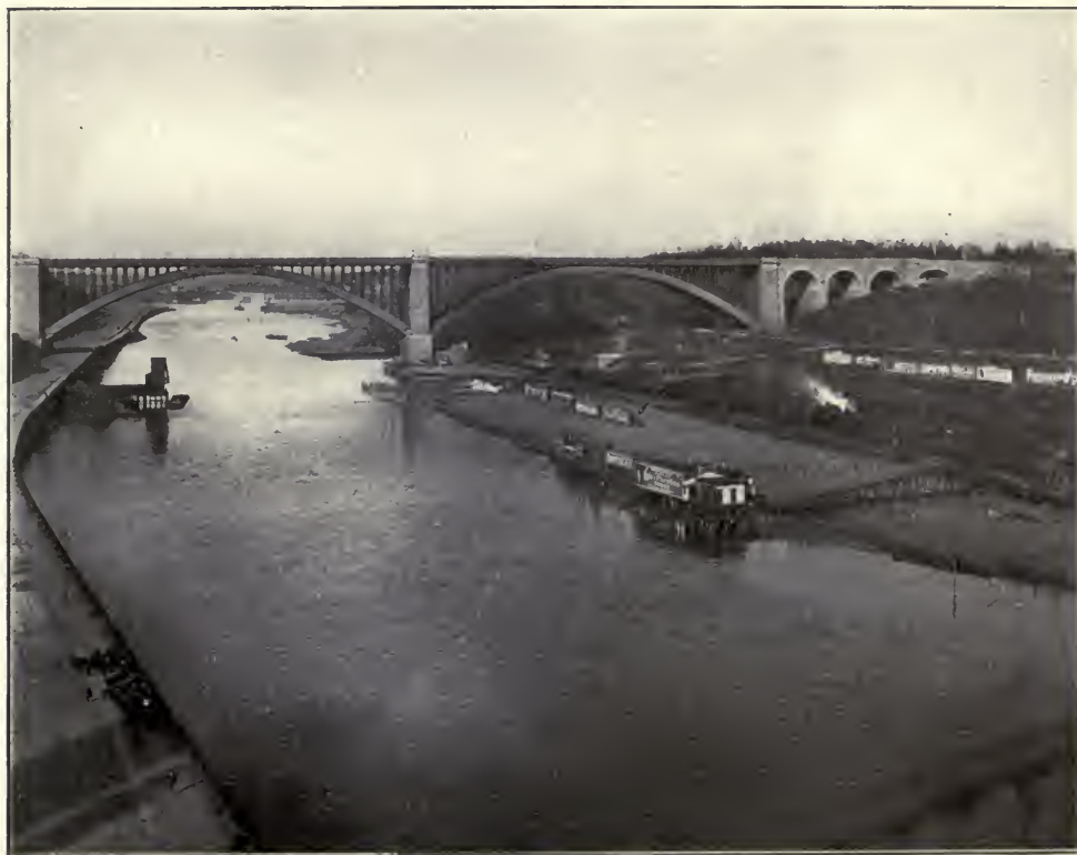
FIG. 16. WASHINGTON BRIDGE FROM THE SOUTH.
