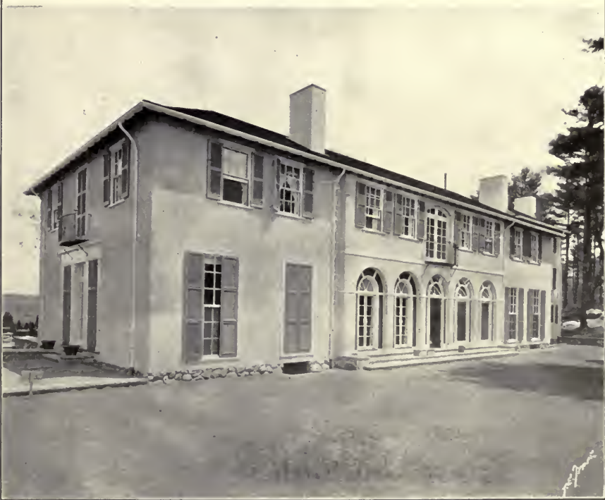
THE SOUTH FRONT OF THE HOUSE OF MR. SAMUEL CABOT.
