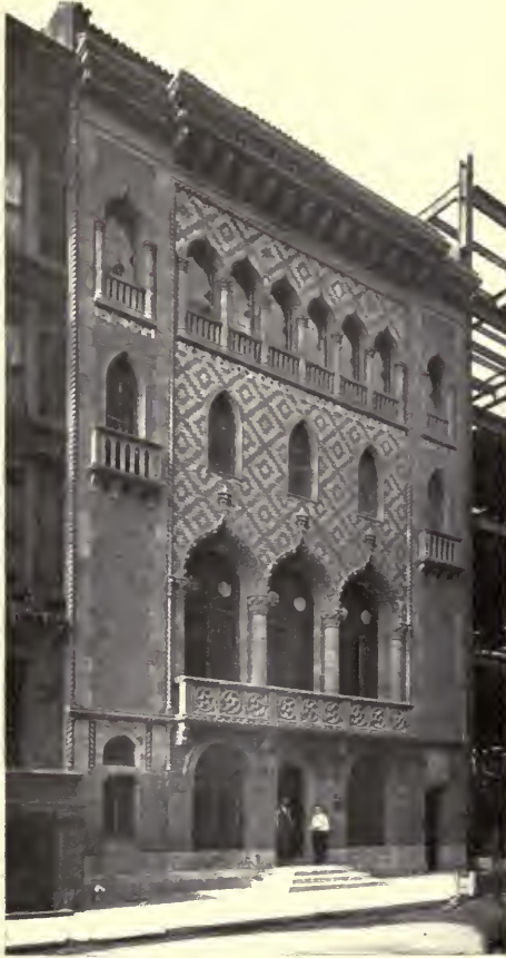
WETZEL BUILDING, EAST 44TH STREET, NEW YORK.
