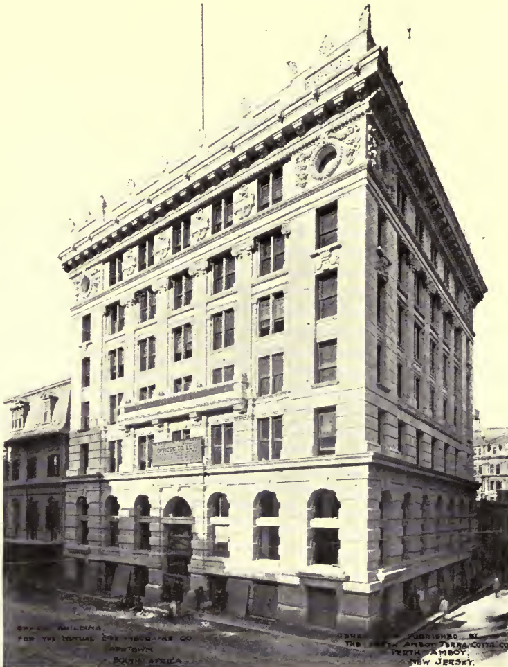
OFFICE BUILDING FOR THE MUTUAL LIFE INSURANCE CO., CAPE TOWN, SOUTH AFRICA.
