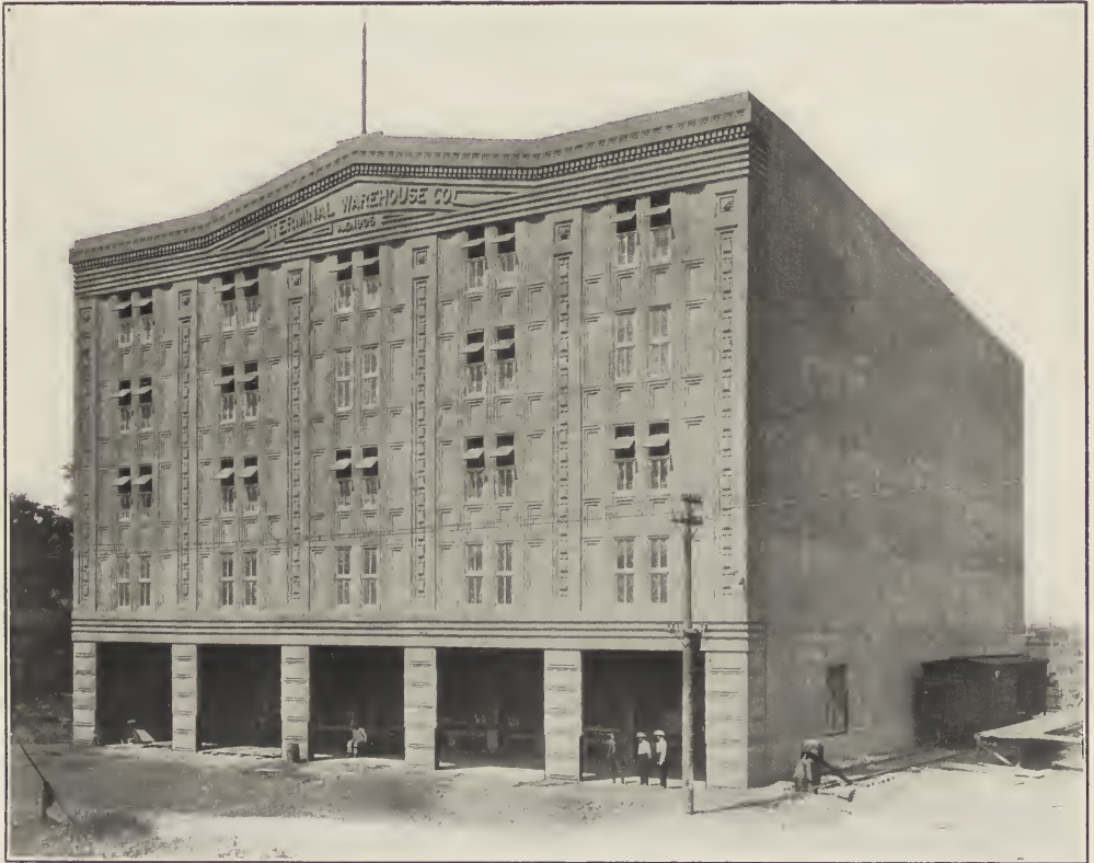
FRONT VIEW—TERMINAL WAREHOUSE.
