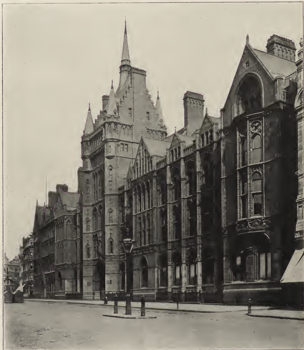
ELEVATION TOWARD HOLBORN—PRUDENTIAL ASSURANCE COMPANY'S BUILDING. Holborn Bars, London. A. Waterhouse & Son, Architects.
