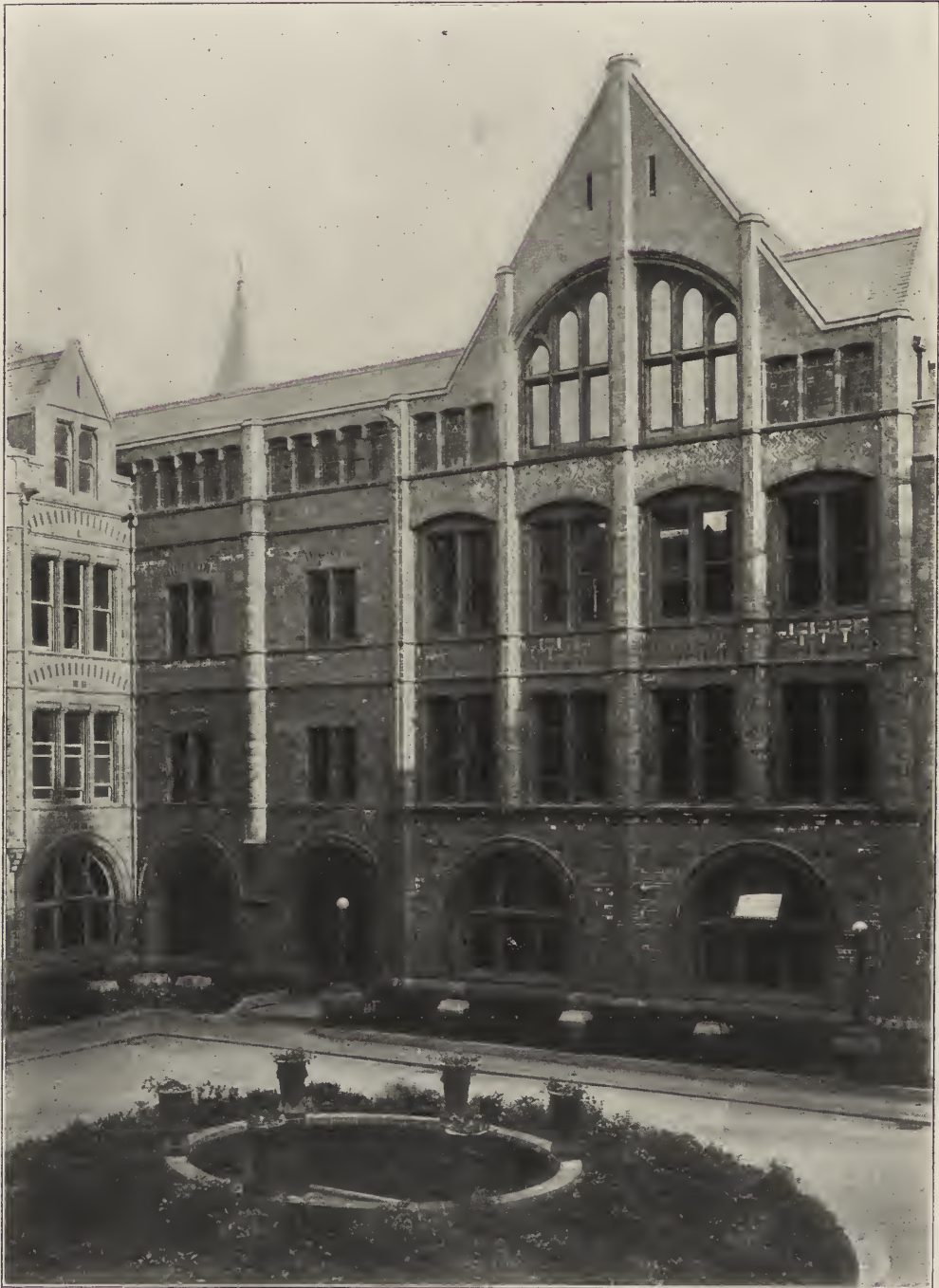
VIEW IN THE INNER COURT—PRUDENTIAL ASSURANCE COMPANY'S BUILDING. Holborn Bars, London. A. Waterhouse & Son, Architects.
