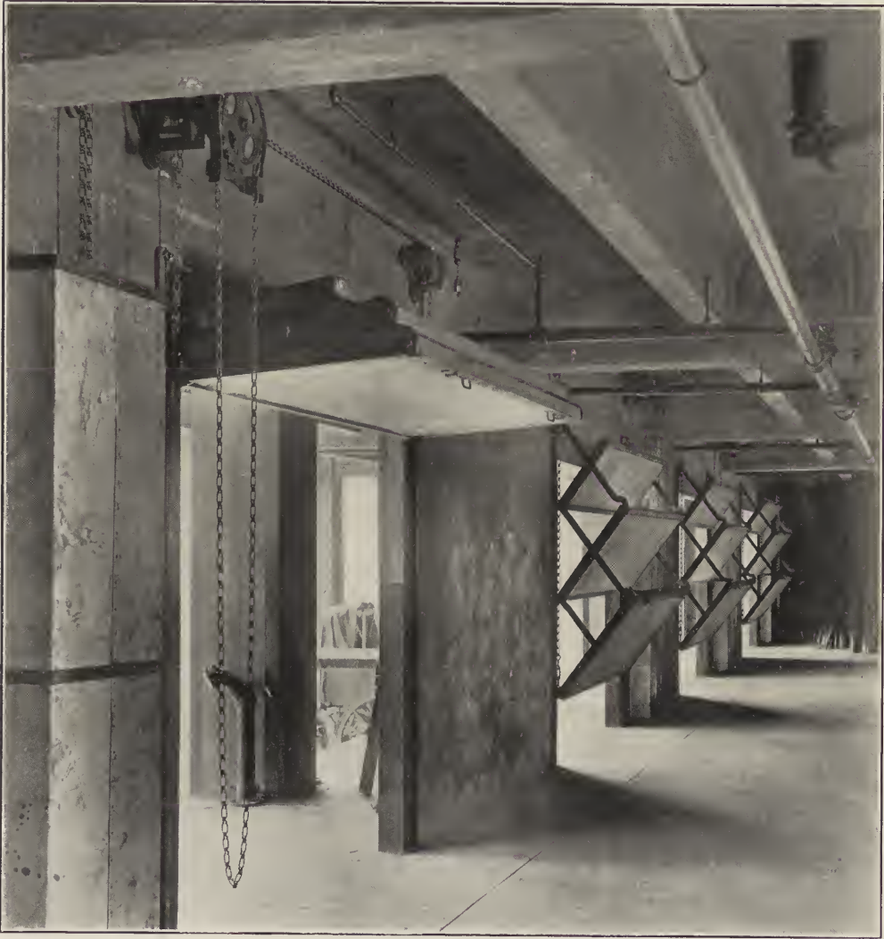
COLLAPSIBLE FIREPROOF DOORS, MADE OF CEMENT ON A STEEL FRAME—TERMINAL WAREHOUSE.
