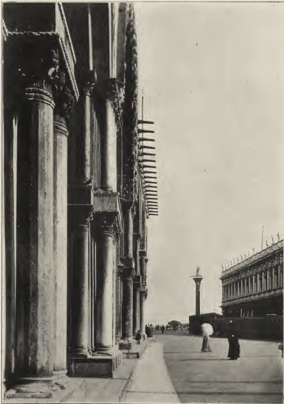
FIG. 11. CURVE IN PLAN, CONCAVE TO EXTERIOR, FAÇADE OF ST. MARK'S AT VENICE. The deflection, of ten inches, is best seen on the outer line of the paving slabs in front of the church. Photograph of the Brooklyn Museum Survey of 1905.
