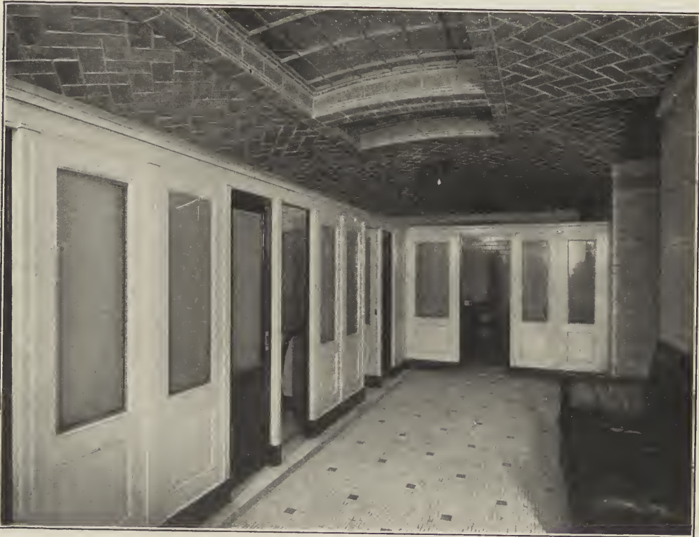
VIEW IN THE BASEMENT.
