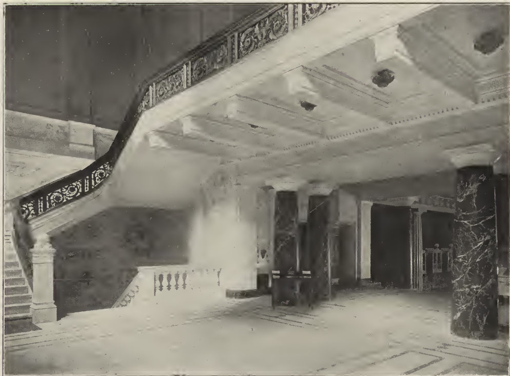
Chicago. NORTHERN TRUST COMPANY—STAIRCASE TO MAIN FLOOR. Frost & Granger, Architects.
