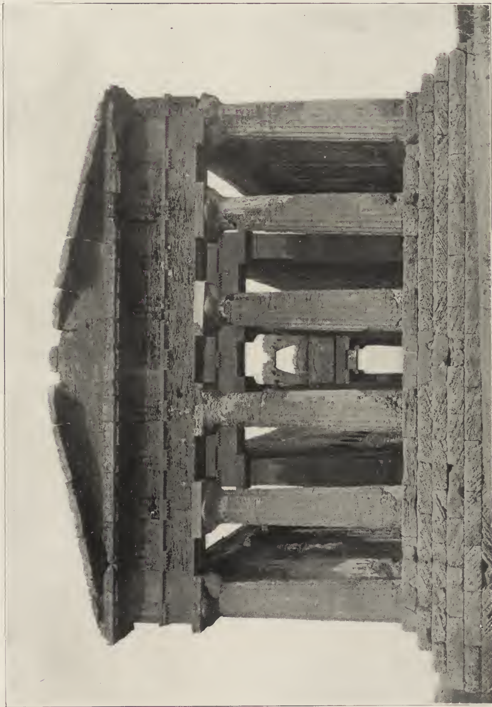
FIG. 8. WEST FRONT OF THE TEMPLE OF CONCORD (SO-CALLED) AT GIRGENTI. In parallel perspective. Illustrating the absence of curvature in the entablature, under the gable. Photograph of the Brooklyn Museum Survey of 1895.
