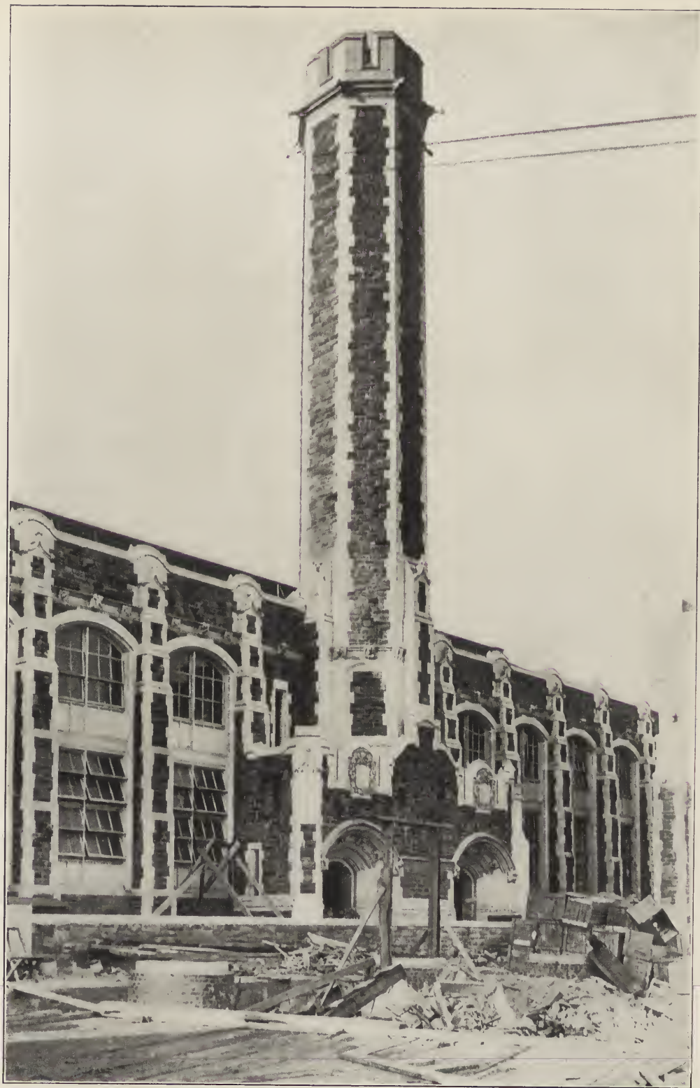
C. C. N. Y. MECHANICAL ARTS BUILDING FROM THE QUADRANGLE. Washington Heights, New York City. (Photo by J. H. Symmons.) George B. Post, Architect.
