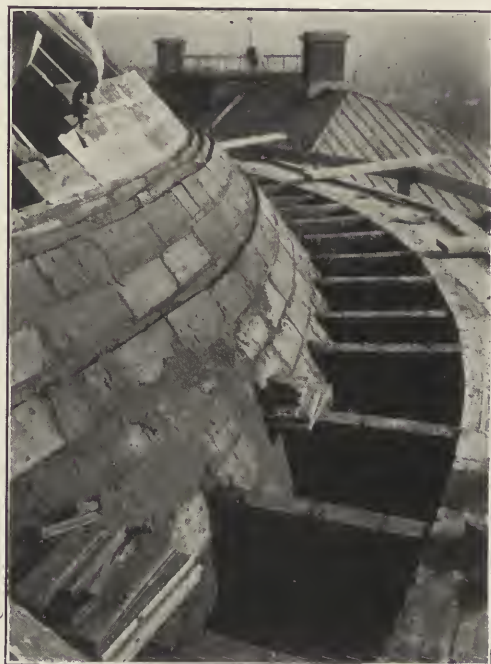
Fig. 10.—The Inner Shell of the Dome Near its Spring.
