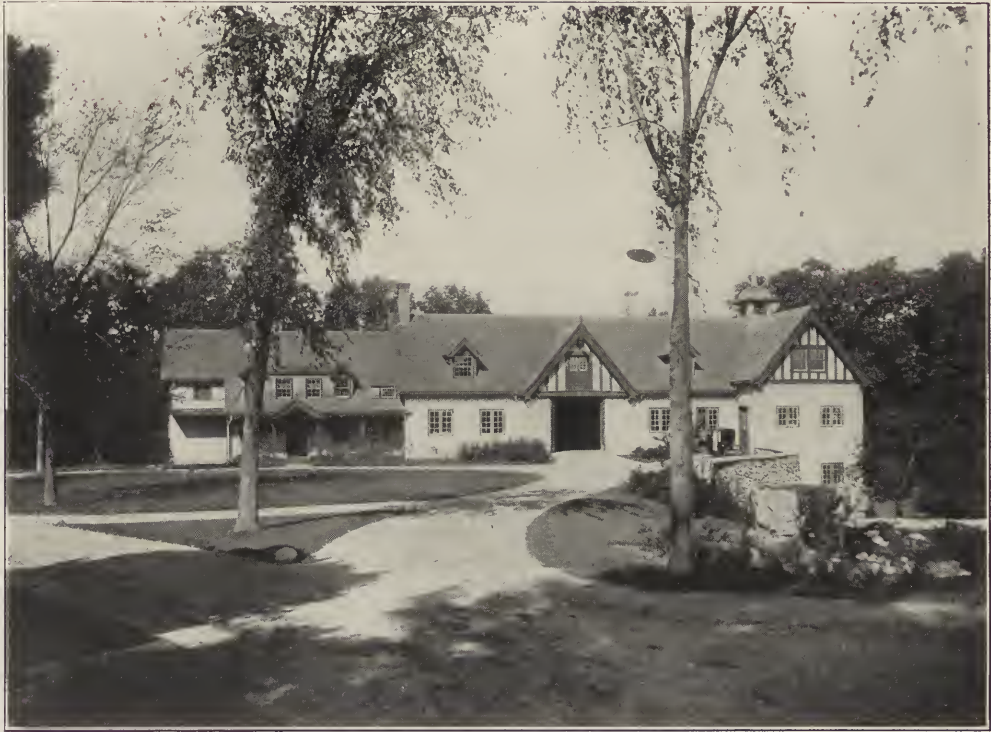
STABLE OF THE SLATER HOUSE.
