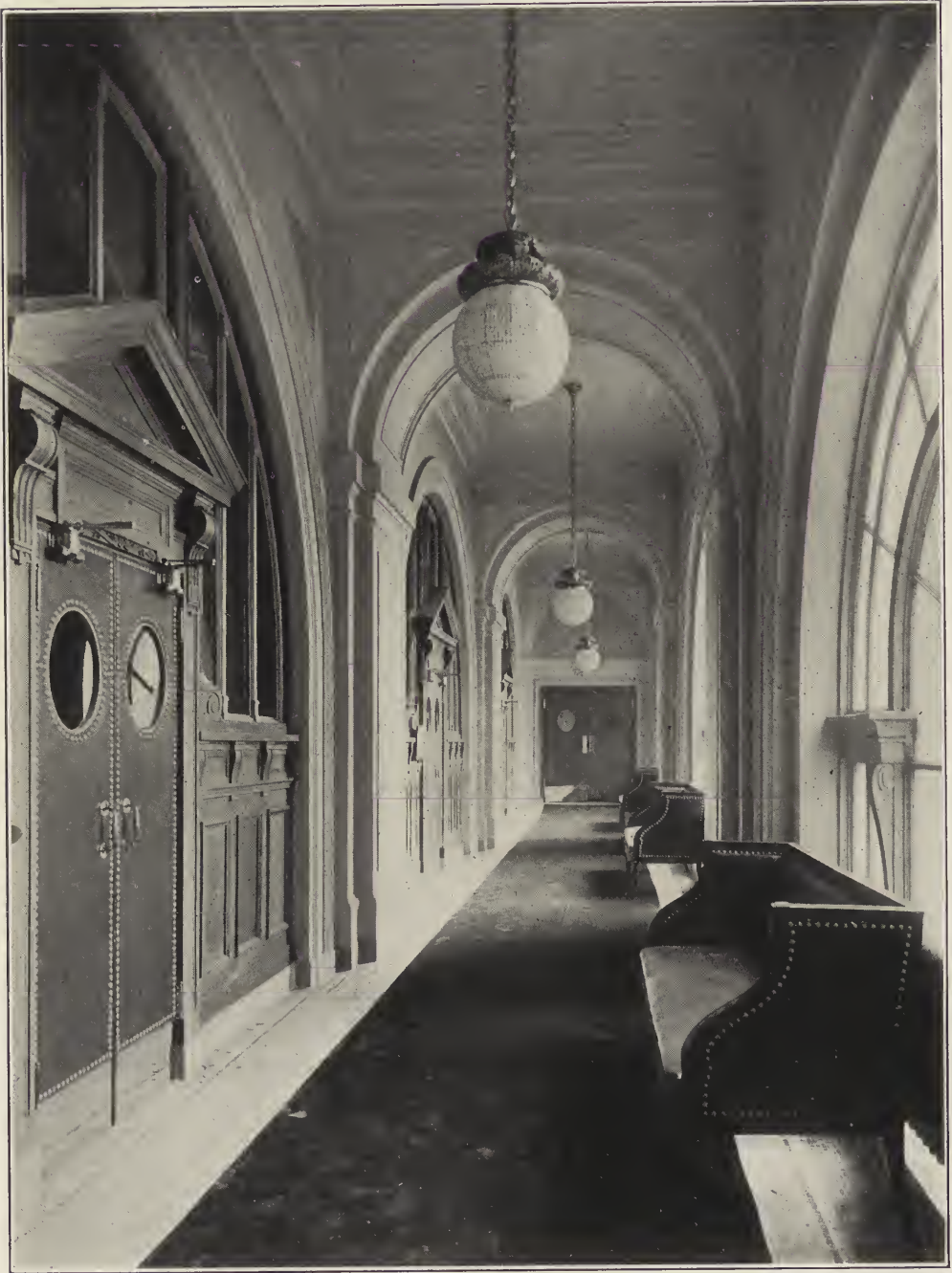
ENGINEERING SOCIETIES' BUILDING—CORRIDOR.
