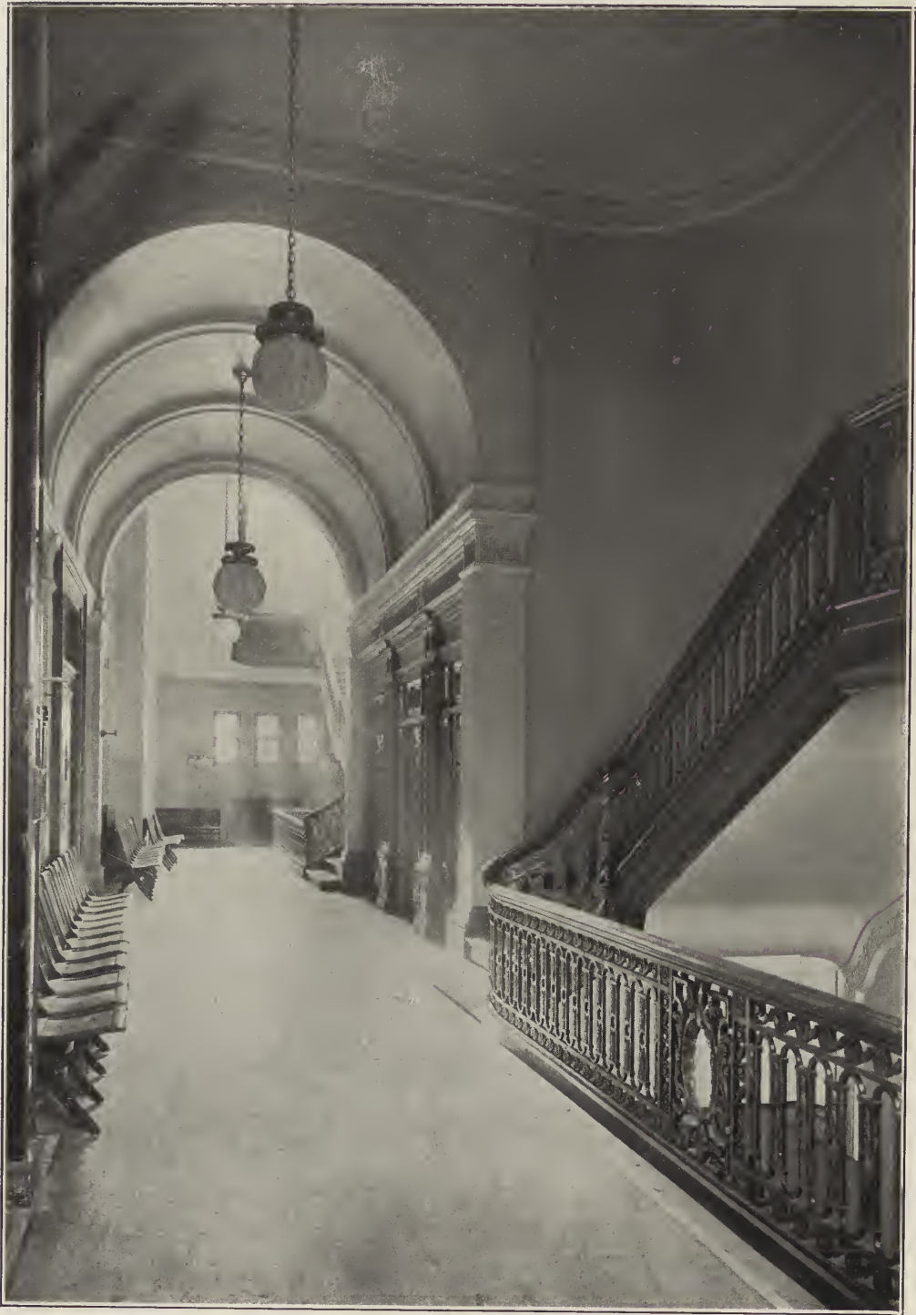
ENGINEERING SOCIETIES' BUILDING—STAIRCASE HALL.
