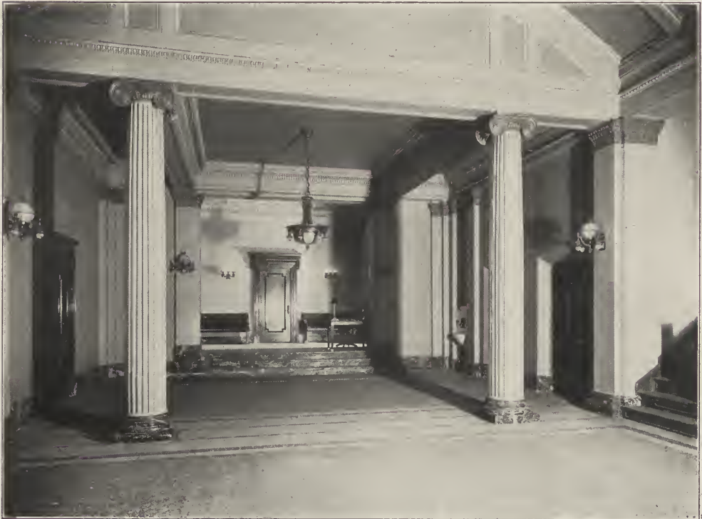
NORTHERN TRUST COMPANY—SECOND FLOOR CORRIDOR. Chicago. Frost & Granger, Architects.
