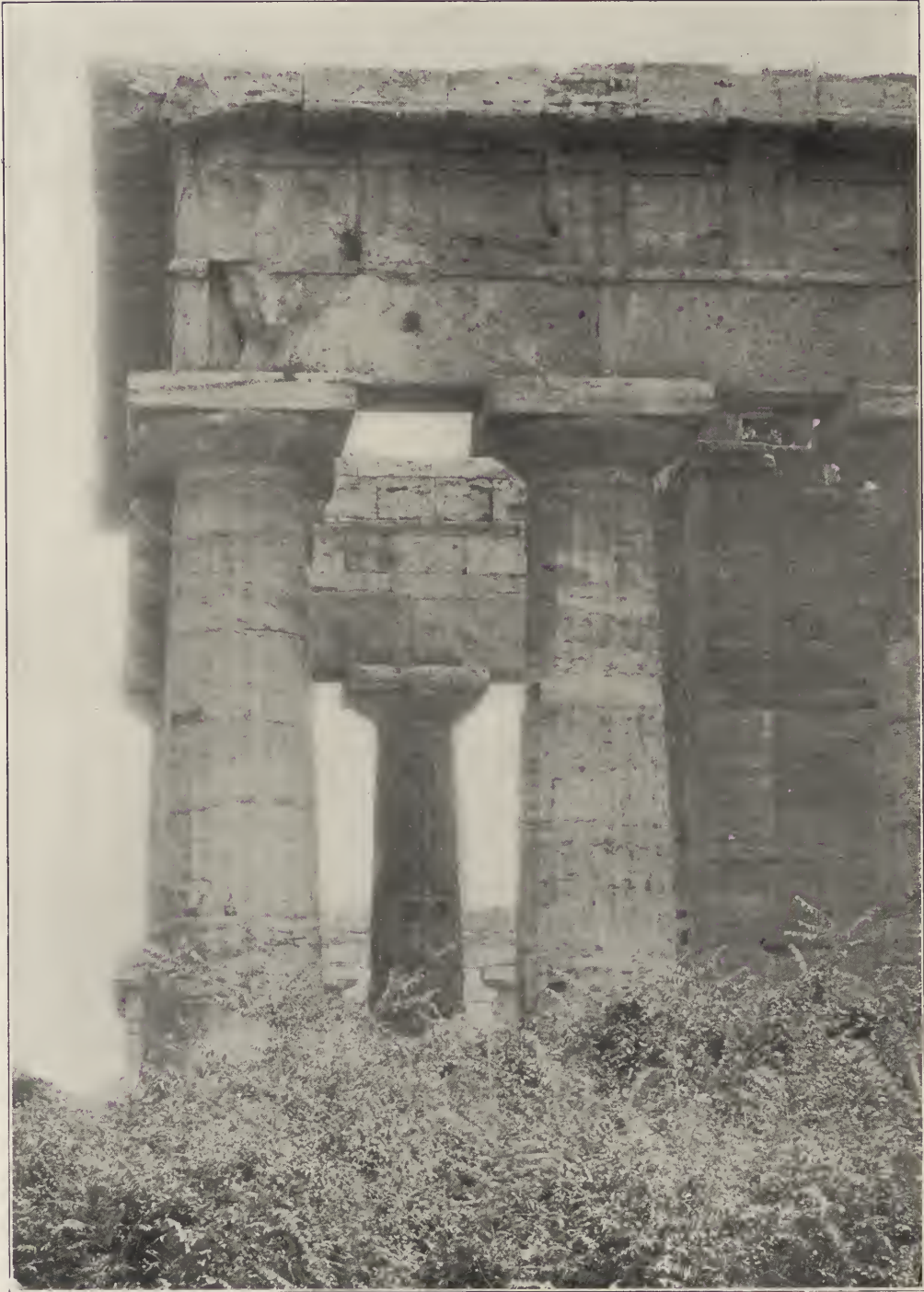
FIG. 10. CURVES IN PLAN, CONCAVE TO EXTERIOR, EAST FRONT OF THE TEMPLE OF NEPTUNE (SO-CALLED) AT PAESTUM. Photograph of the Brooklyn Museum Survey of 1895.
