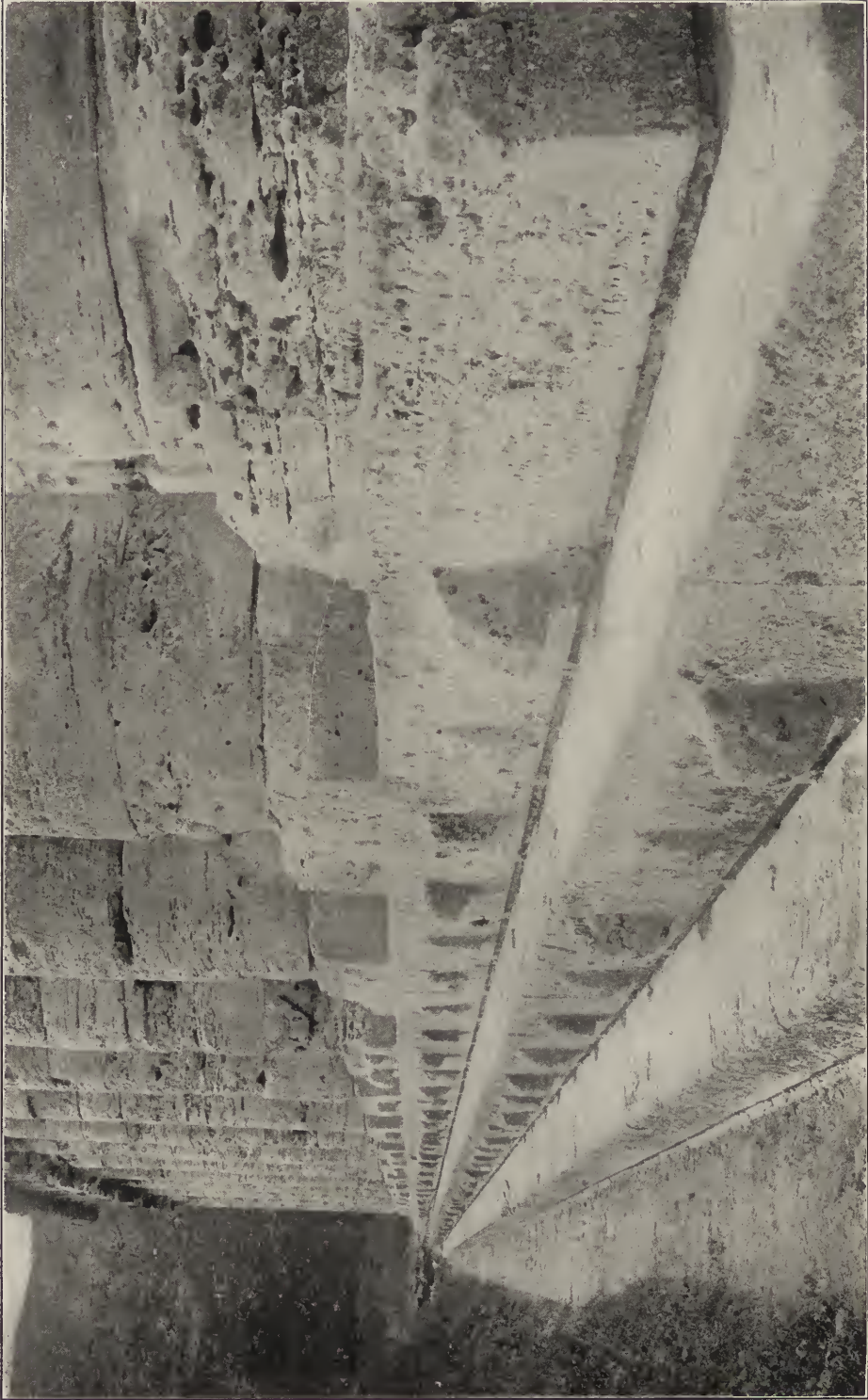
FIG. 4. THE TEMPLE AT EGESTA. Showing the rising curve in elevation of the stylobate. Photograph of the Brooklyn Museum Survey of 1895.
