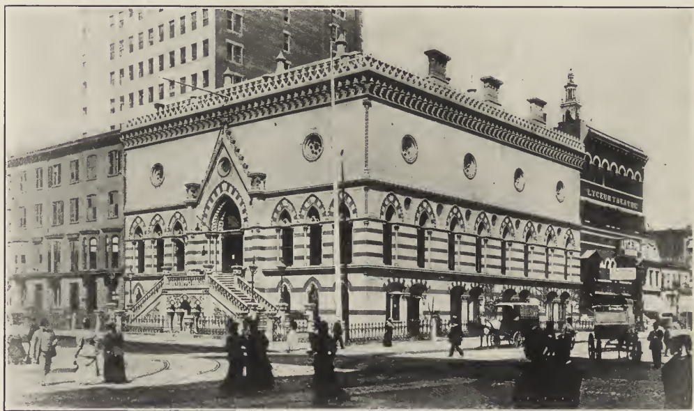
THE ACADEMY OF DESIGN, AT TWENTY-THIRD STREET AND MADISON AVENUE, RECENTLY DEMOLISHED. THE METROPOLITAN LIFE INSURANCE COMPANY'S BUILDING NOW OCCUPIES THE SITE.
