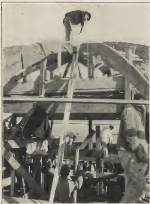
Fig. 9.—The Summit of the Centering for the Dome.
