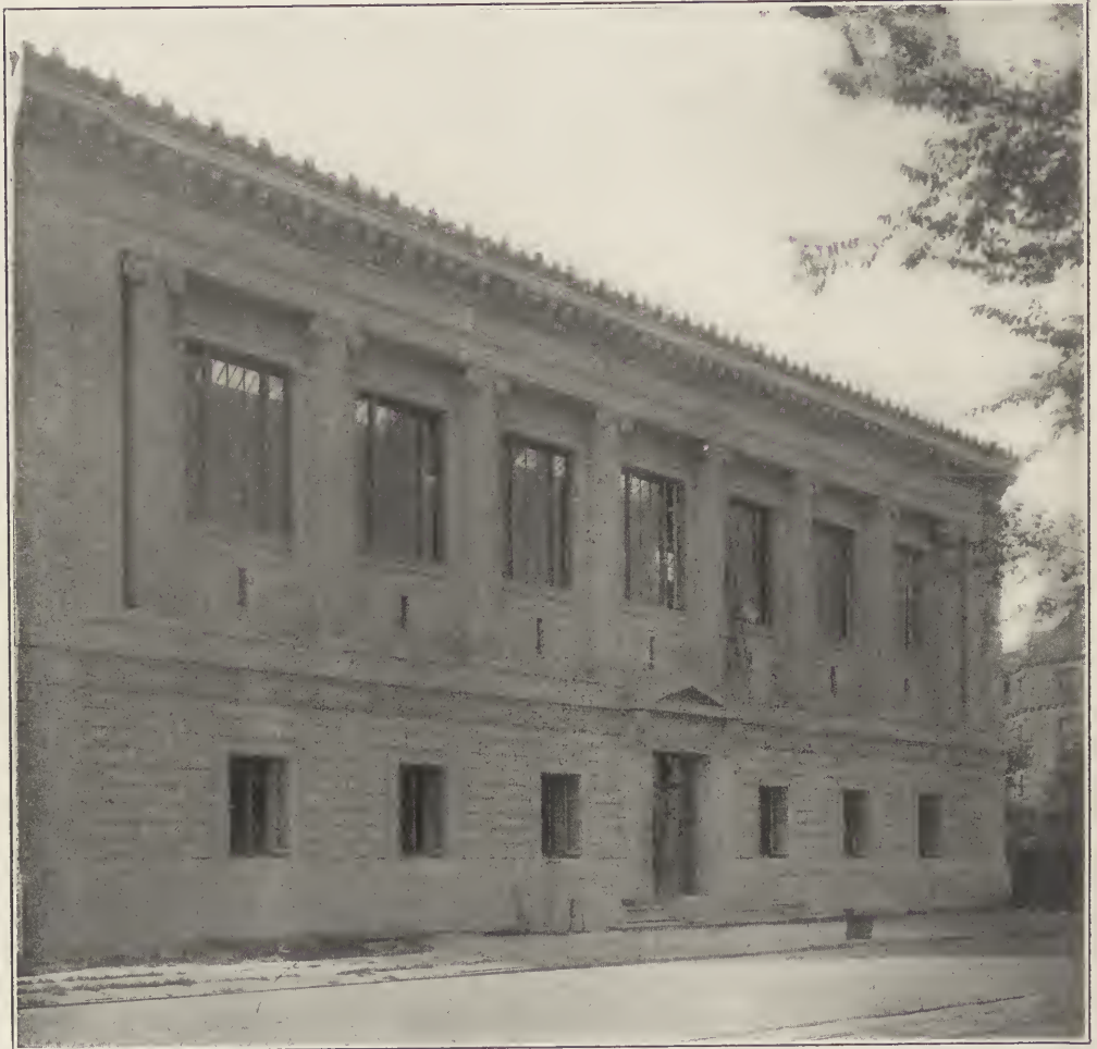
THE NEW BUILDING OF THE NEW YORK HISTORICAL SOCIETY. 77th Street and Central Park West, New York.
