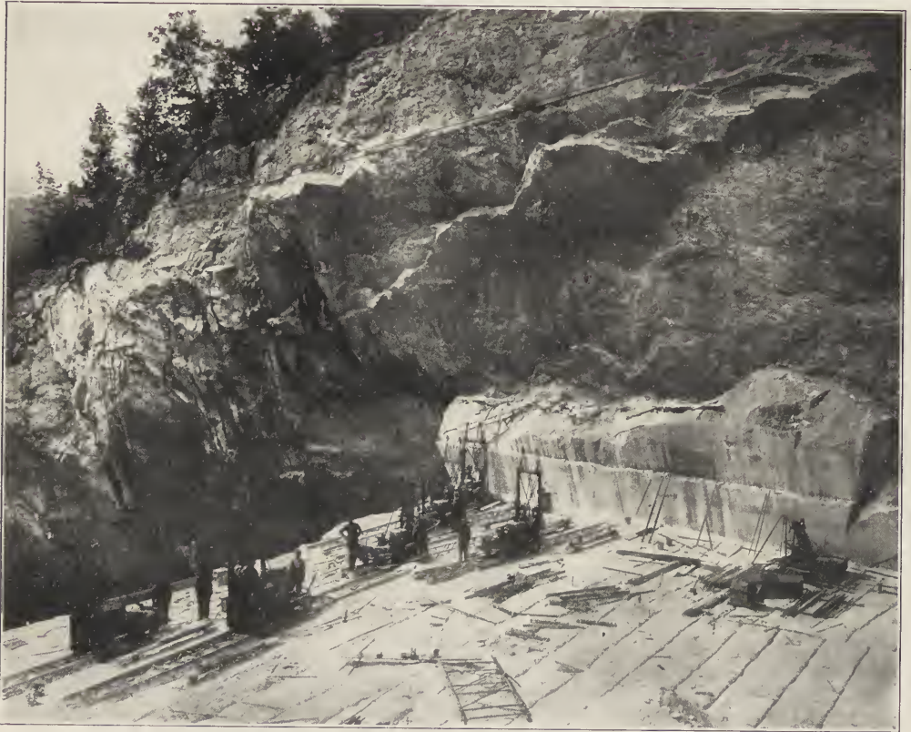
THE CUTTING MACHINES AT WORK IN THE AMERICAN CARRARA.
