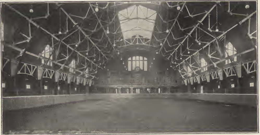
INTERIOR OF RIDING ACADEMY OF MR. ALFRED G. VANDERBILT—OAKLAND FARM. Portsmouth, R. I. Ewing & Chappell, Architects.
