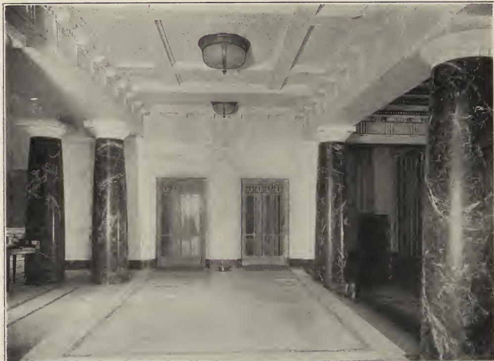
NORTHERN TRUST COMPANY—BASEMENT CORRIDOR.
