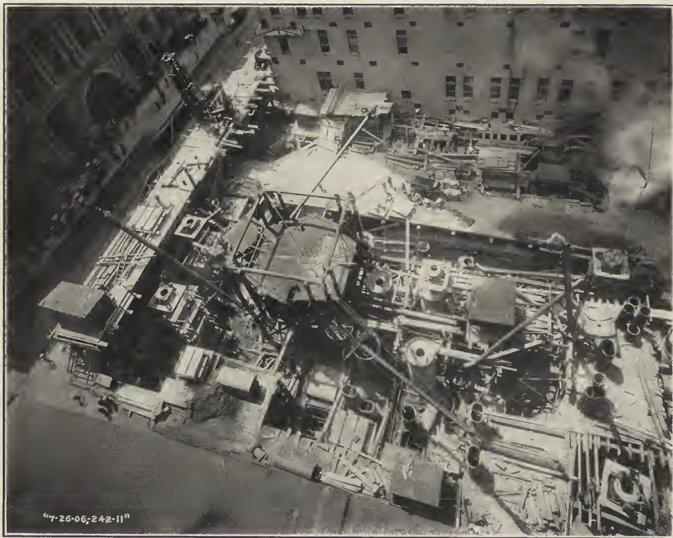
BIRD'S-EYE VIEW, SHOWING CAISSONS IN VARIOUS STAGES OF SINKING AT THE U. S. REALTY BUILDING, NEW YORK.
