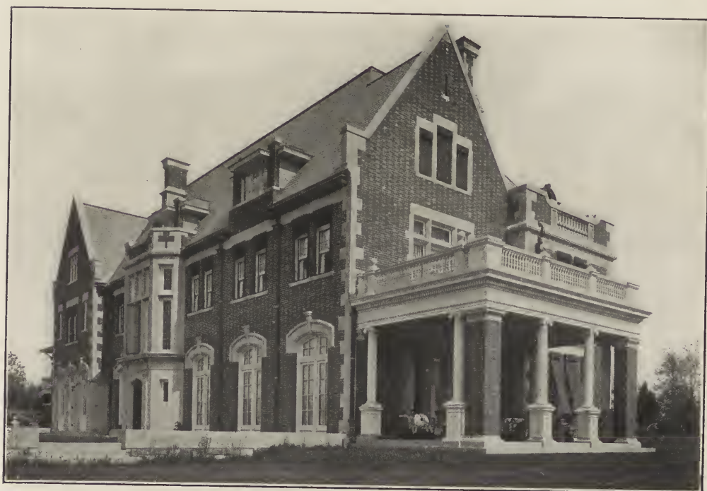
REAR VIEW—RESIDENCE OF MR. G. L. BOISSEVAIN. Mount Kisco, N. Y. George E. Wood, Architect. (Photos by A. Patzig.)
