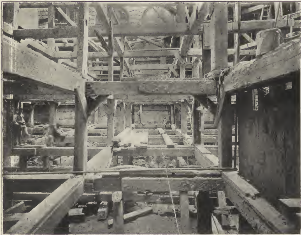
DOWN IN THE FOUNDATION OF THE COMMERCIAL CABLE ANNEX, NEW YORK.
