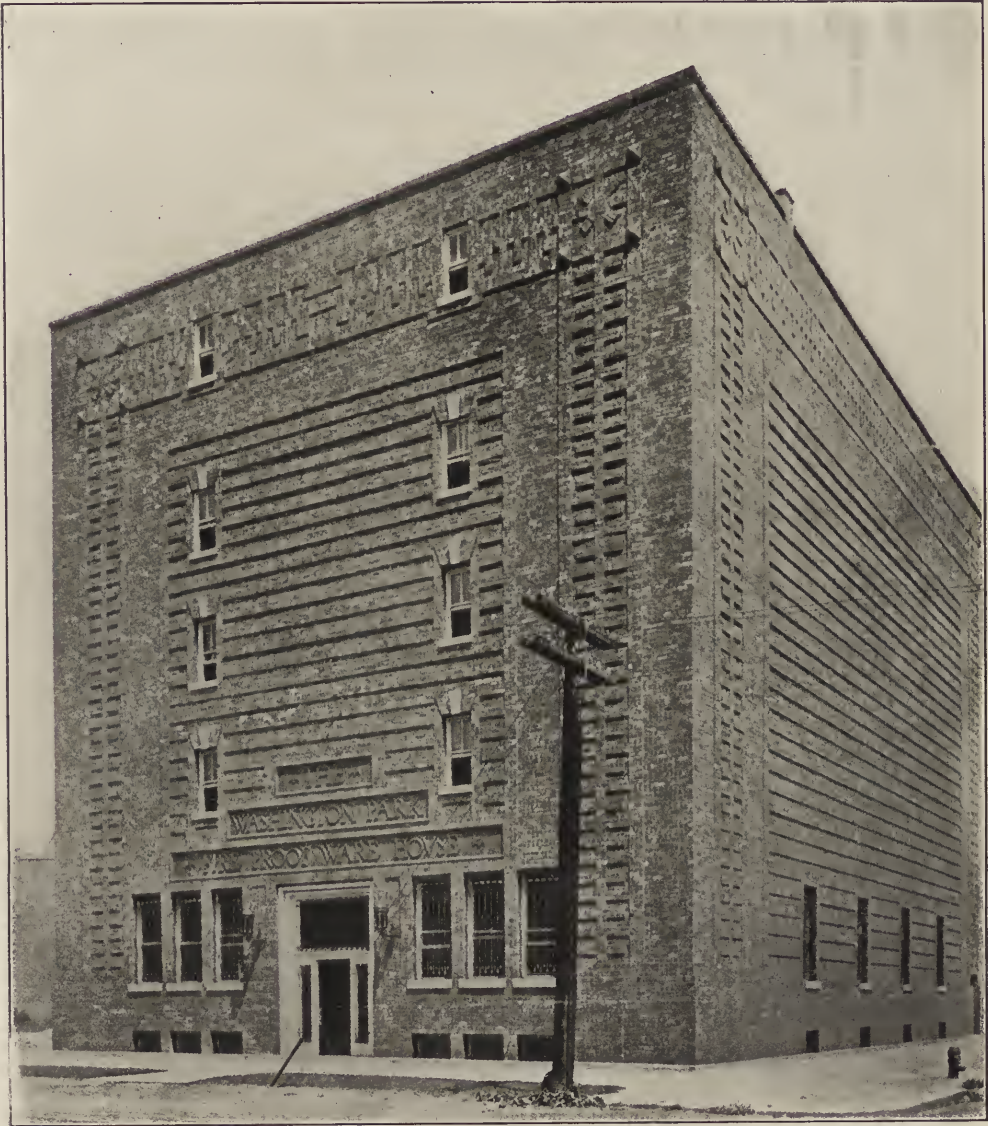
FIG. 2. WASHINGTON PARK WAREHOUSE.
