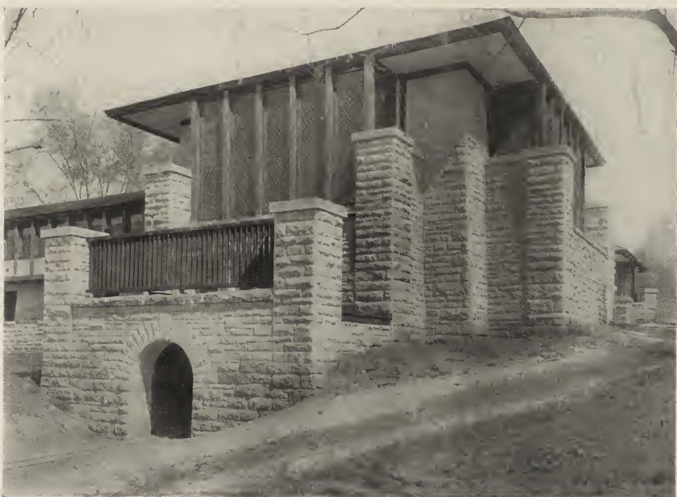
Detail of exterior of assembly room.
