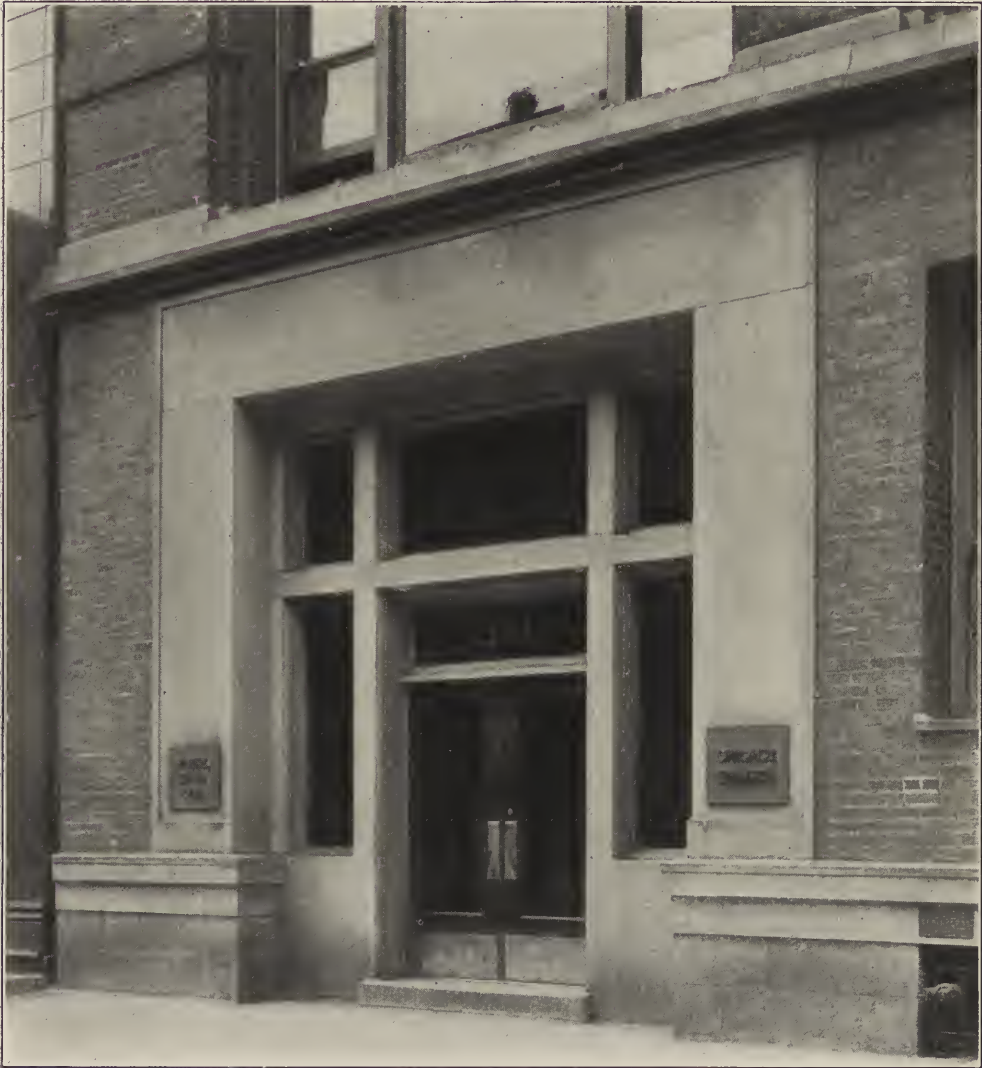
PARKE, DAVIS & CO.'S WAREHOUSE—DETAIL OF FIG. 1.
