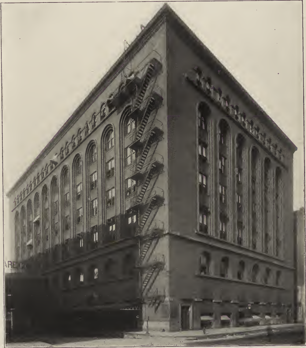
FIG. 10. THE CUPPLES WAREHOUSE.
