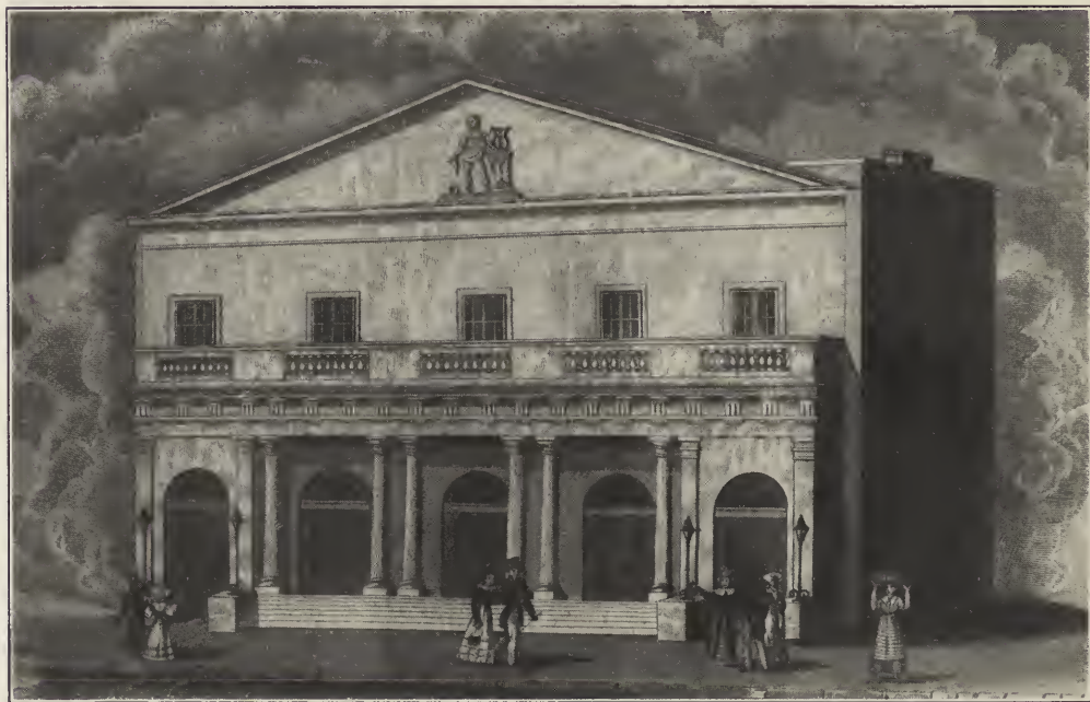
THE ARCH STREET THEATRE BEFORE ALTERATIONS.
