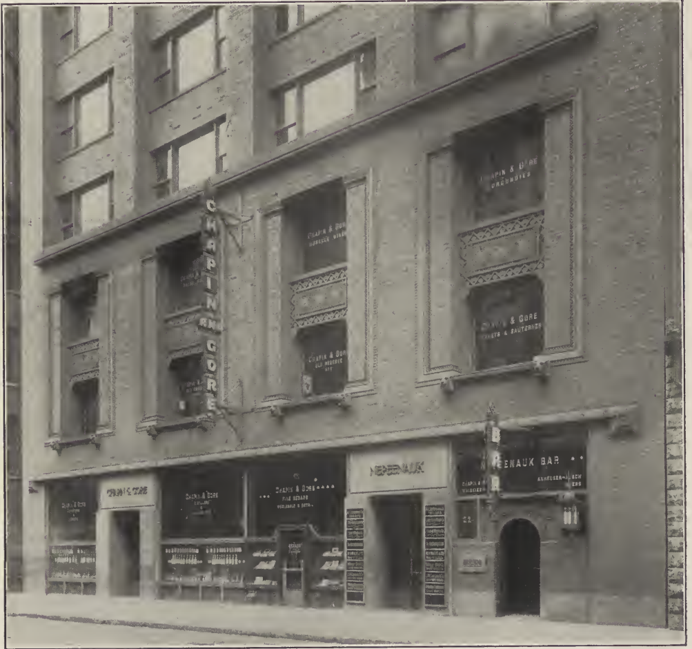
THE CHAPIN & GORE BUILDING. DETAIL OF LOWER STORIES. Chicago, Ill. Richard E. Schmidt, Architect.
