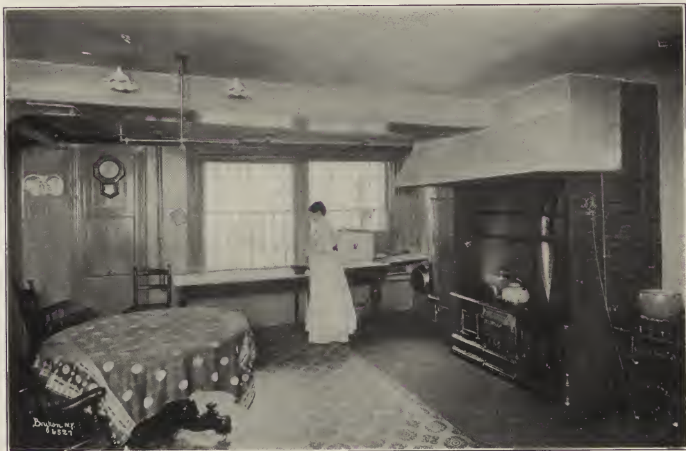
The ventilation of a kitchen must be carefully attended to. A hood over the range connected with a large flue running up next the smoke flue must be provided to carry up hot air.
