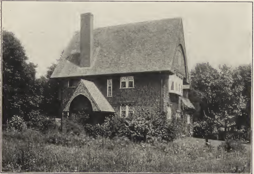
FIG. 7. HOUSE OF HENRY V. KIRBY, ARCHITECT. South Orange, N. J.
