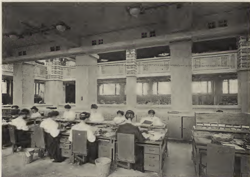
FIG. 4. LARKIN BUILDING—FOURTH STORY GALLERY.
