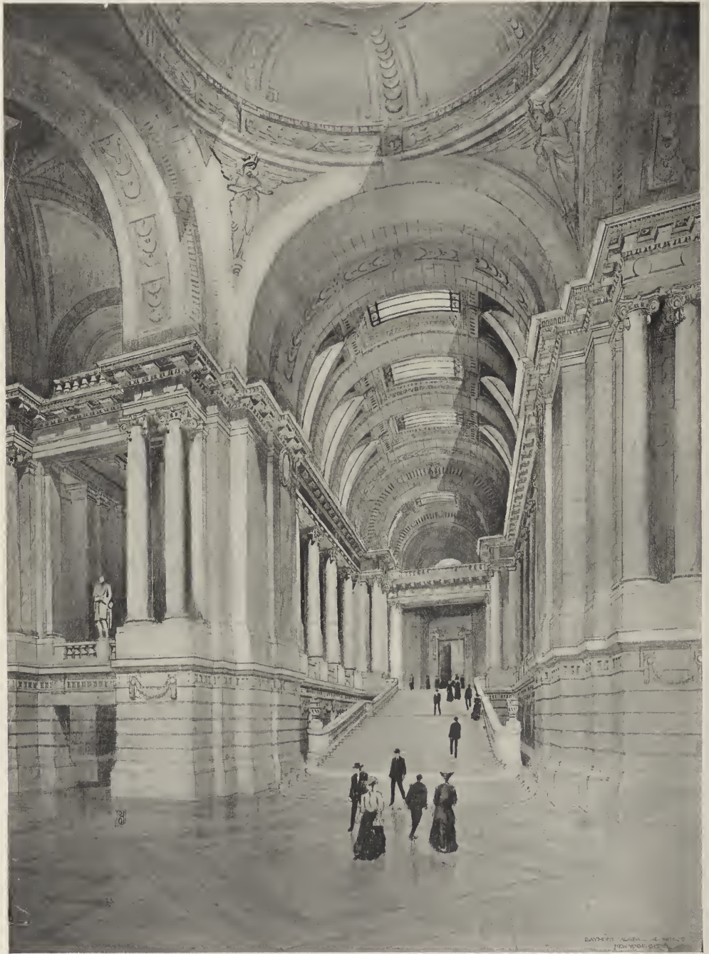
VIEW OF THE GREAT ENTRANCE VESTIBULE ON THE FIRST FLOOR, LOOKING TOWARDS THE GRAND STAIRCASE. BROOKLYN CENTRAL LIBRARY. Brooklyn, New York City. Raymond F. Almirall, Architect.
