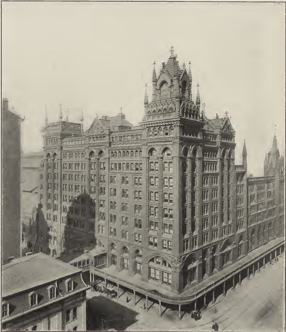
PENNSYLVANIA R. R.—BROAD STREET STATION, CITY HALL SQUARE.
