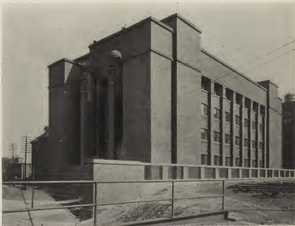
FIG. 6. LARKIN OFFICE BUILDING—REAR.
