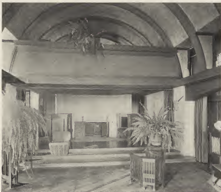
DANA HOUSE—FIREPLACE ALCOVE AT END OF GALLERY. BALCONY ABOVE.
