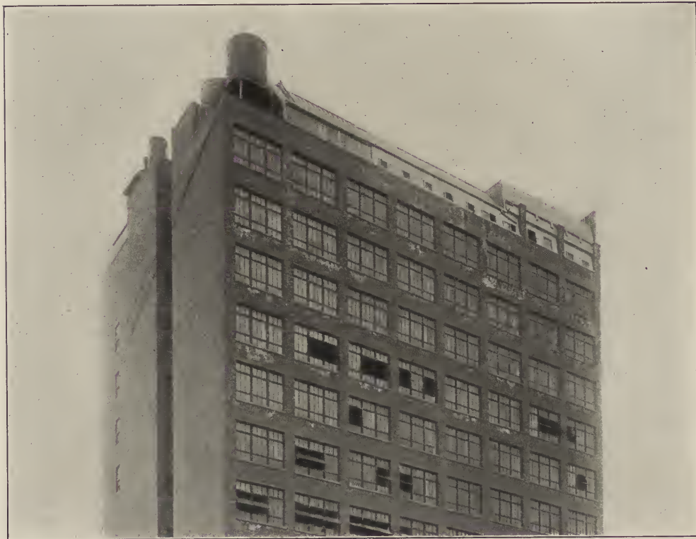
FIG. 4. REAR UPPER PORTION OF THE NEW SCRIBNER PUBLISHING HOUSE.
