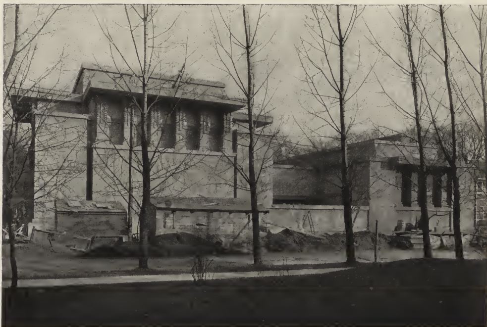
BUILDING FOR UNITY CHURCH IN PROCESS OF CONSTRUCTION. Oak Park, Ill.
