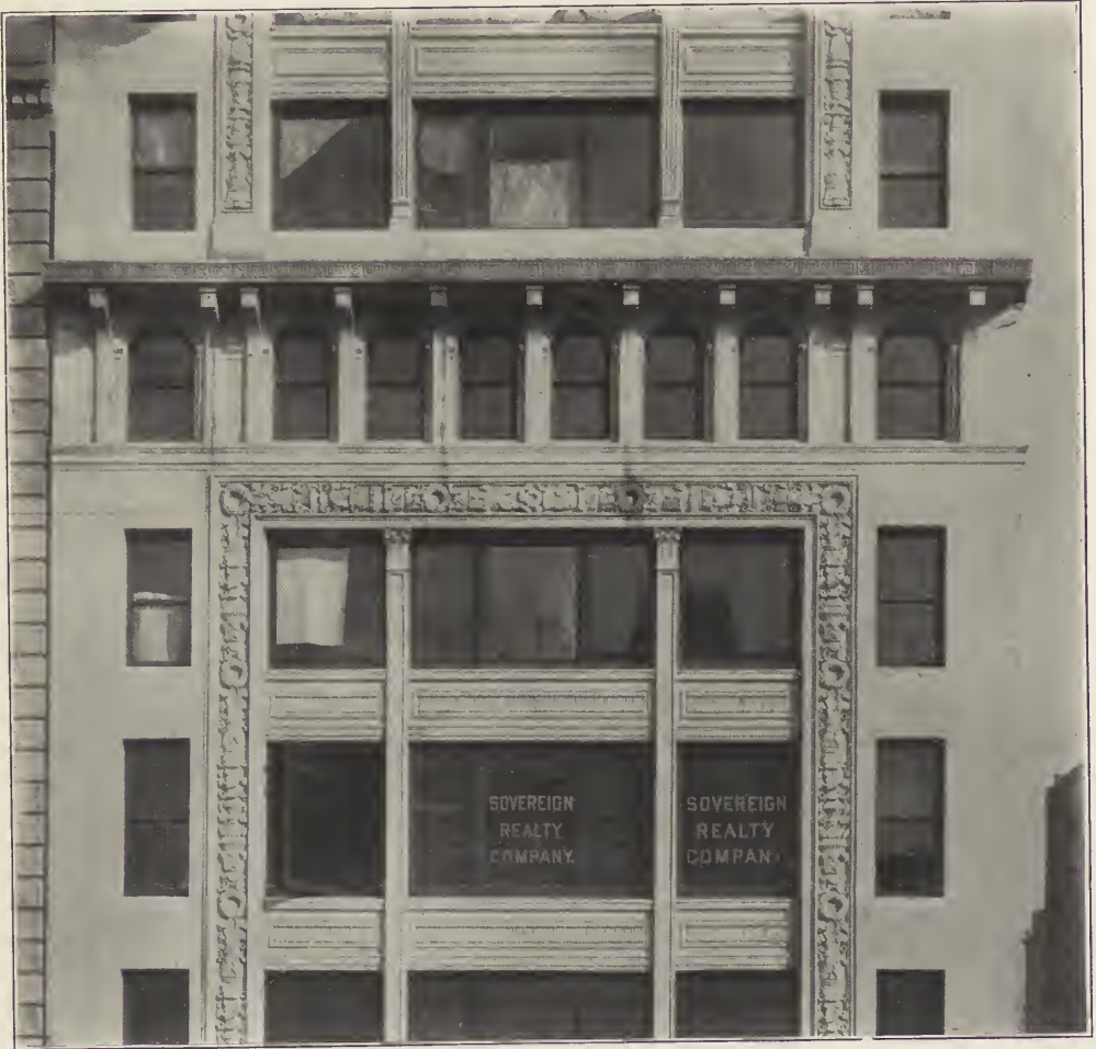
DETAIL OF THE MONOLITH BUILDING.
