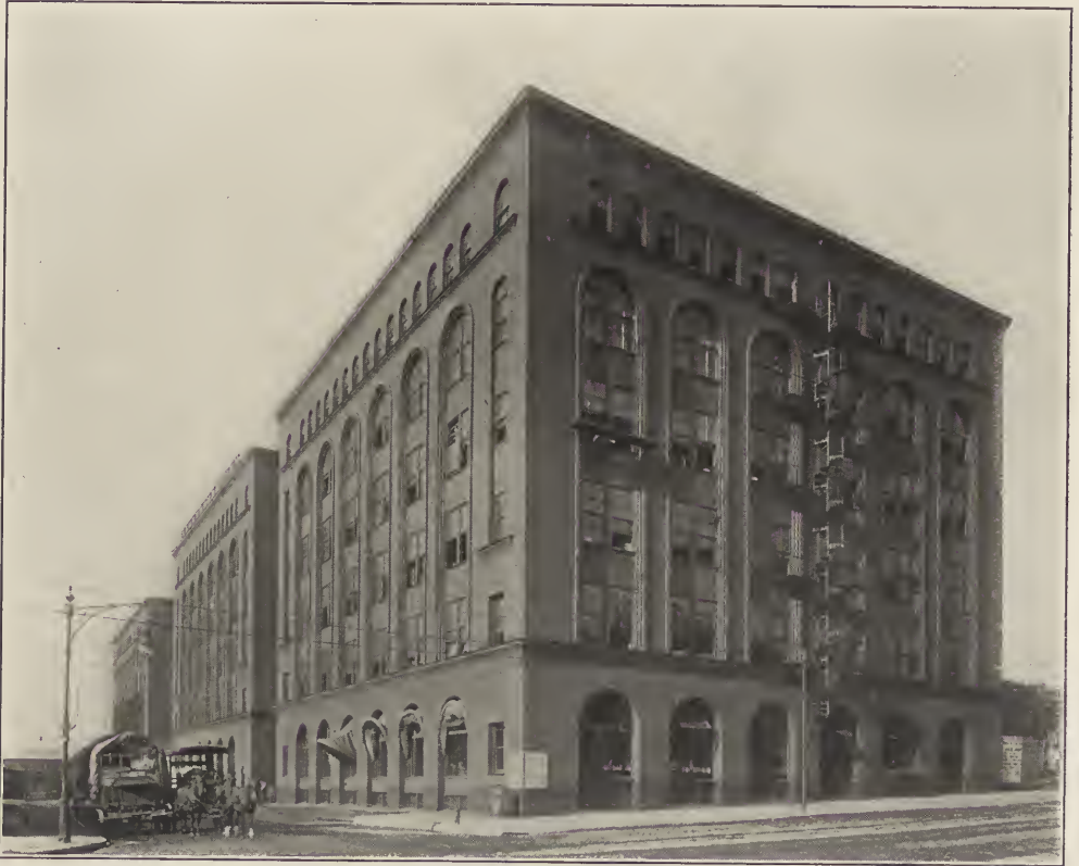
FIG. 9. THE CUPPLES WAREHOUSE.
