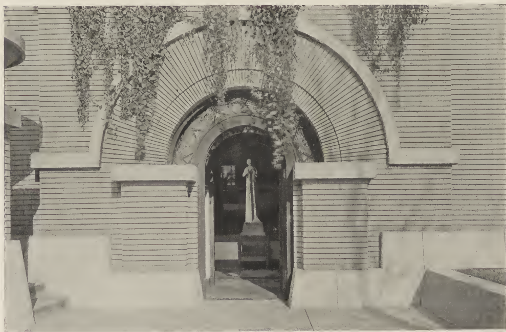
DANA HOUSE—DETAIL OF MAIN ENTRANCE, SHOWING VISTA INTO LIVING HALL.
