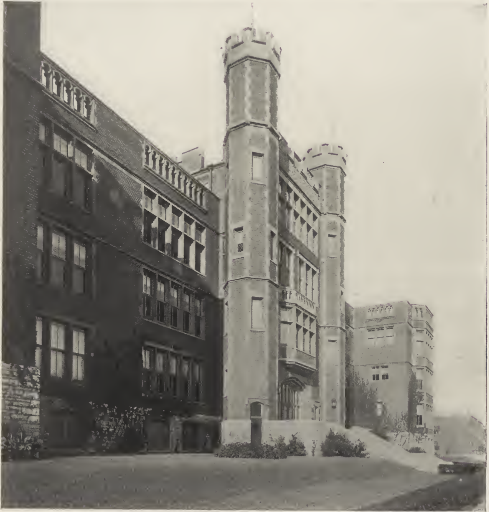
McKINLEY HIGH SCHOOL—DETAIL OF ENTRANCE TOWER. ST. LOUIS, MO. St. Louis, Mo. W. B. Ittner, Architect.
