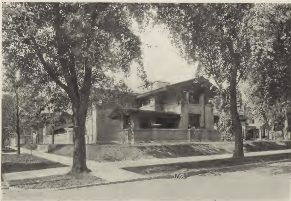
DANA HOUSE—GENERAL VIEW FROM CORNER.
