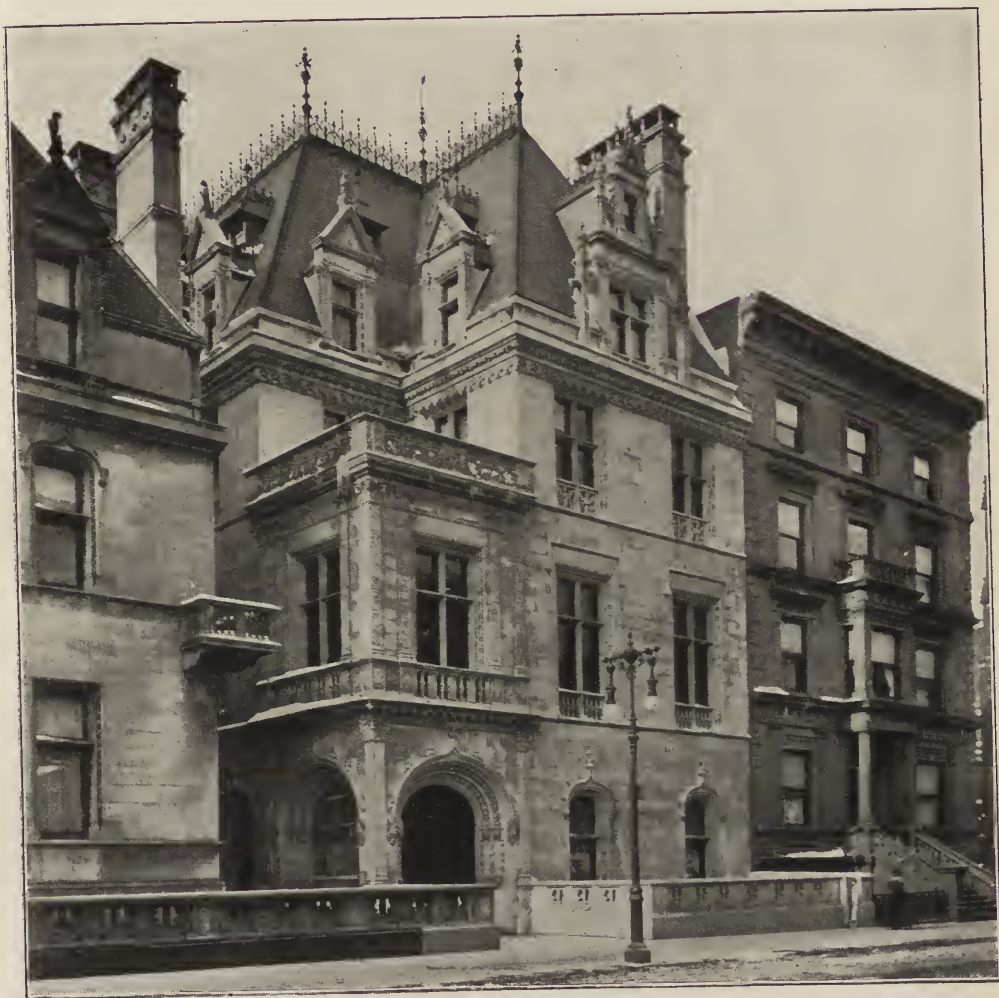
THE W. K. VANDERBILT, JR., RESIDENCE, SHOWING THE OLDER HOUSE ON THE LEFT. 52d Street and 5th Avenue, New York. McKim, Mead & White, Architects. (Photo by J. H. Symmons.)
