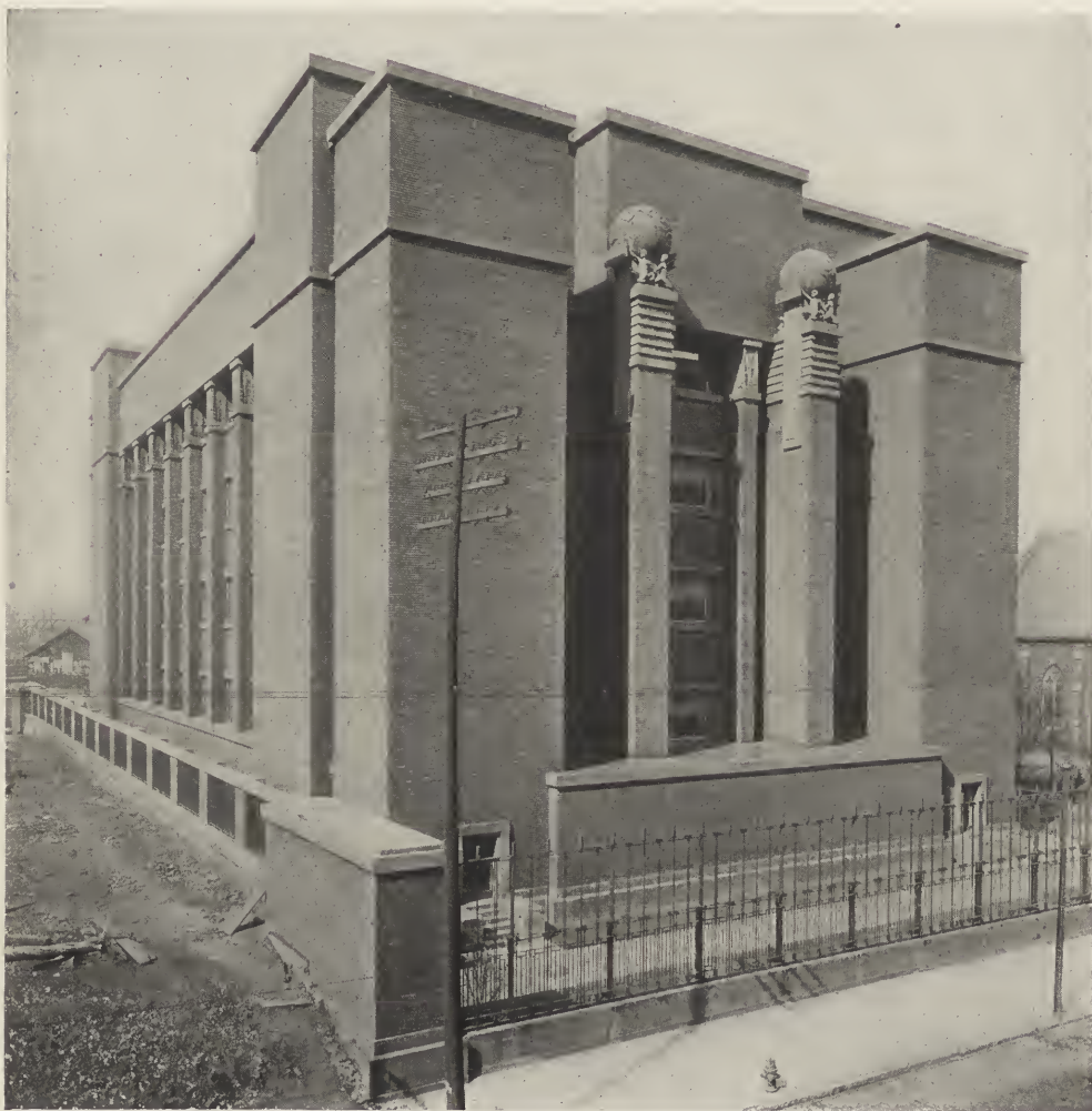
FIG. 1. LARKIN OFFICE BUILDING—REAR.
