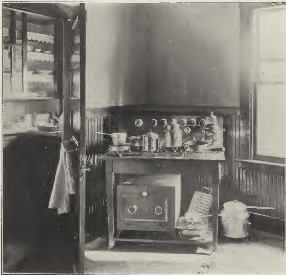
Where electricity is cheap, it is used in the ideal kitchen. Ovens, broilers, stoves and saucepans are to be found, as well as the familiar chafing dish and tea kettle. A complete outfit occupies little space.
