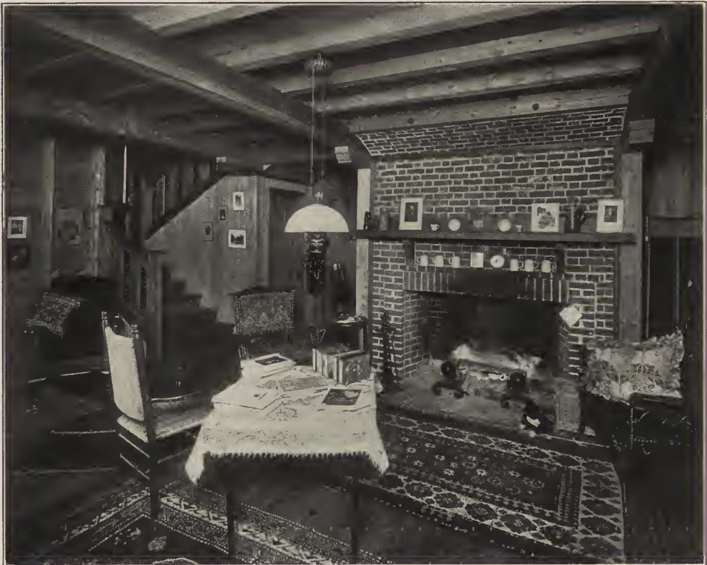
A COMPOSITION OF LIVING ROOM AND STAIRCASE, IN WHICH THE KEYNOTE IS A FRANKNESS IN THE USE OF WOOD.
