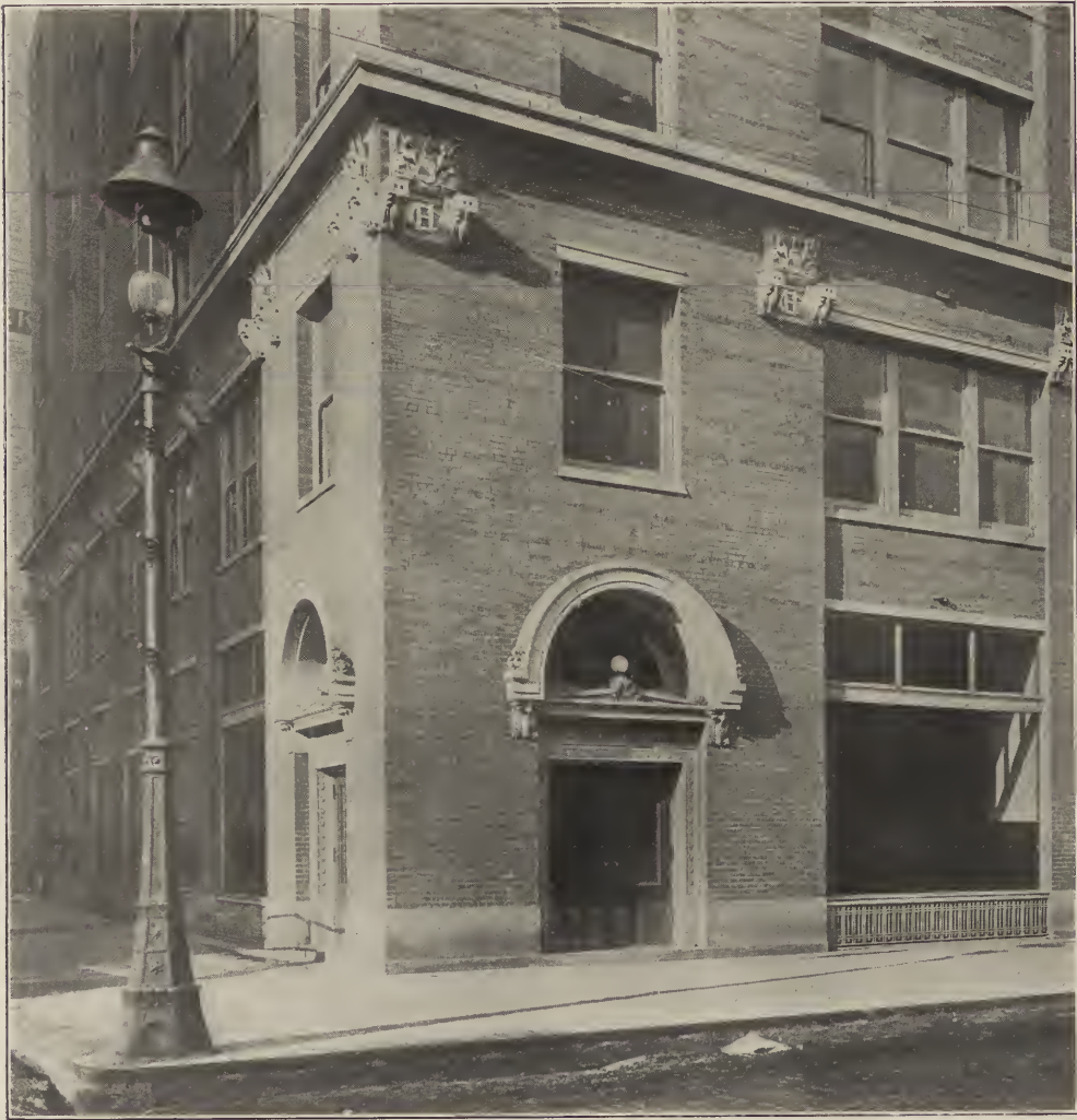
FIG. 6. THE CARTER & HOLMES WAREHOUSE—DETAIL.
