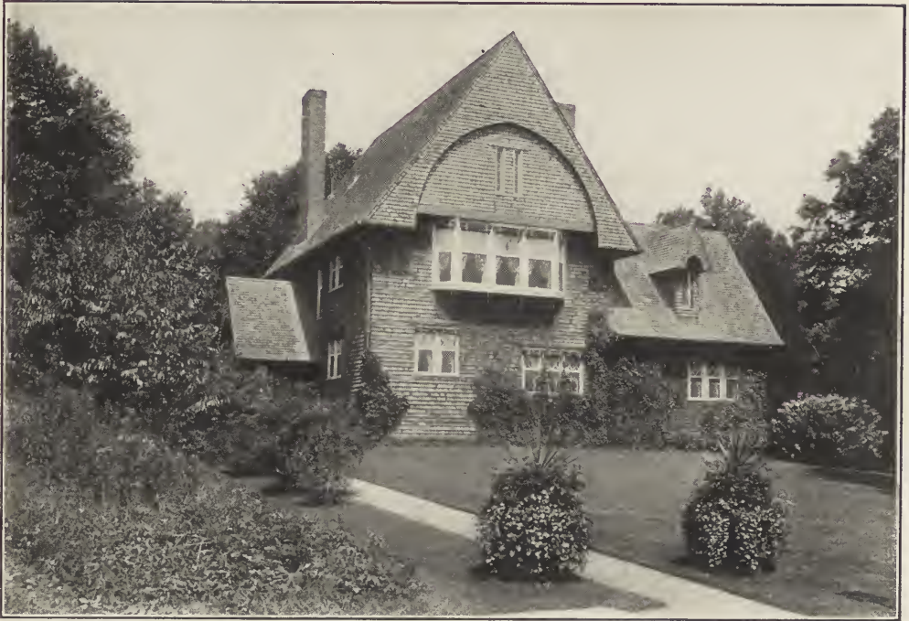
FIG. 6. HOUSE OF HENRY V. KIRBY, ARCHITECT. South Orange, N. J.
