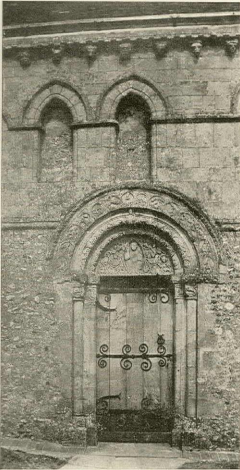
Fig. 152. South Doorway, Barfreston Church.
