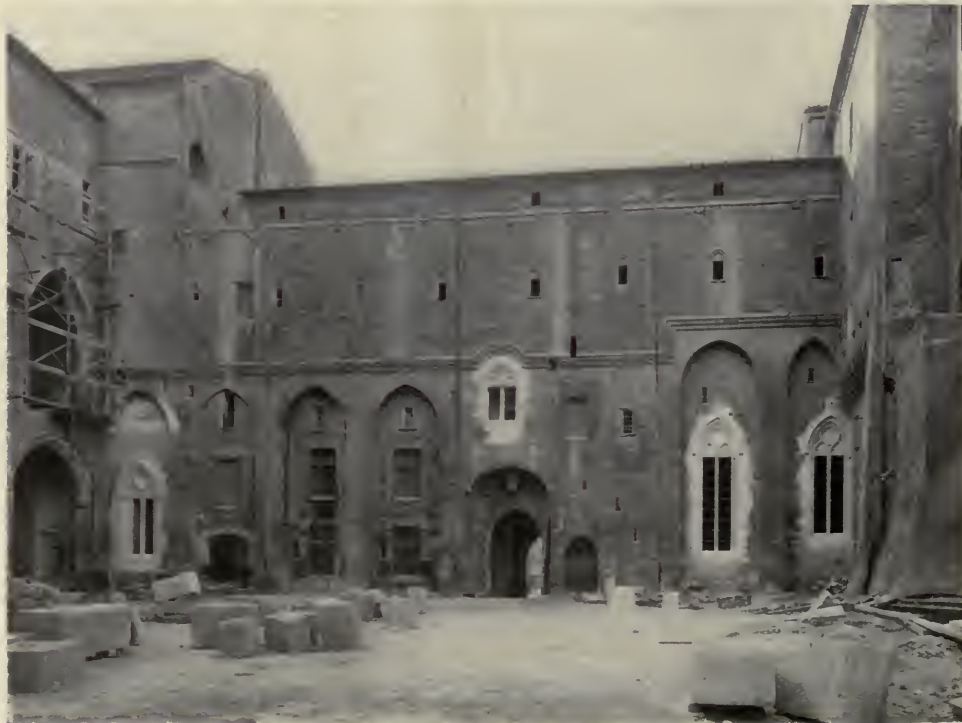
WESTERN FAÇADE FACING COURTYARD.
