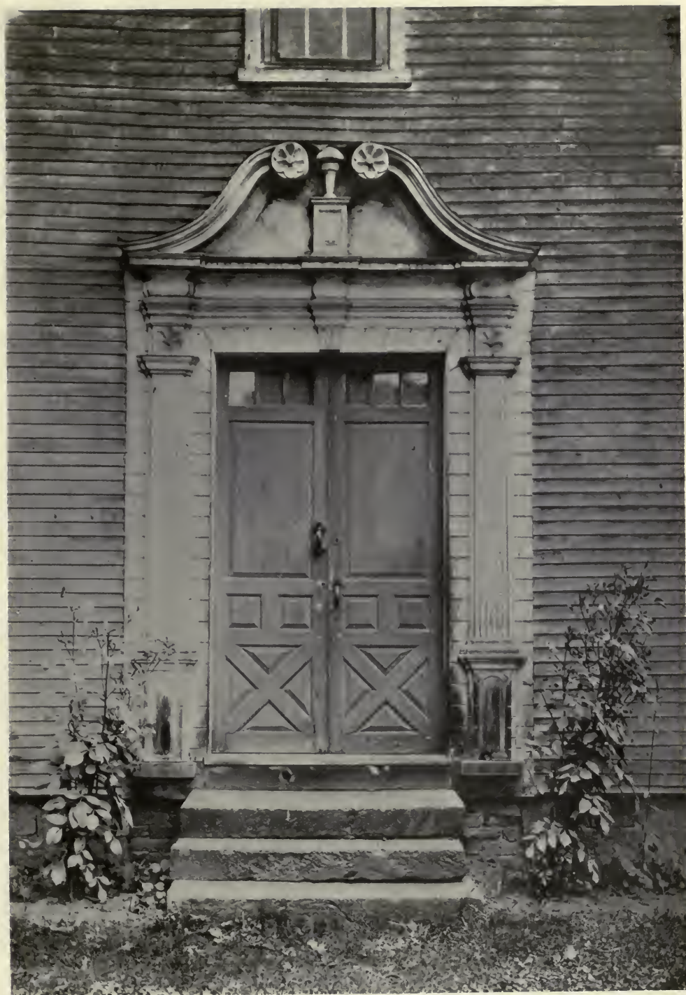
An ambitious Deerfield door which claims to have been built in 1750, the same year as the house, but is probably several decades later. It is a wooden copy of Georgian stone work even to the voussoirs. The broken pediment here used, became later a great favorite with Colonial builders and was much improved upon.
