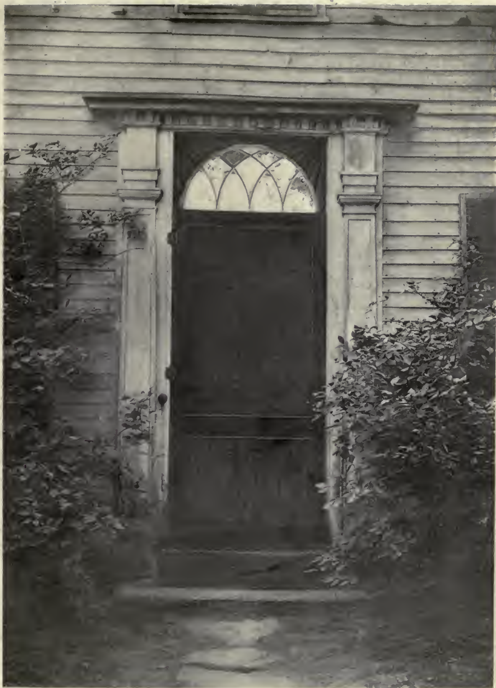
A 1770 entrance in Deerfield. The very extenuated doorway would appear less so if the spandrels over the arch had been painted white instead of dark, as no doubt they were originally. It is interesting to note that even in this unpretentious doorway, the pilasters have a most subtle entasis.
