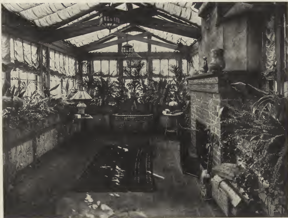
SOLARIUM IN THE RESIDENCE OF H. P. DAVISON, ESQ., NEW YORK CITY. Walker & Gillette, Architects.
