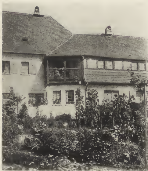
DETAIL OF ARTISAN'S HOUSES, HELLERAU. Prof. Richard Riemerschmid, Architect.
