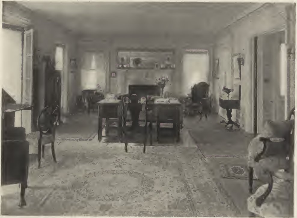
FIG. 1. THE ABSENCE OF CEILING FIXTURES IS SOMETIMES A RELIEF. GENERAL LIGHTING CAN BE OBTAINED BY PLACING ONE OR TWO LIGHTS WITHIN ARCHITECTURAL PROJECTIONS.
