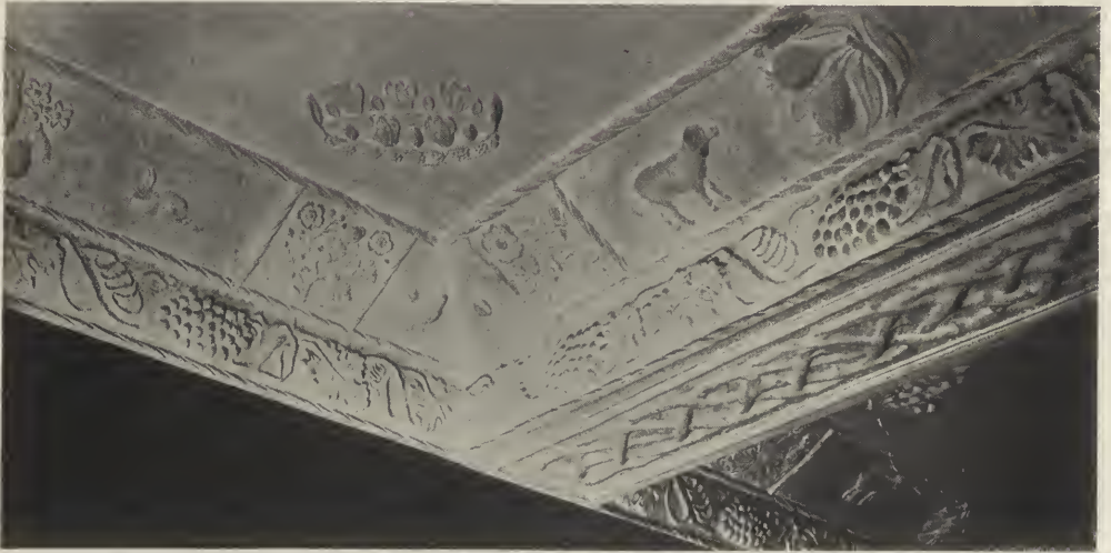
DETAIL OF FIGURED PLASTER CEILING. THE SACRISTY. ST. THOMAS' CHURCH, NEW YORK CITY. Cram, Goodhue & Ferguson, Architects.
