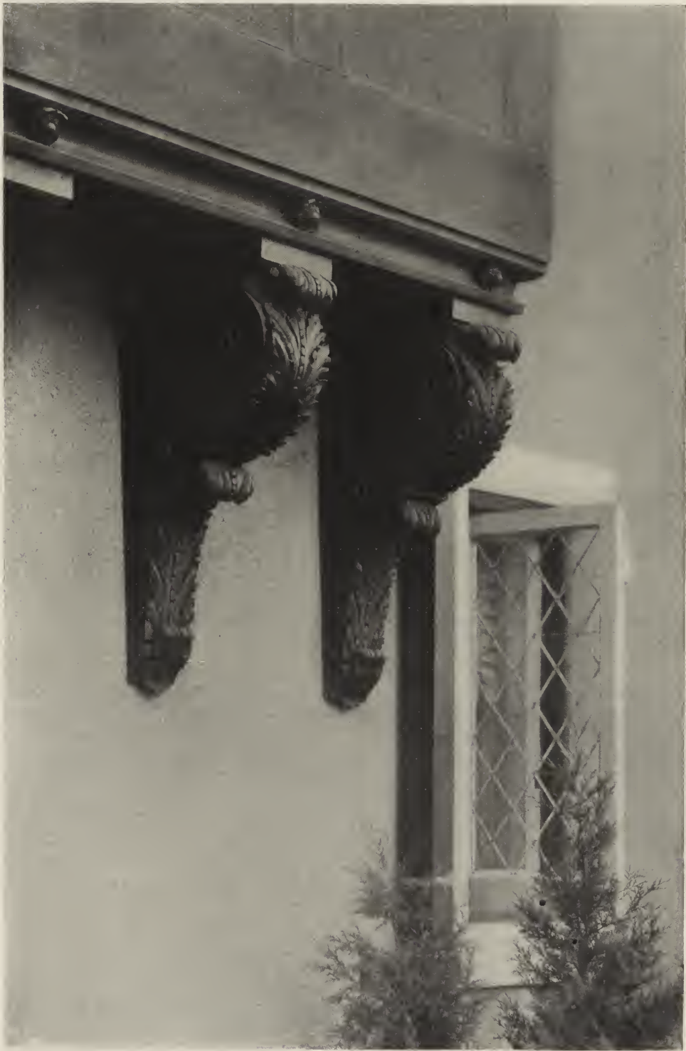
DETAIL OF CARVED WOOD BRACKETS, RESIDENCE OF J. A. GARVER, ESQ., OYSTER BAY, L. I. STEPHENSON & WHEELER, ARCHITECTS.
