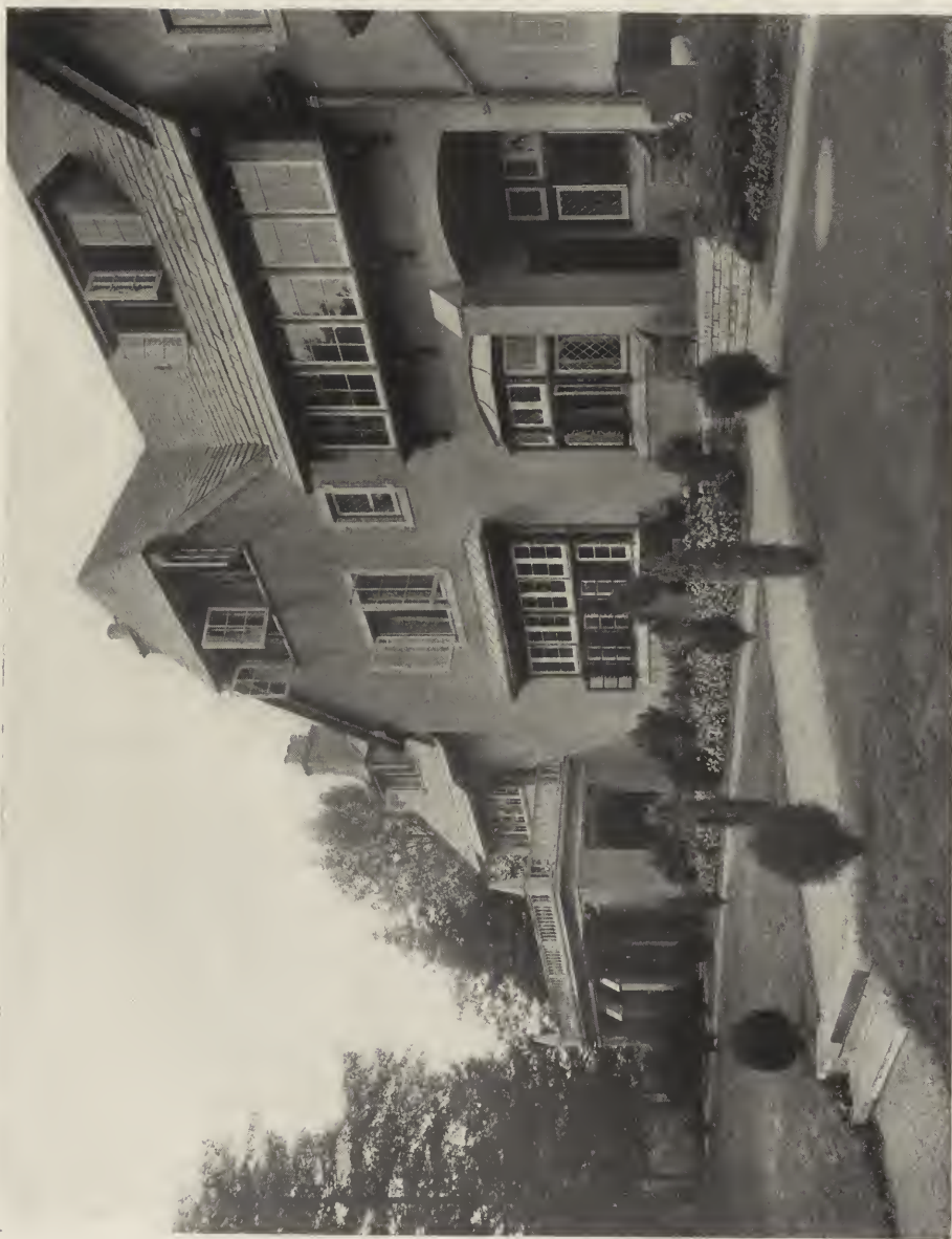
PORTION OF THE GARDEN FRONT, RESIDENCE OF J. A. GARVER, ESQ., OYSTER BAY, L. I. STEPHENSON & WHEELER, ARCHITECTS.
