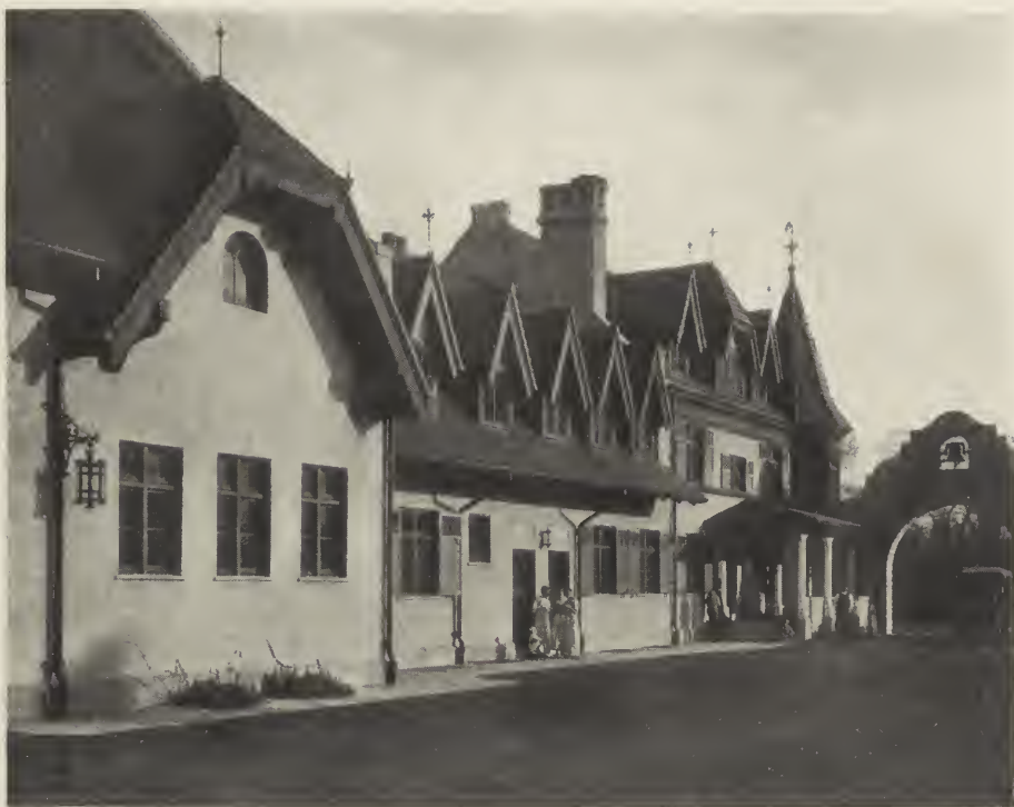
DWELLINGS—THE "BAUERNHOF," ON THE ESTATE OF AUGUST A. BUSCH, NEAR ST. LOUIS, MO. Klipstein & Rathmann, Architects.
