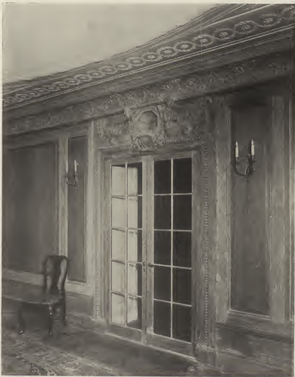
A DOOR DETAIL—HOTEL BILTMORE, NEW YORK CITY. Warren & Wetmore, Architects.
