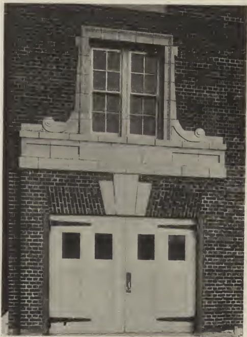
ENTRANCE TO CHEMICAL ENGINE ROOM, NELA PARK, CLEVELAND, OHIO. Wallis & Goodwillie, Architects.
