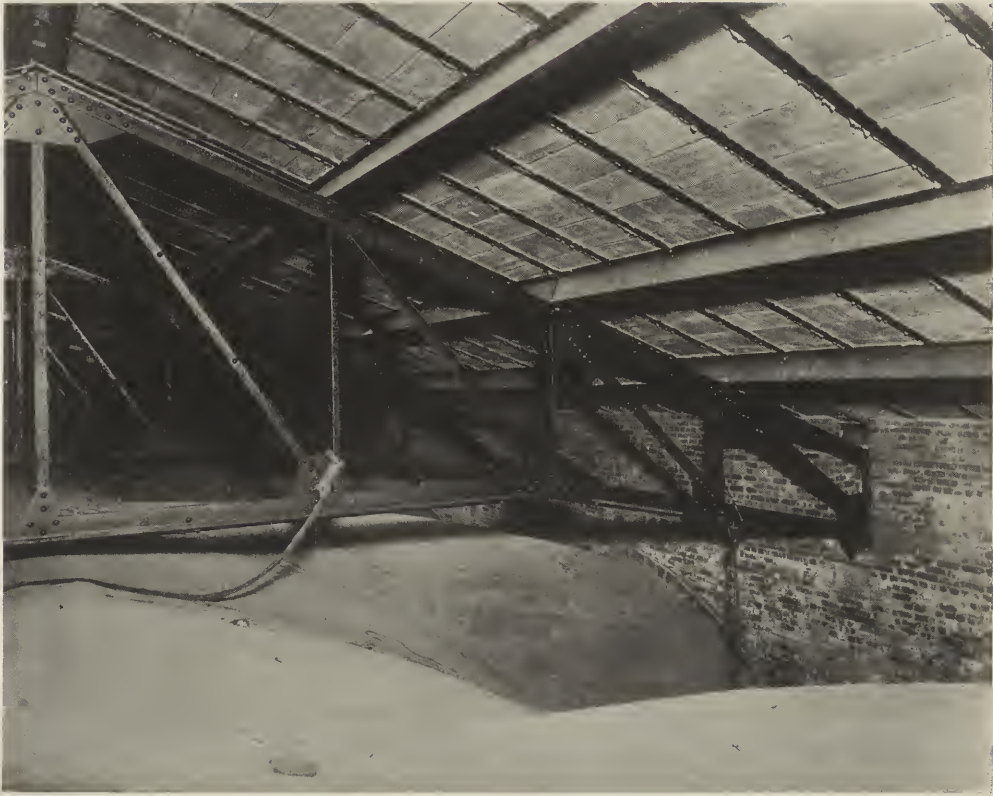
AN INTERESTING CONSTRUCTION PHOTOGRAPH OF ST. THOMAS' CHURCH, NEW YORK CITY.
