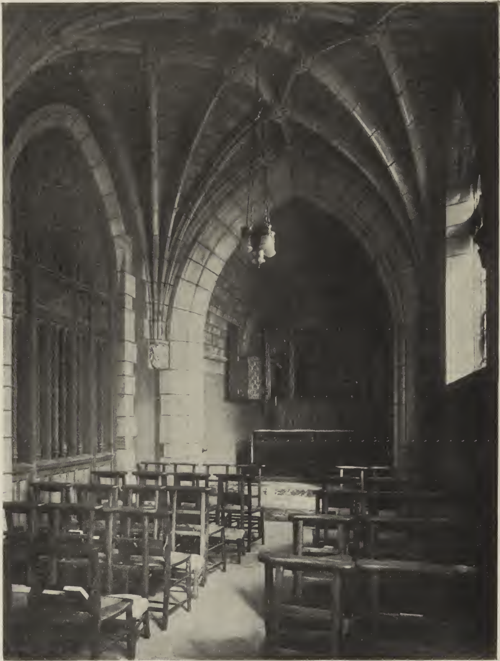
MORNING CHAPEL—CHAPEL OF THE INTERCESSION, NEW YORK. ARCHITECT, BERTRAM GROSVENOR GOODHUE. (Cram, Goodhue & Ferguson.)
