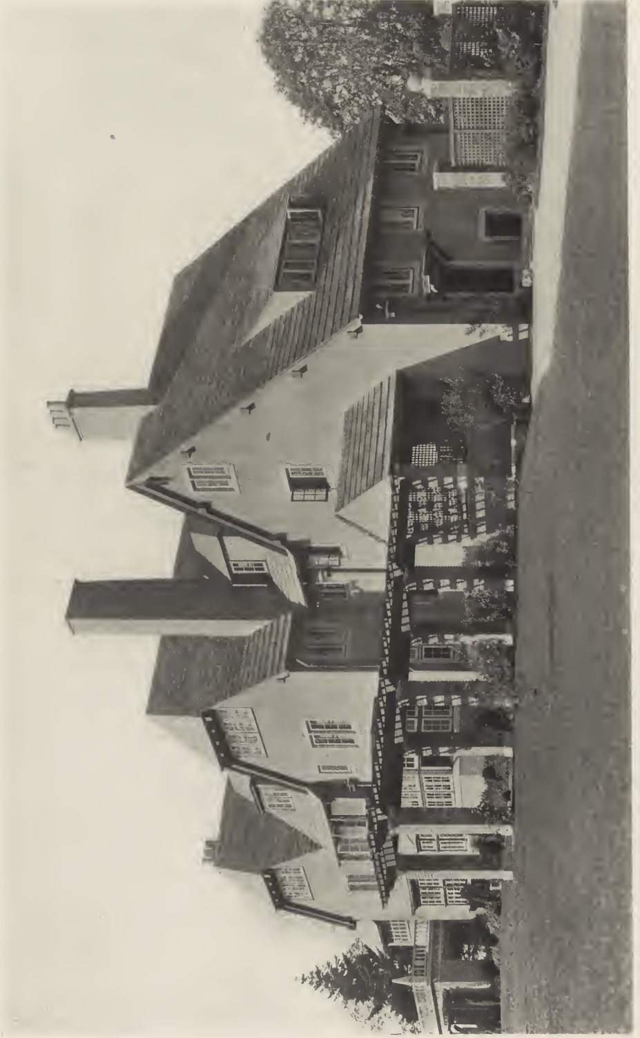
GARDEN FRONT AND SERVICE ENTRANCE, RESIDENCE OF J. A. GARVER, ESQ., OYSTER BAY, L. I. STEPHENSON & WHEELER, ARCHITECTS.
