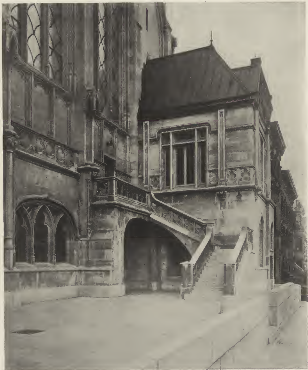
STAIR DETAIL—QUEEN OF ALL SAINTS CHAPEL, BROOKLYN, N. Y. Reiley & Steinback, Architects.
