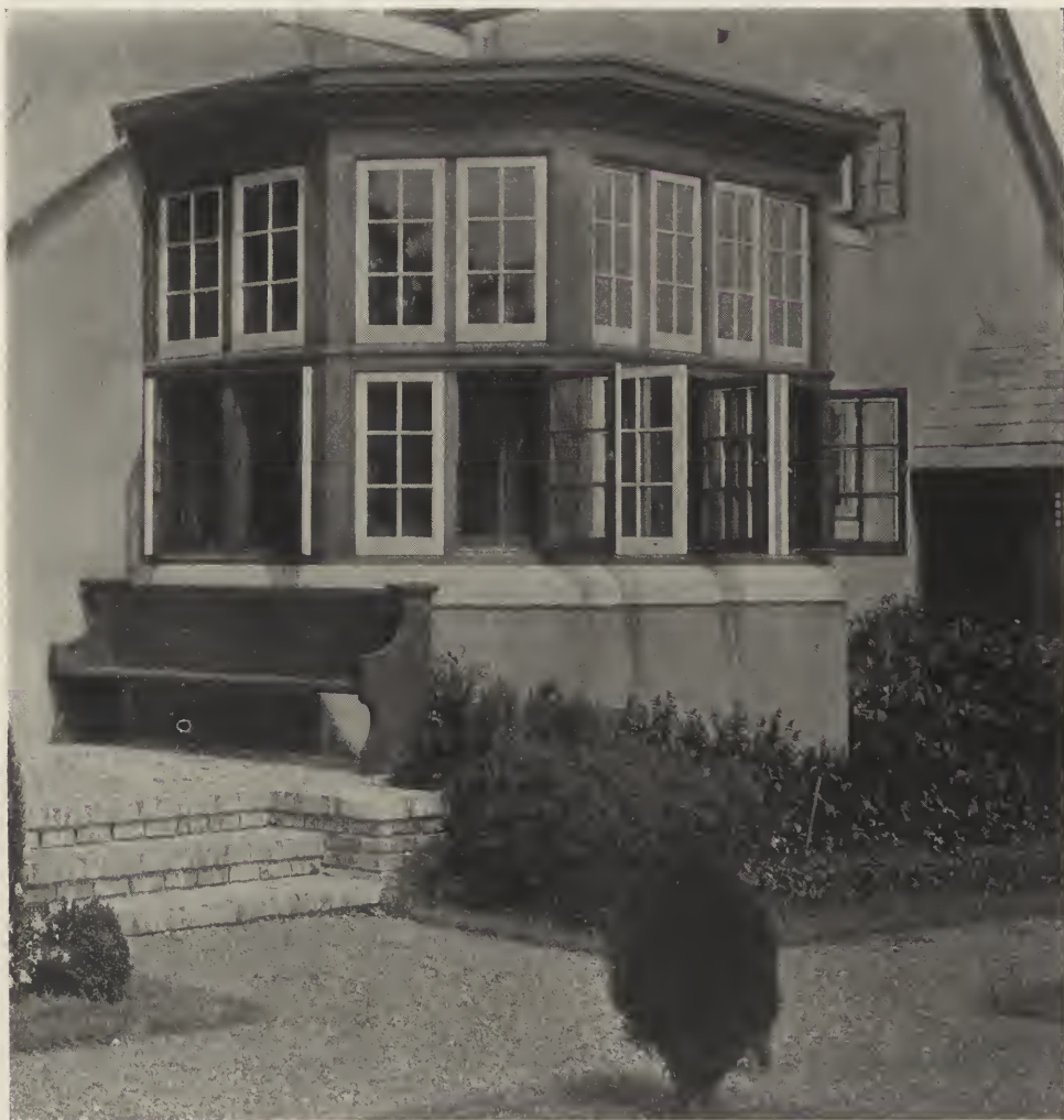
DETAIL OF THE DINING ROOM BAY, RESIDENCE OF J. A. GARVER, ESQ., OYSTER BAY, L. I. Stephenson & Wheeler, Architects.
