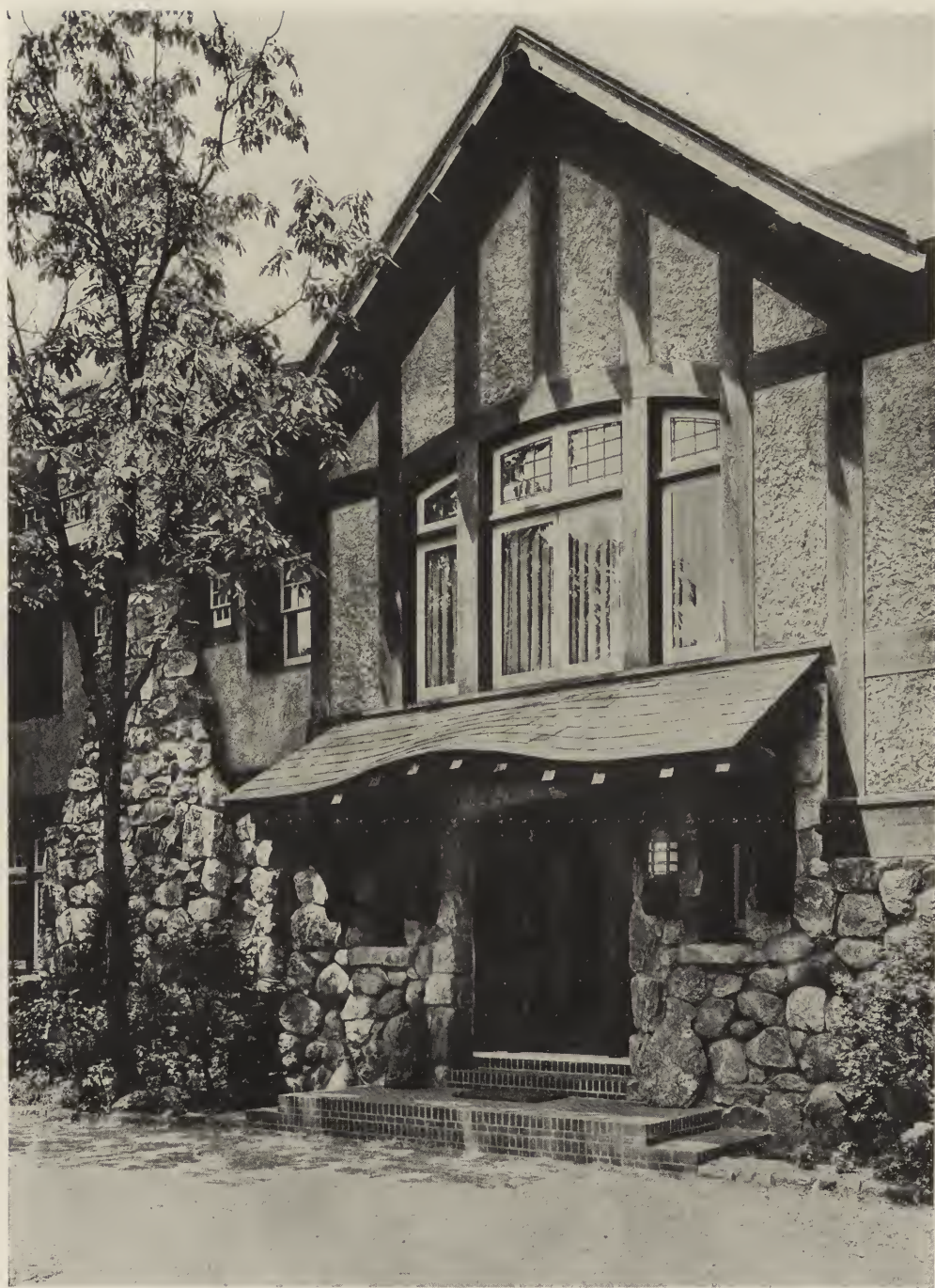
ENTRANCE DETAIL, RESIDENCE OF MISSES SCOFIELD, TUXEDO PARK, N. Y., WALKER & GILLETTE, ARCHITECTS.
