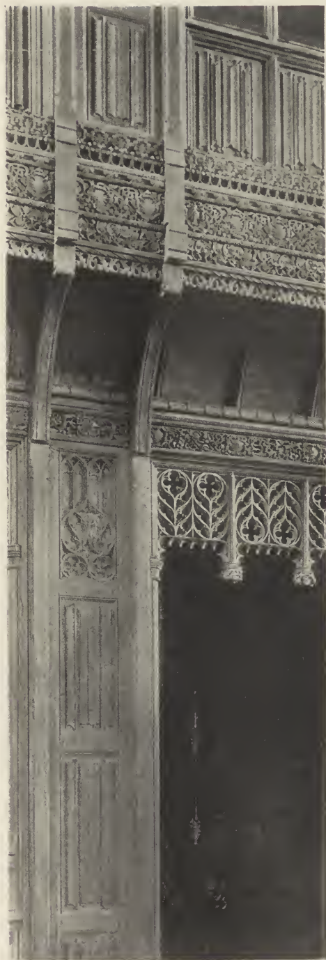
DETAIL OF WOOD SCREEN IN THE GREAT HALL. THE GRADUATE COLLEGE OF PRINCETON UNIVERSITY, PRINCETON, N. J.
