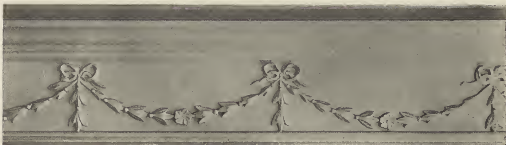
DETAIL OF THE CORNICE IN THE SENATE CHAMBER, CONGRESS HALL, PHILADELPHIA, PA.
