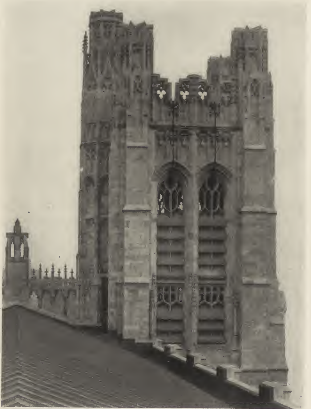
ELEVATION OF THE SQUARE TOWER, ST. THOMAS' CHURCH, NEW YORK CITY. CRAM, GOODHUE & FERGUSON, ARCHITECTS.
