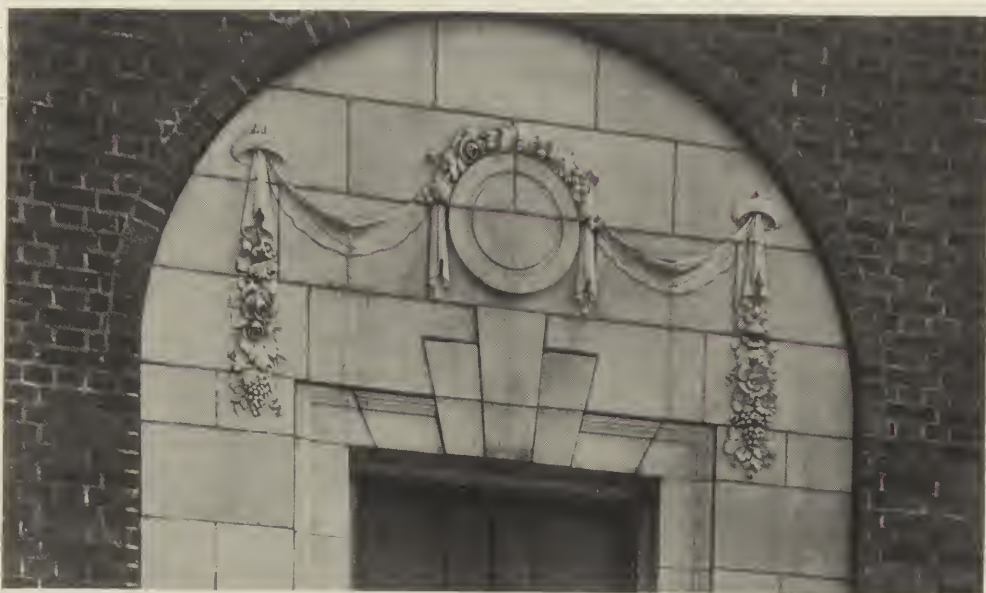
DETAIL OF RESEARCH LABORATORY, NELA PARK, CLEVELAND, OHIO. Wallis & Goodwillie, Architects.
