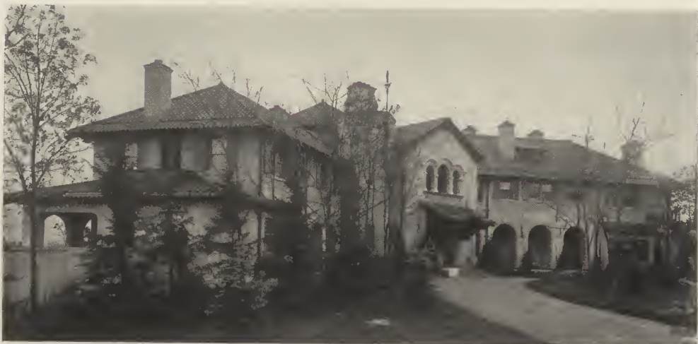
THE ENTRANCE FRONT—RESIDENCE OF JOSEPH E. STEVENS, ESQ., TUXEDO PARK, N. Y. Walker & Gillette, Architects.
