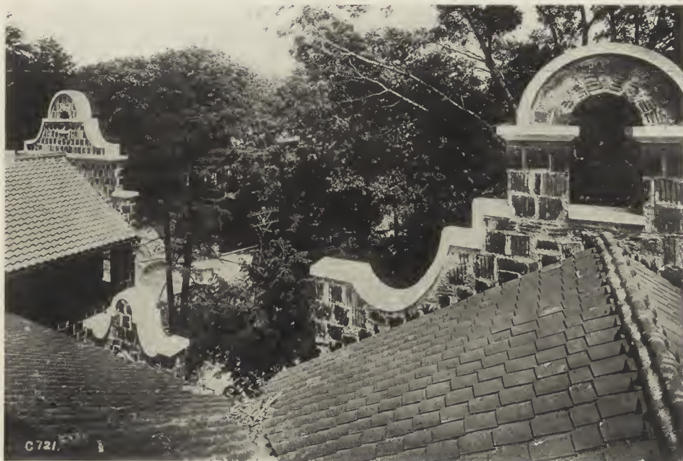
PROGRESS PHOTOGRAPH SHOWING "MISSION" GABLE END, BEFORE STUCCO WAS APPLIED.
