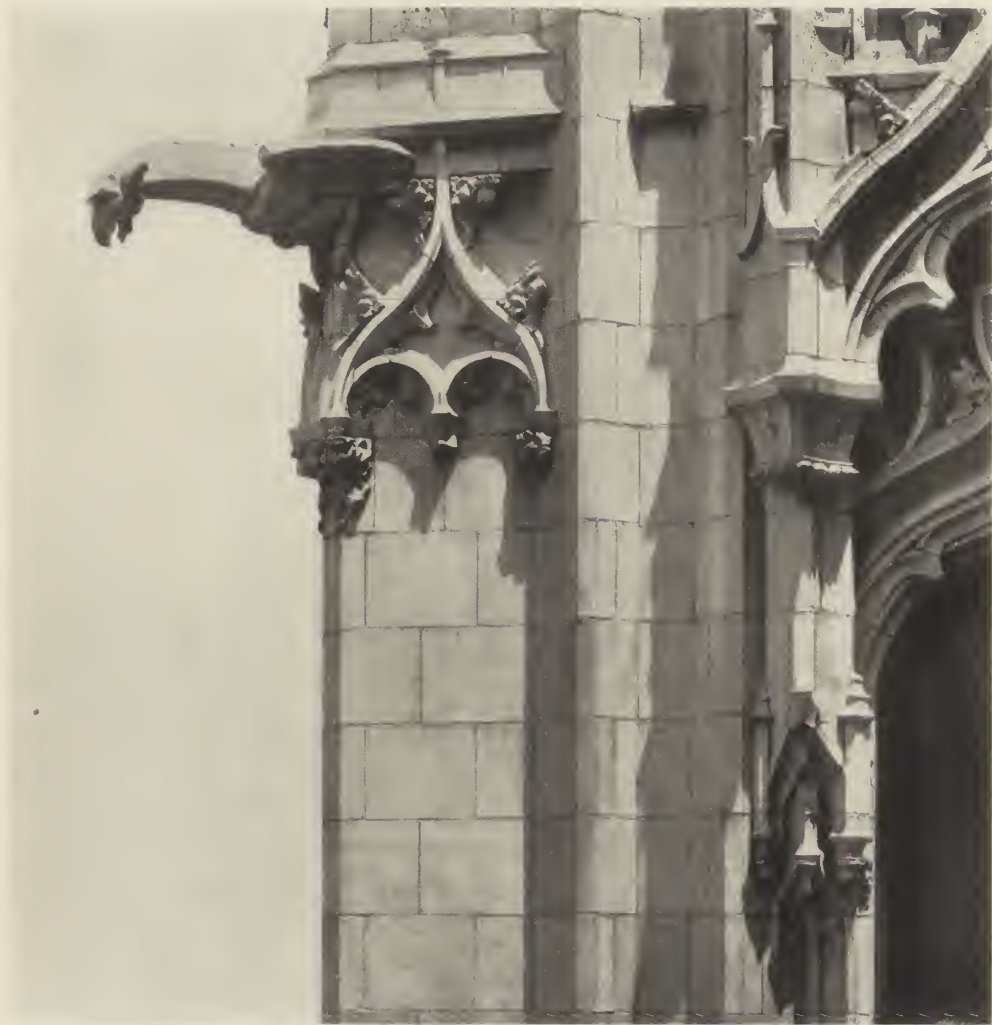
GARGOYLE—DETAIL FROM THE WOOLWORTH BUILDING, NEW YORK CITY. Cass Gilbert, Architect.
