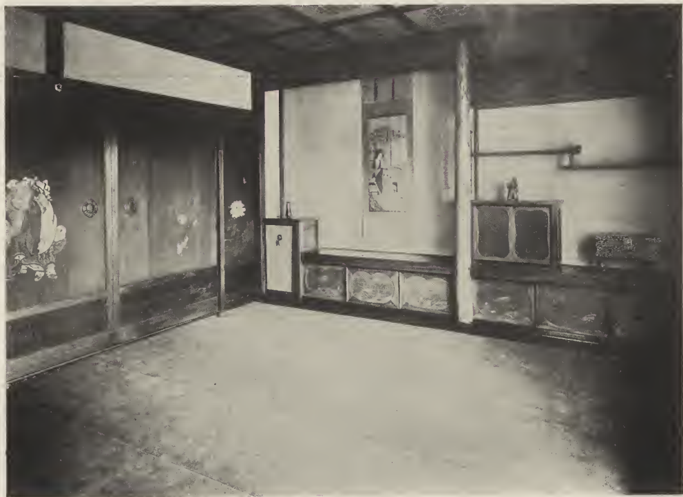
JAPANESE INTERIOR—RESIDENCE OF MISSES SCOFIELD, TUXEDO PARK, N. Y. Walker & Gillette, Architects.
