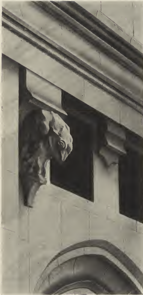
GARGOYLE—DETAIL FROM THE WOOLWORTH BUILDING, NEW YORK CITY. Cass Gilbert, Architect.
