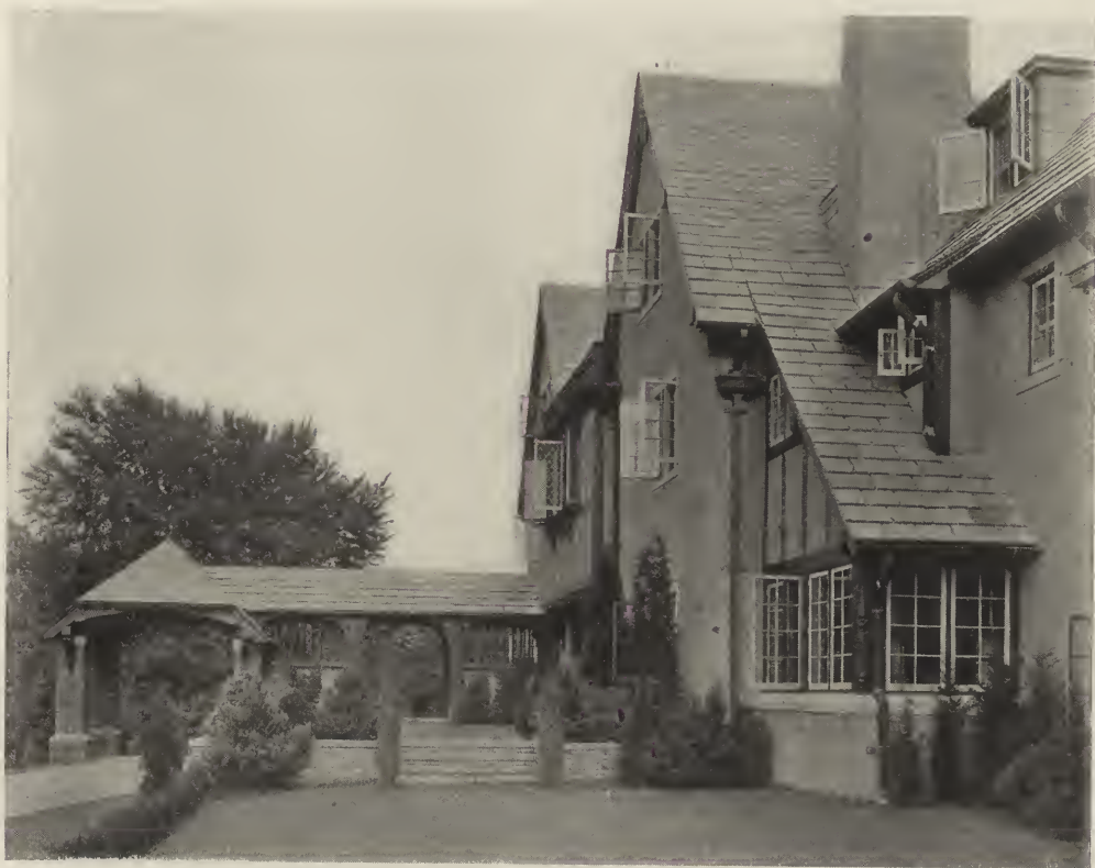
THE ENTRANCE FRONT AND PORTE-COCHERE—RESIDENCE OF J. A. GARVER, ESQ., OYSTER BAY, L. I.
