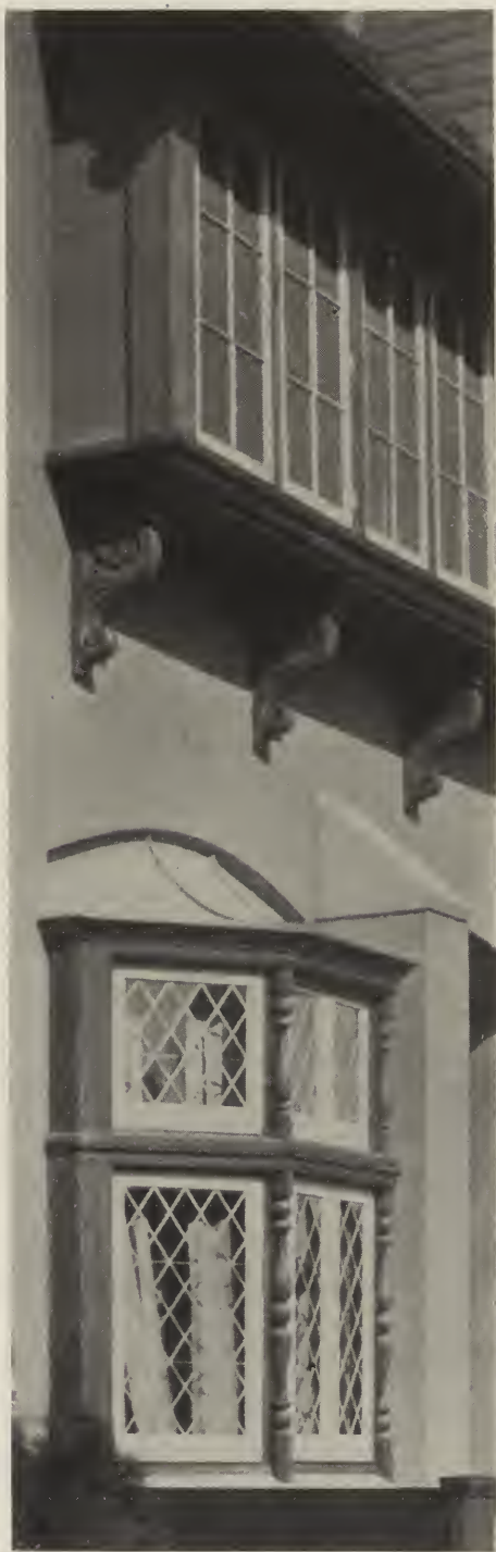
WINDOW DETAIL, RESIDENCE OF J. A. GARVER, ESQ., OYSTER BAY, L. I. STEPHENSON & WHEELER, ARCHITECTS.
