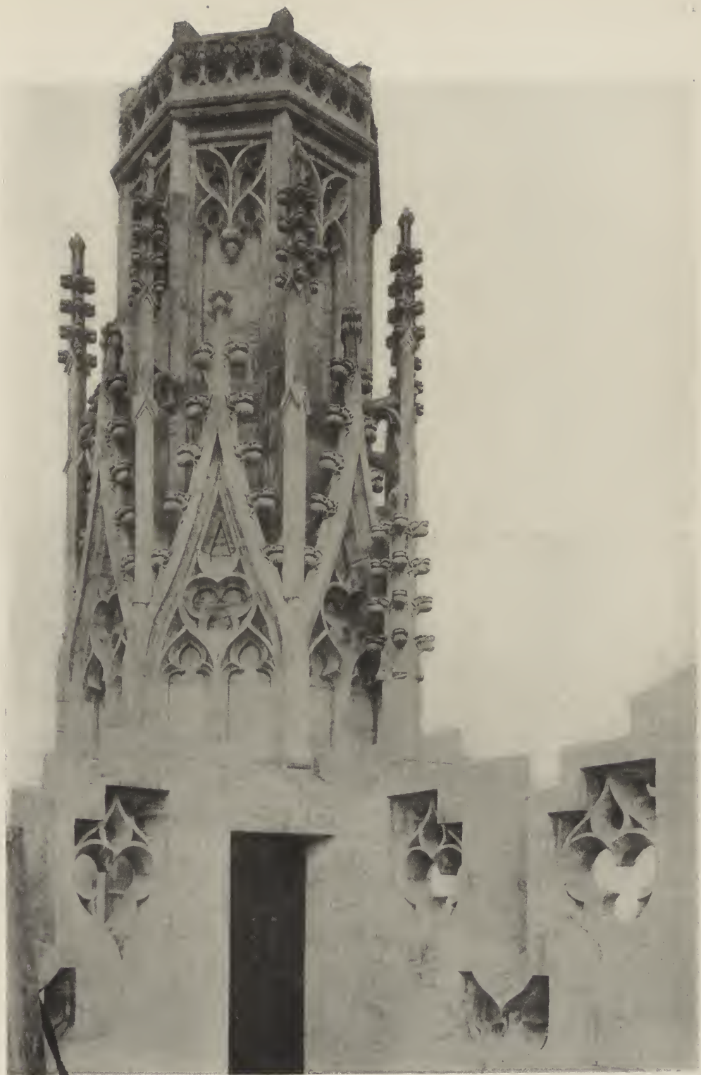
DETAIL OF STAIR TURRET, FROM THE DECK OF THE SQUARE TOWER. ST THOMAS' CHURCH, NEW YORK CITY. CRAM, GOODHUE & FERGUSON, ARCHITECTS.
