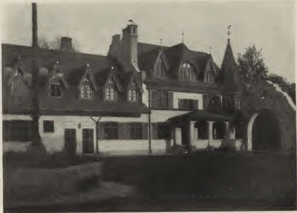
DWELLINGS—THE "BAUERNHOF," ON THE ESTATE OF AUGUST A. BUSCH, NEAR ST. LOUIS, MO. Klipstein & Rathmann, Architects.
