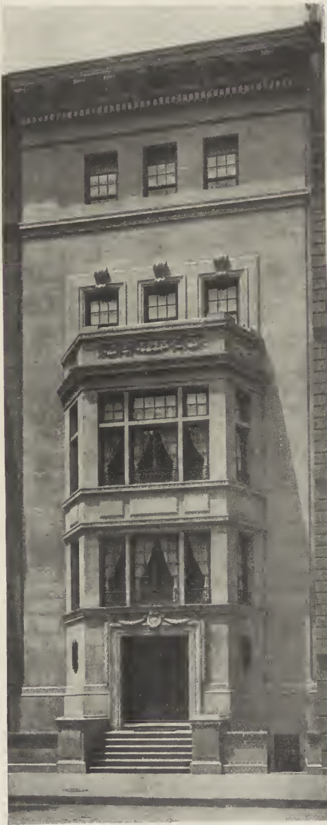
RESIDENCE OF W. G. LOEW, ESQ., NEW YORK CITY. Walker & Gillette, Architects.
