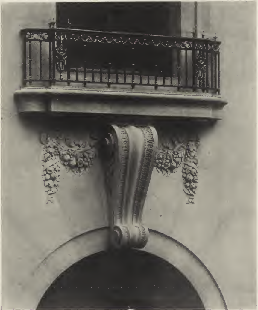
DETAIL—CONSOLE AND WINDOW BALCONY, HOTEL BILTMORE, NEW YORK CITY. Warren & Wetmore, Architects.
