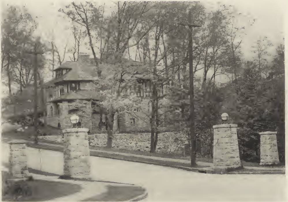
RESIDENCE OF FREDERICK R. A. CAMP, ESQ., AT "FIELDSTON," NEW YORK CITY. Nathaniel Vickers, Architect.
