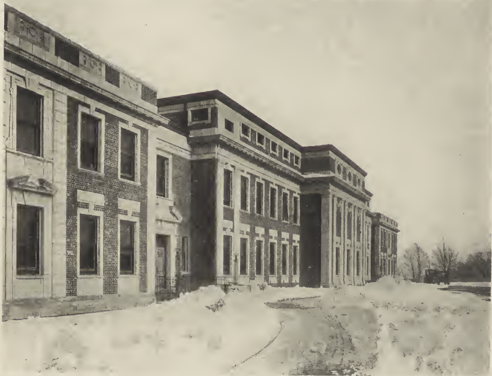
SOUTH SIDE OF ENGINEERING LABORATORY, NELA PARK, CLEVELAND, OHIO. Wallis & Goodwillie, Architects.
