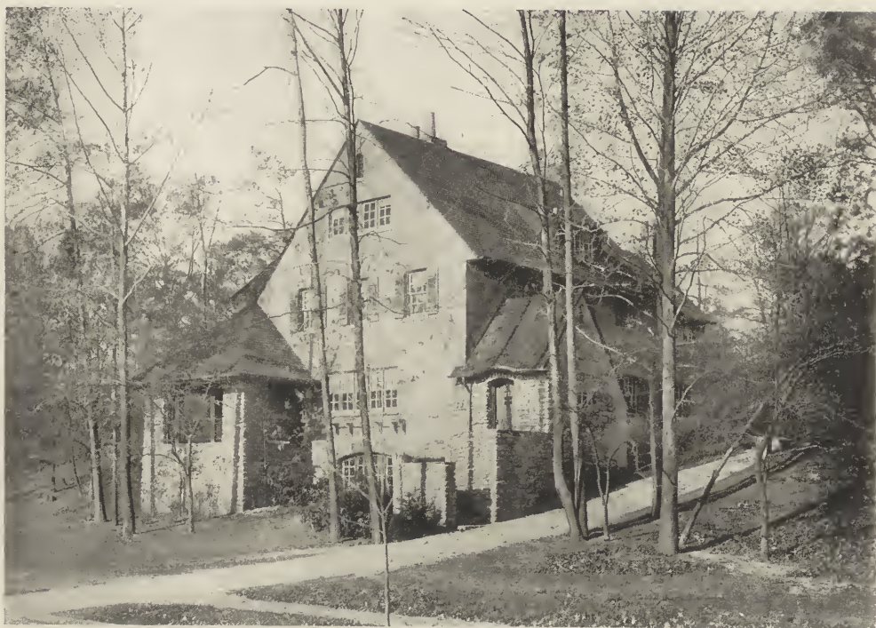
RESIDENCE OF NICHOLAS KELLEY, ESQ., AT "FIELDSTON," NEW YORK CITY. Harrie T. Lindeberg, Architect.
