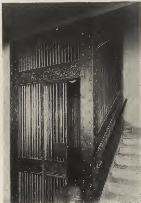
DETAIL OF WROUGHT ELEVATOR GRILLE IN THE PARISH HOUSE. ST. THOMAS' CHURCH, NEW YORK CITY. Cram, Goodhue & Ferguson, Architects.
