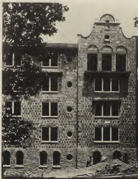
TWO PROGRESS PHOTOGRAPHS, THE FIRST SHOWING THE FLOOR CONSTRUCTION, THE SECOND, A PORTION OF THE EXTERIOR BEFORE THE APPLICATION OF THE STUCCO.
