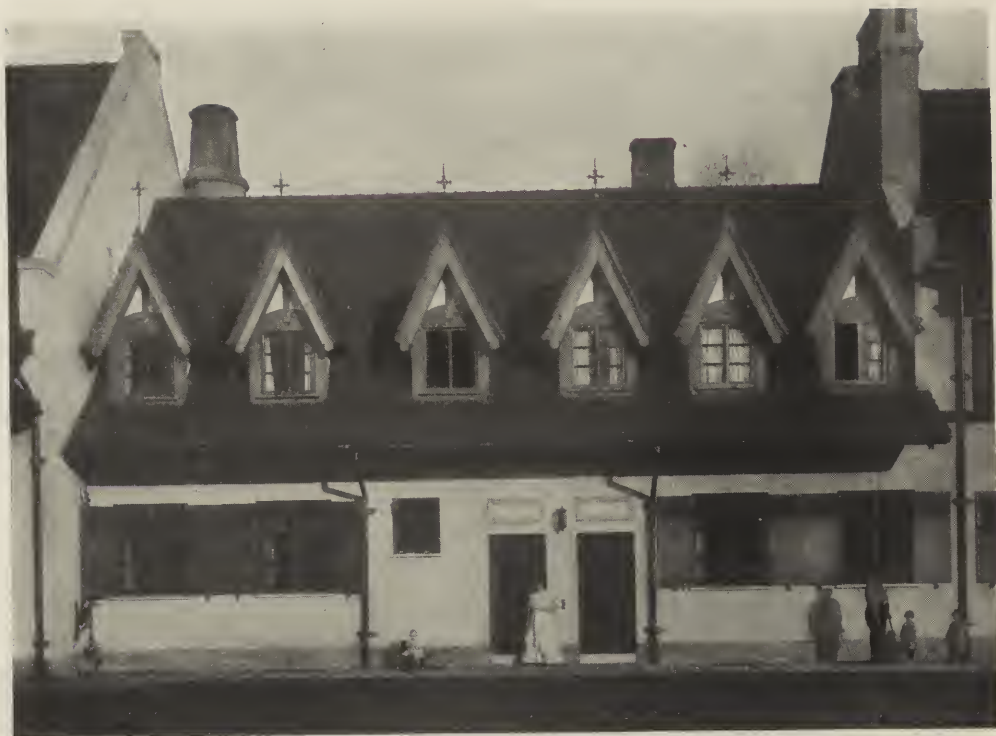
DWELLINGS—THE "BAUERNHOF," ON THE ESTATE OF AUGUST A. BUSCH, NEAR ST. LOUIS, MO. Klipstein & Rathmann, Architects.
