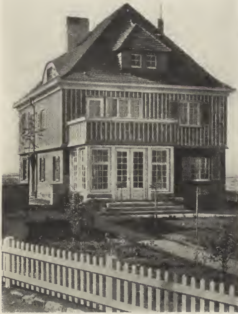
STREET VIEW, ONE-FAMILY HOUSE, HELLERAU Prof. Heinrich Tscherman, Architect.
