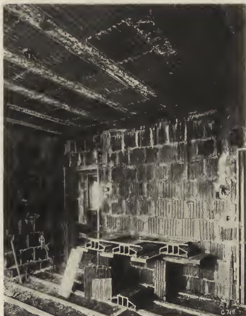
TWO PROGRESS PHOTOGRAPHS, THE FIRST SHOWING THE FLOOR CONSTRUCTION, THE SECOND, A PORTION OF THE EXTERIOR BEFORE THE APPLICATION OF THE STUCCO.
