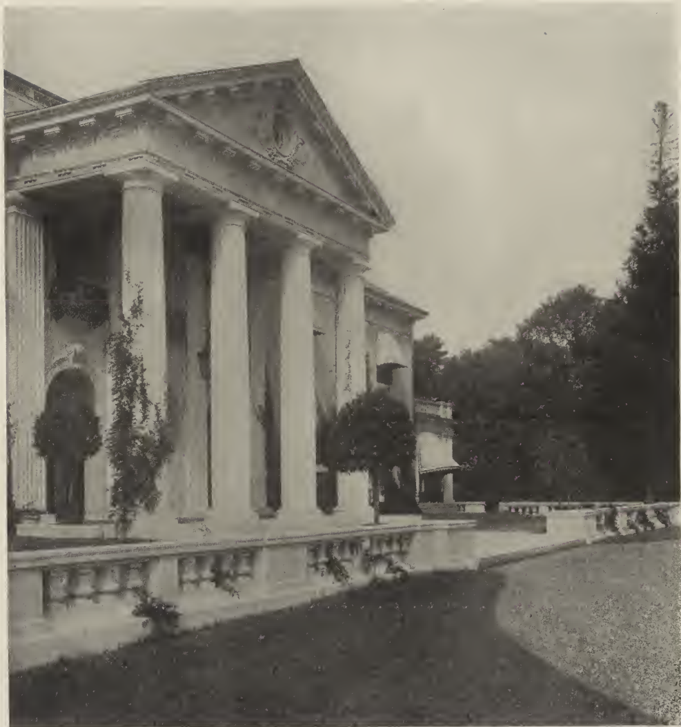
PORTICO—RESIDENCE OF W. M. SALISBURY, ESQ., PITTSFIELD, MASS. Walker & Gillette, Architects.
