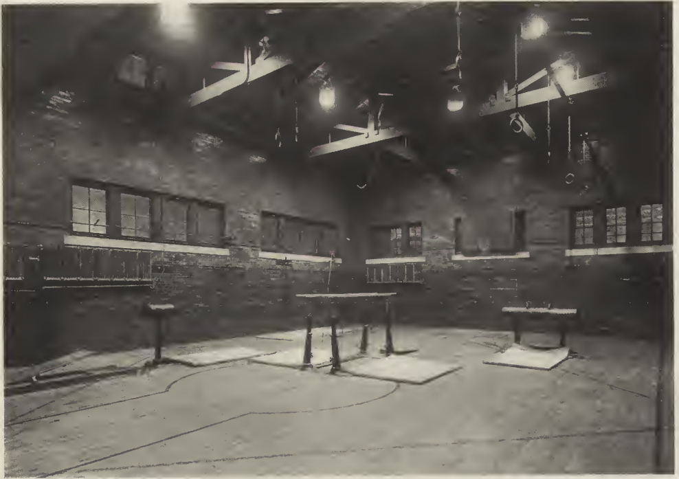
FIG. 10. ANOTHER INSTANCE WHERE LOSS OF LIGHT UPWARD IS ELIMINATED BY UTILIZING OPAQUE REFLECTORS (PROTECTED BY WIRE CAGES). AT SUCH HEIGHTS USE SPACING TO GIVE UNIFORM ILLUMINATION DESIRED.
