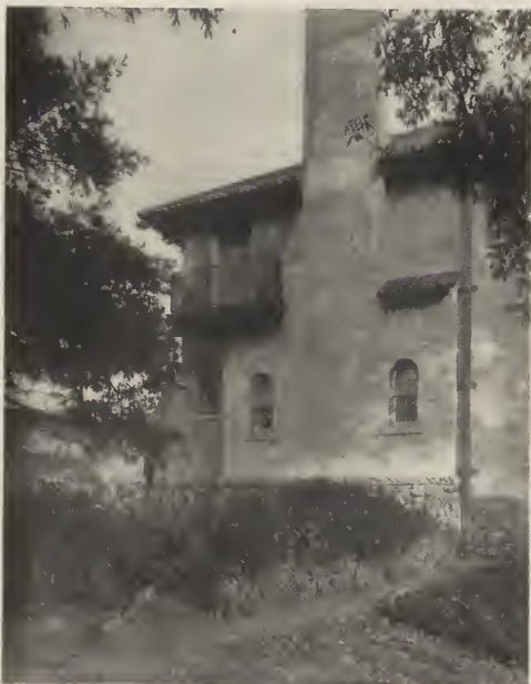
DETAIL—RESIDENCE OF JOSEPH E. STEVENS, ESQ., TUXEDO PARK, N. Y. Walker & Gillette, Architects.
