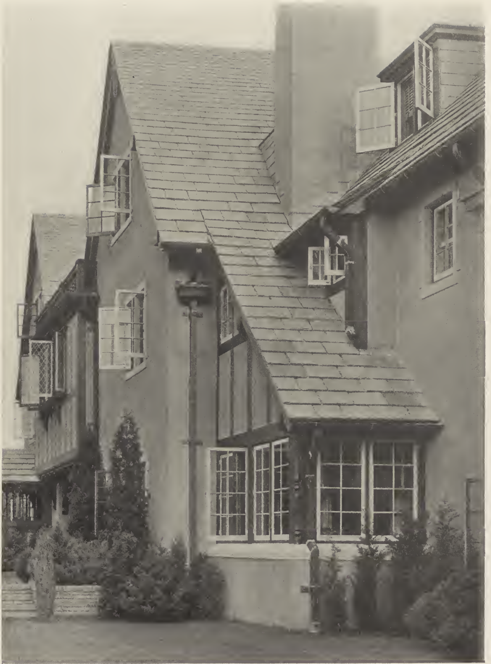
DETAIL—RESIDENCE OF J. A. GARVER, ESQ., OYSTER BAY, L. I. STEPHENSON & WHEELER, ARCHITECTS.
