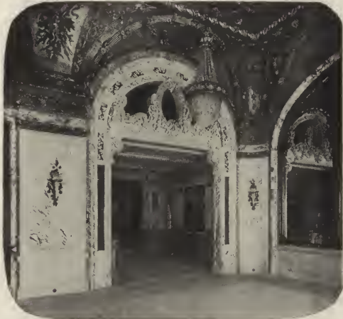
FIG. 7. ANOTHER SUITABLE APPLICATION FOR OPAQUE REFLECTORS. THE LIGHT FLOOR REDIRECTS SUFFICIENT LIGHT UPWARD TO REVEAL THE CEILING ORNAMENTATION.
