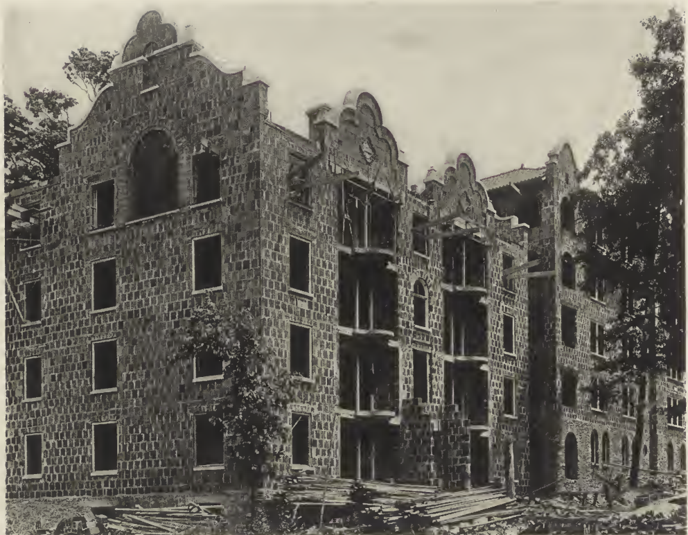
PROGRESS PHOTOGRAPH OF "GRAMATAN COURT," BRONXVILLE, N. Y. Bates & How, Architects.
