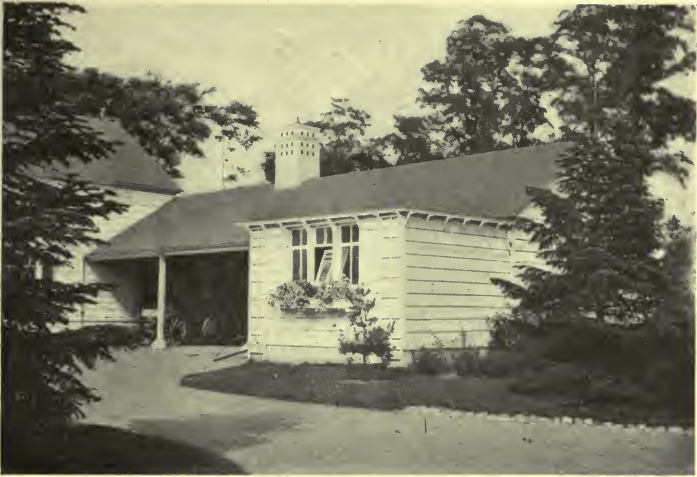
WAGON SHED AND TOOL ROOM—ESTATE OF C. V. BROKAW, ESQ., GLEN COVE, L. I. Alfred Hopkins, Architect.
