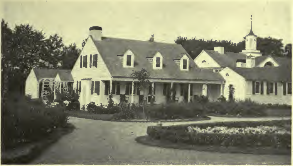
FARMER'S COTTAGE—ESTATE OF C. V. BROKAW, ESQ., GLEN COVE, L. I. Alfred Hopkins, Architect.
