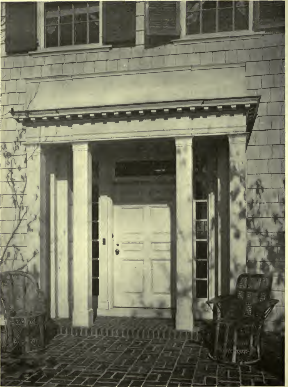
DOORWAY—HOUSE OF GEORGE K. SMITH, ESQ., ST. LOUIS COUNTY, MO. ROTH & STUDY, ARCHITECTS.
