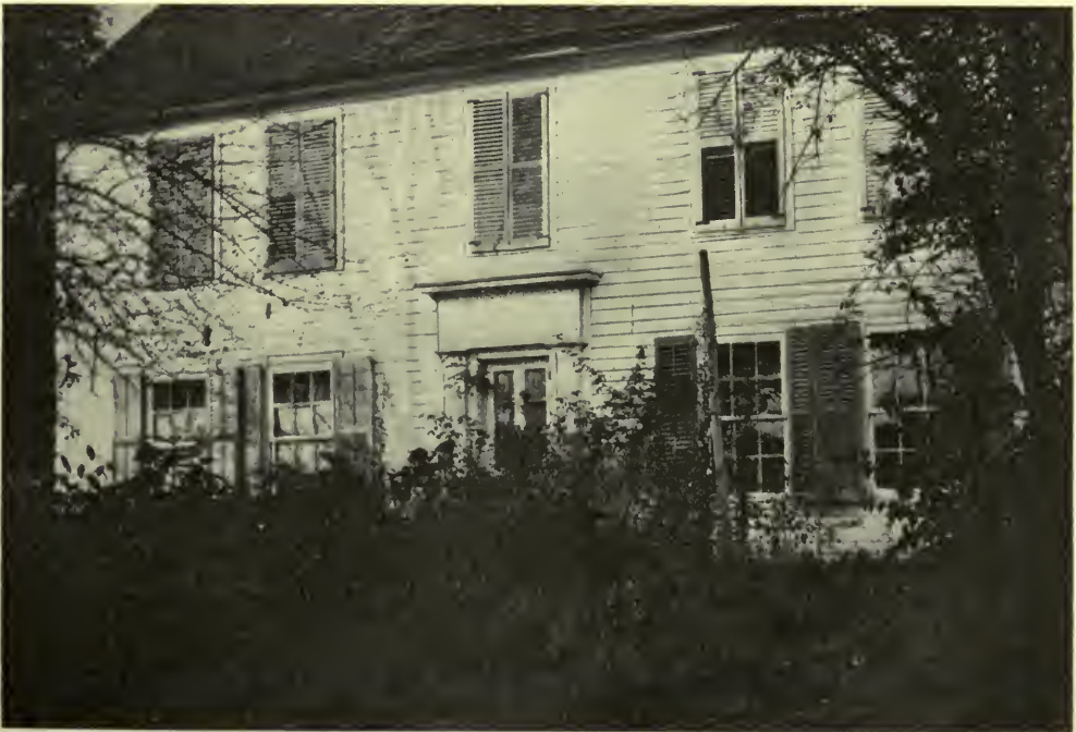
HEZECAH PRATT HOUSE, ESSEX, CONN., BUILT IN 1744. DOOR IS OF LATER DATE.
