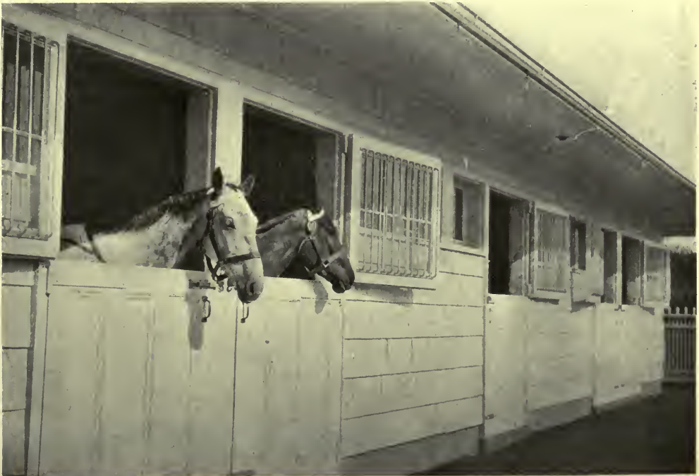
BOX STALL WING OF FARM BUILDINGS—ESTATE OF MRS. GLENN STEWART, LOCUST VALLEY, L. I. Alfred Hopkins, Architect.
