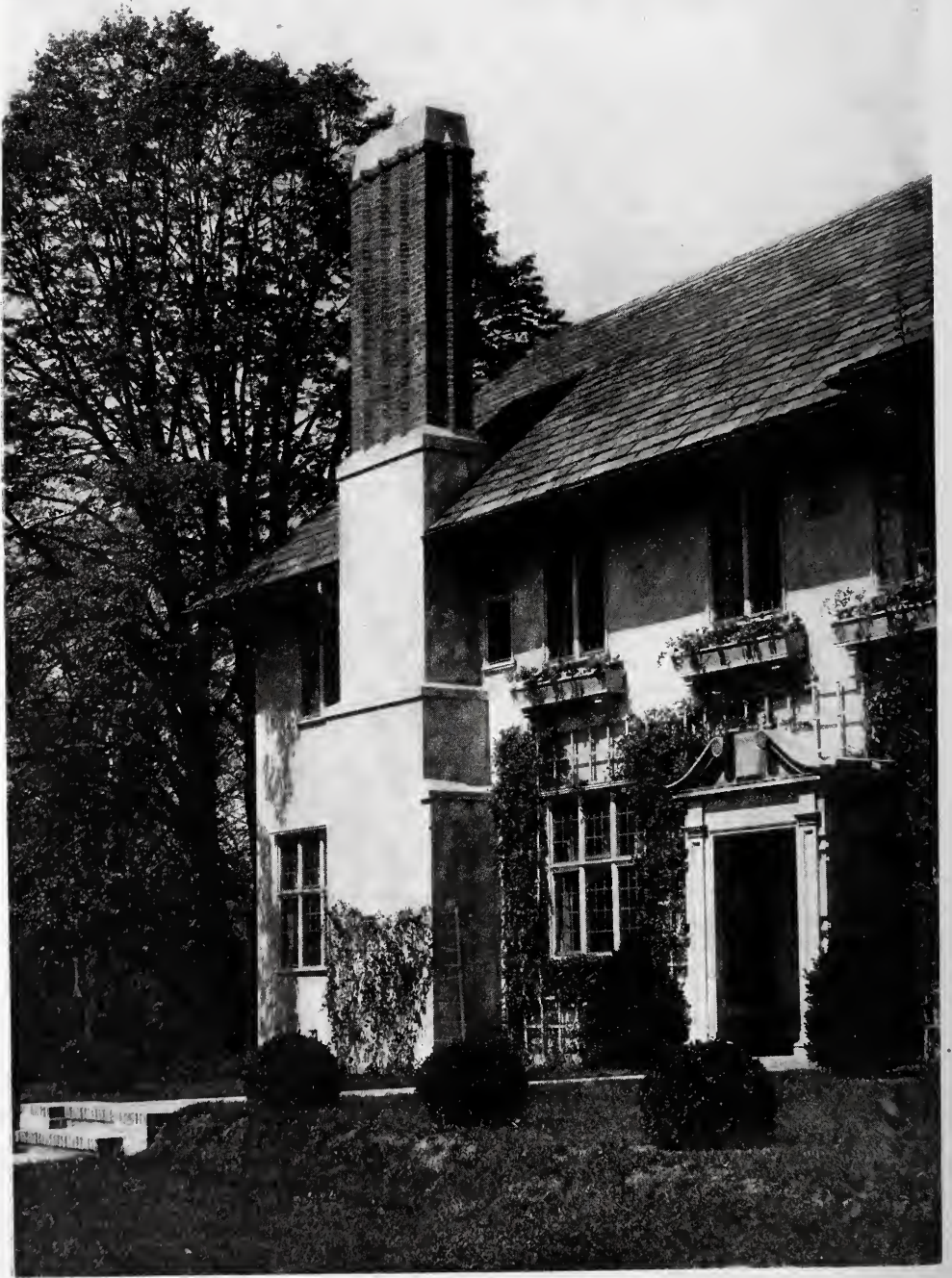
DETAIL—HOUSE OF C. BONYNGE, ESQ., SOUTH ORANGE, N. J. DAVIS, McGRATH & KIESSLING, ARCHITECTS.
