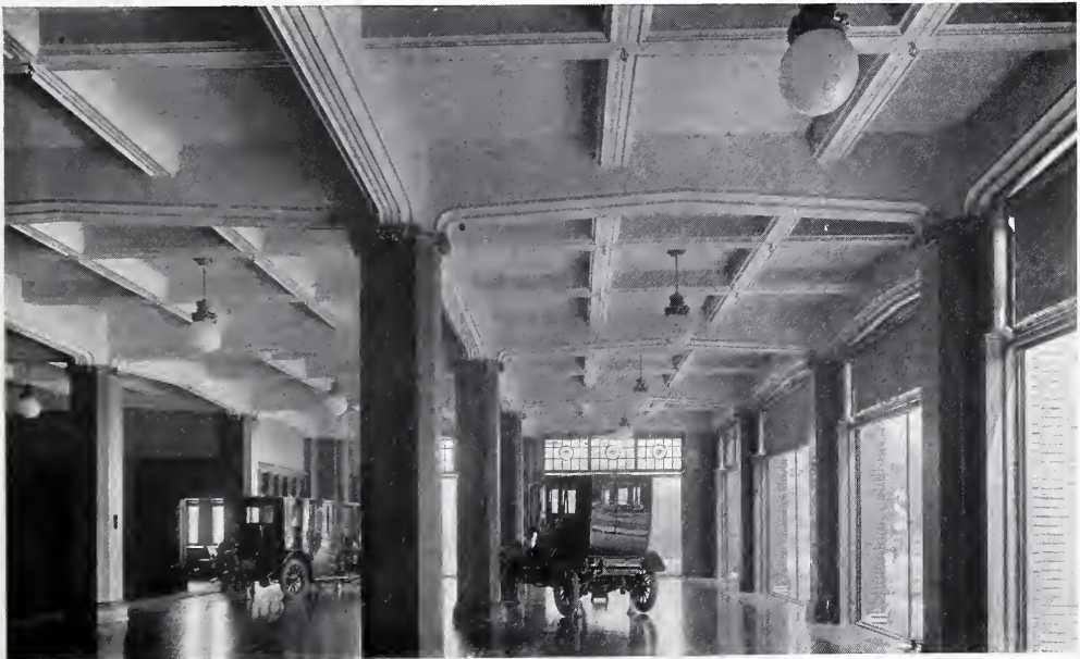
DISPLAY ROOM—BUILDING OF C. P. KIMBALL & CO., CHICAGO. George C. Nimmons, Architect.
