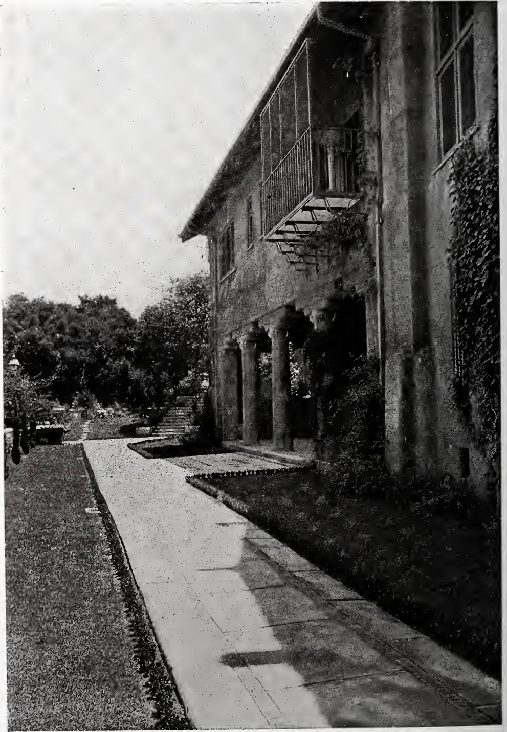
UPPER TERRACE AND LOGGIA—HOUSE OF MISS CORDELIA A. CULBERTSON, PASADENA, CAL. GREENE & GREENE, ARCHITECTS.
