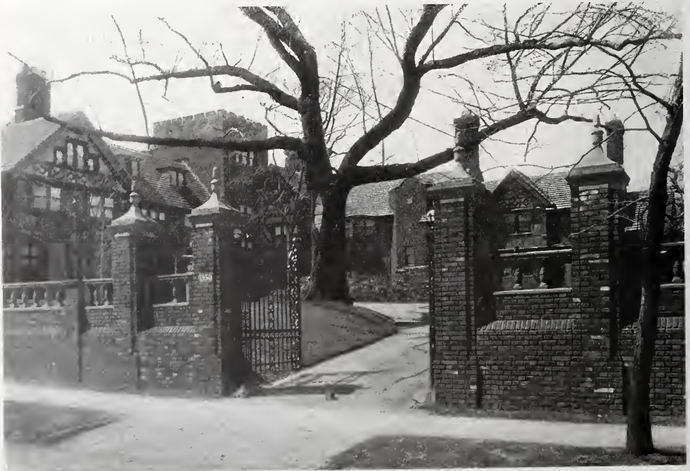
GATEWAY AND COURT—RESIDENCE OF F. E. DRURY, ESQ., CLEVELAND, OHIO. Frank B. Meade and James M. Hamilton, Architects.
