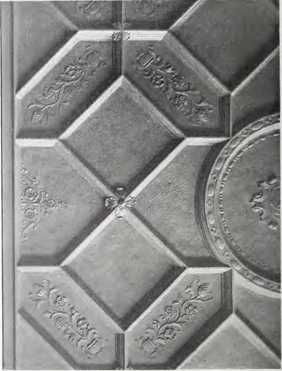
DETAIL OF PLASTER CEILING IN DINING HALL—HARVARD CLUB OF NEW YORK. MCKIM, MEAD & WHITE, ARCHITECTS.
