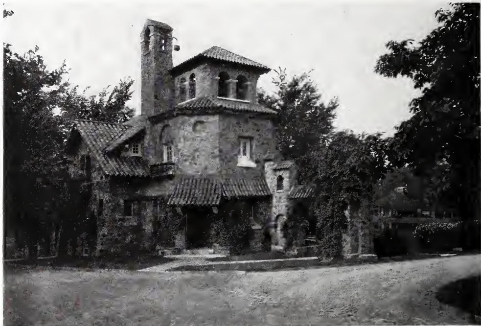
GATE LODGE—ESTATE OF CHARLES S. WALTON, ESQ., ST. DAVIDS, PA. D. Knickerbacker Boyd, Architect.
