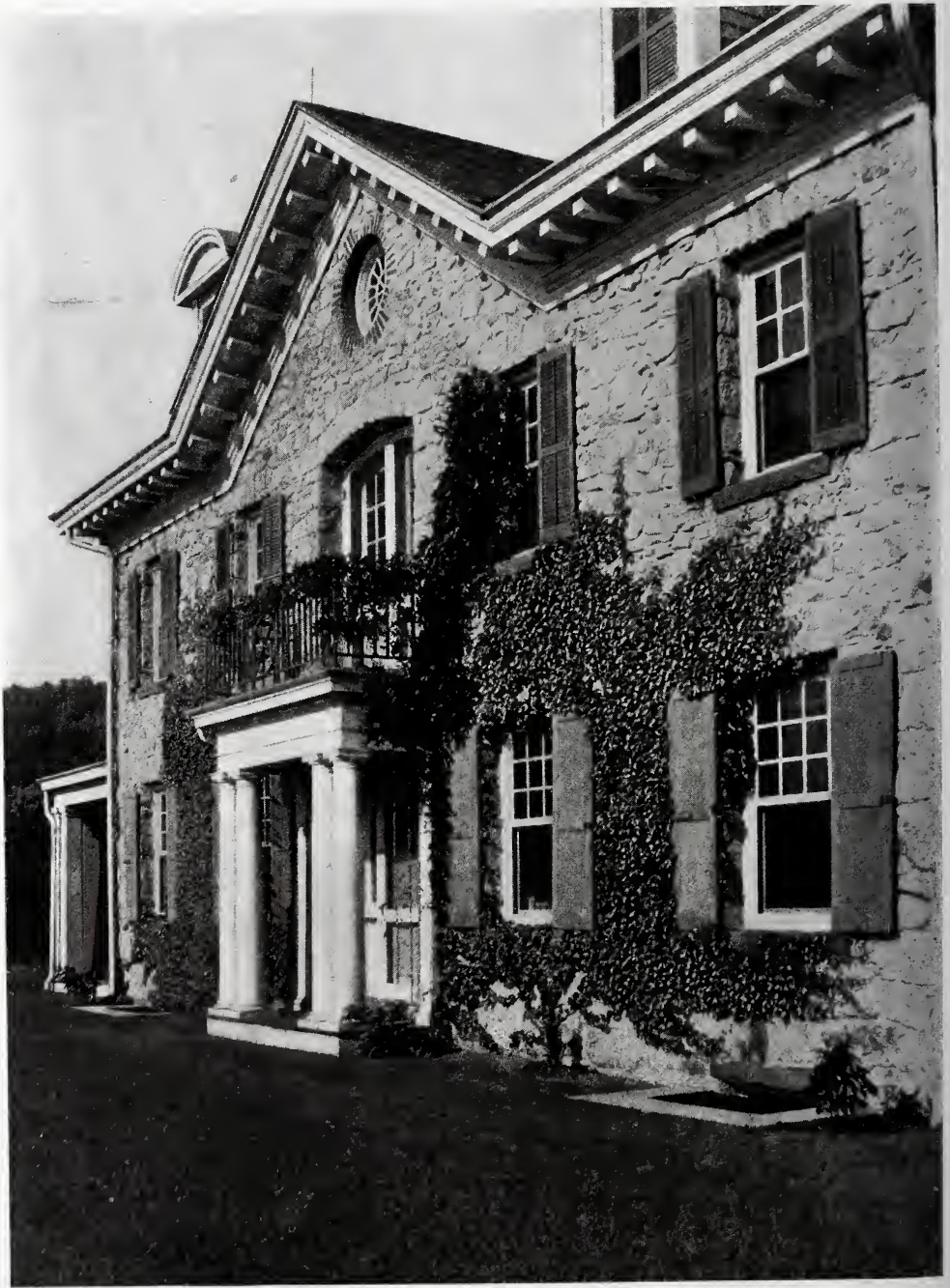
HOUSE OF KNOX TAYLOR, ESQ., HIGH BRIDGE, N. J. WILLIAM EMERSON, ARCHITECT.
