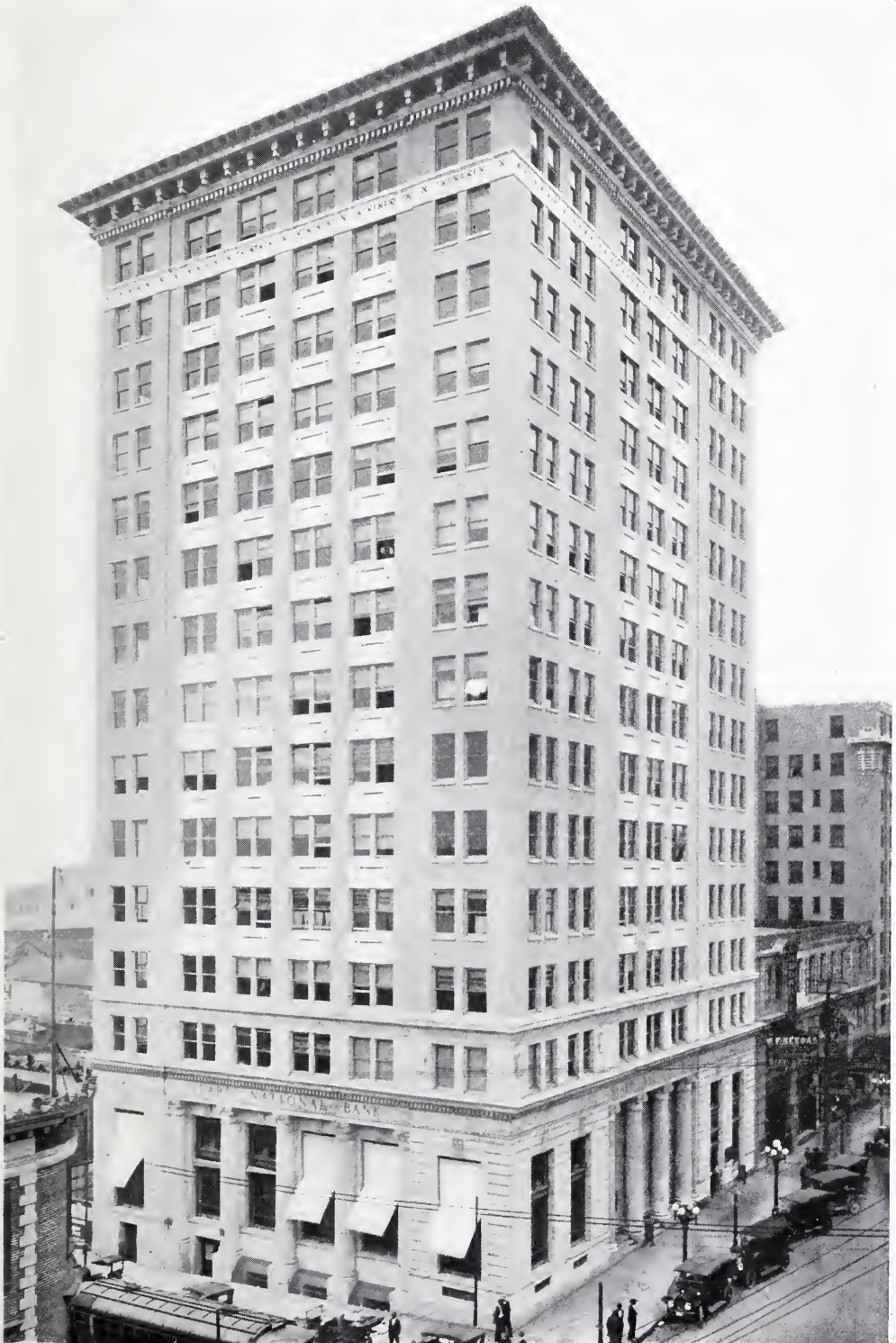
HEARD NATIONAL BANK BUILDING, JACKSONVILLE, FLA. JOHN KEVAN PEBBLES, ARCHITECT.
