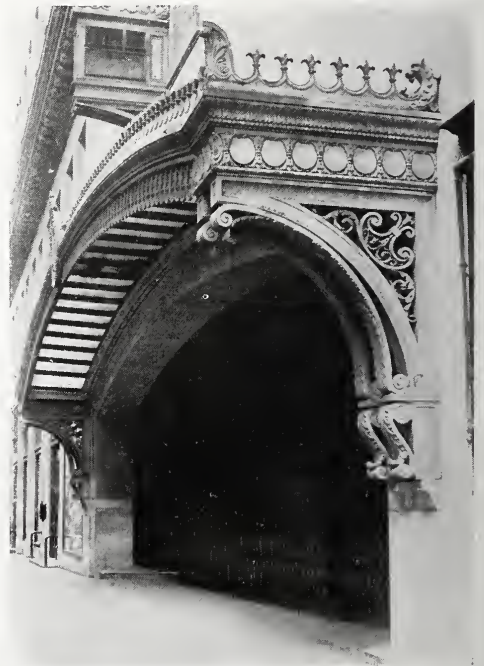
MARQUEE OF LORD & TAYLOR'S STORE, NEW YORK. Starrett & Van Vleck, Architects.
