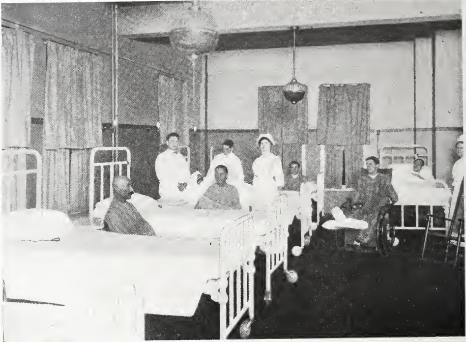
FIG. 27. MALE WARD, OHIO VALLEY GENERAL HOSPITAL, WHEELING, W. VA. Edward F. Stevens, Architect.
