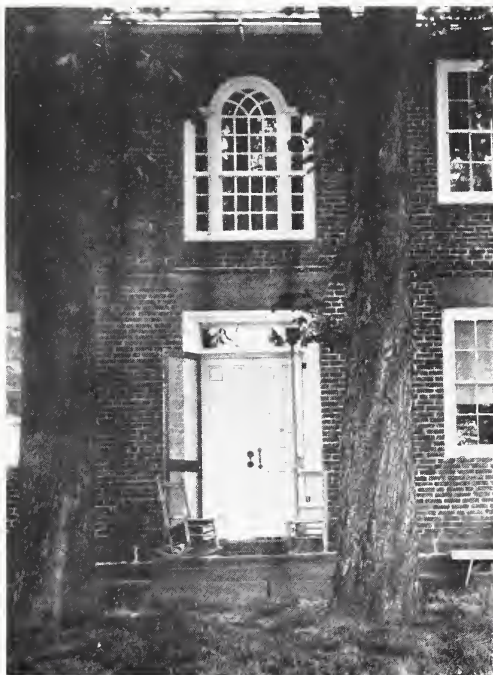
DOORWAY OF THE DUKE OF CUMBERLAND INN., ROCKY HILL, CONN. BUILT OF FIRST BRICK MADE IN AMERICA.
