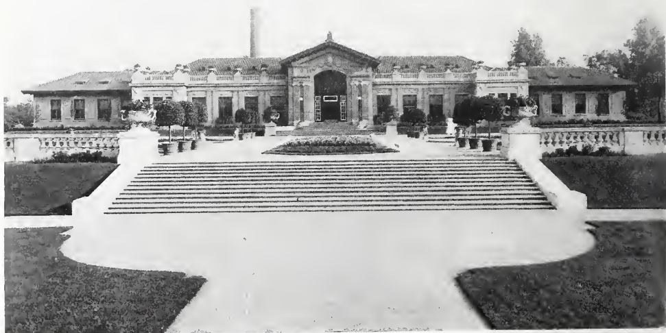
ADMINISTRATION BUILDING AND FORMAL GARDENS, WASHINGTON PARK, CHICAGO, 1910, 1912. D. H. Burnham & Co., Architects.
