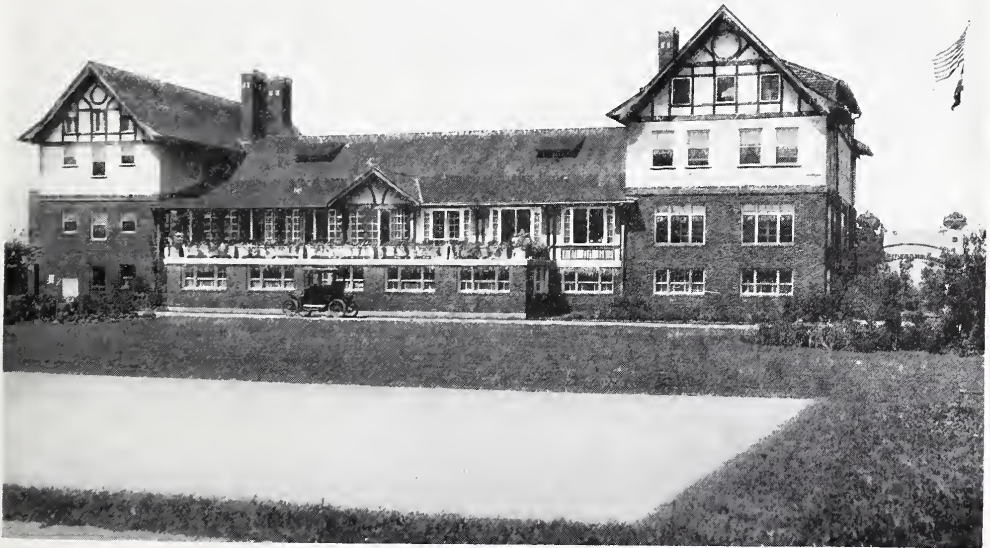
SOUTH FRONT—EDGEWATER GOLF CLUB, CHICAGO. Hill & Woltersdorf, Architects.
