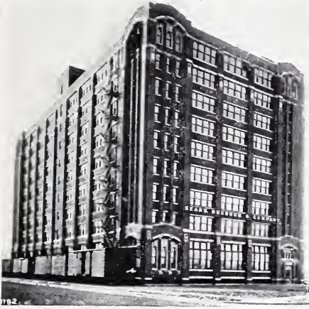
Completed First Unit.
