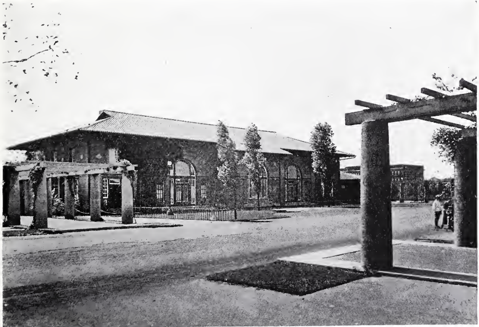
SHERMAN PARK BUILDING, CHICAGO. D. H. Burnham & Co., Architects.
