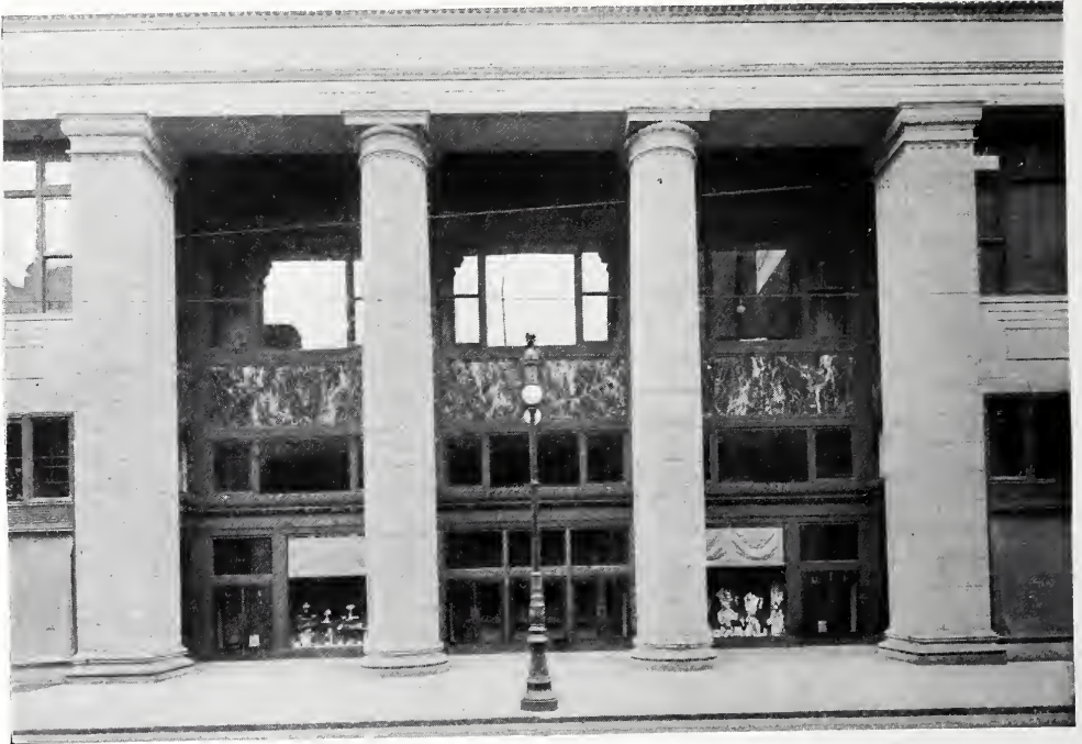
CHESTNUT STREET ENTRANCE—THE WANAMAKER STORE, PHILADELPHIA. D. H. Burnham & Co., Architects.
