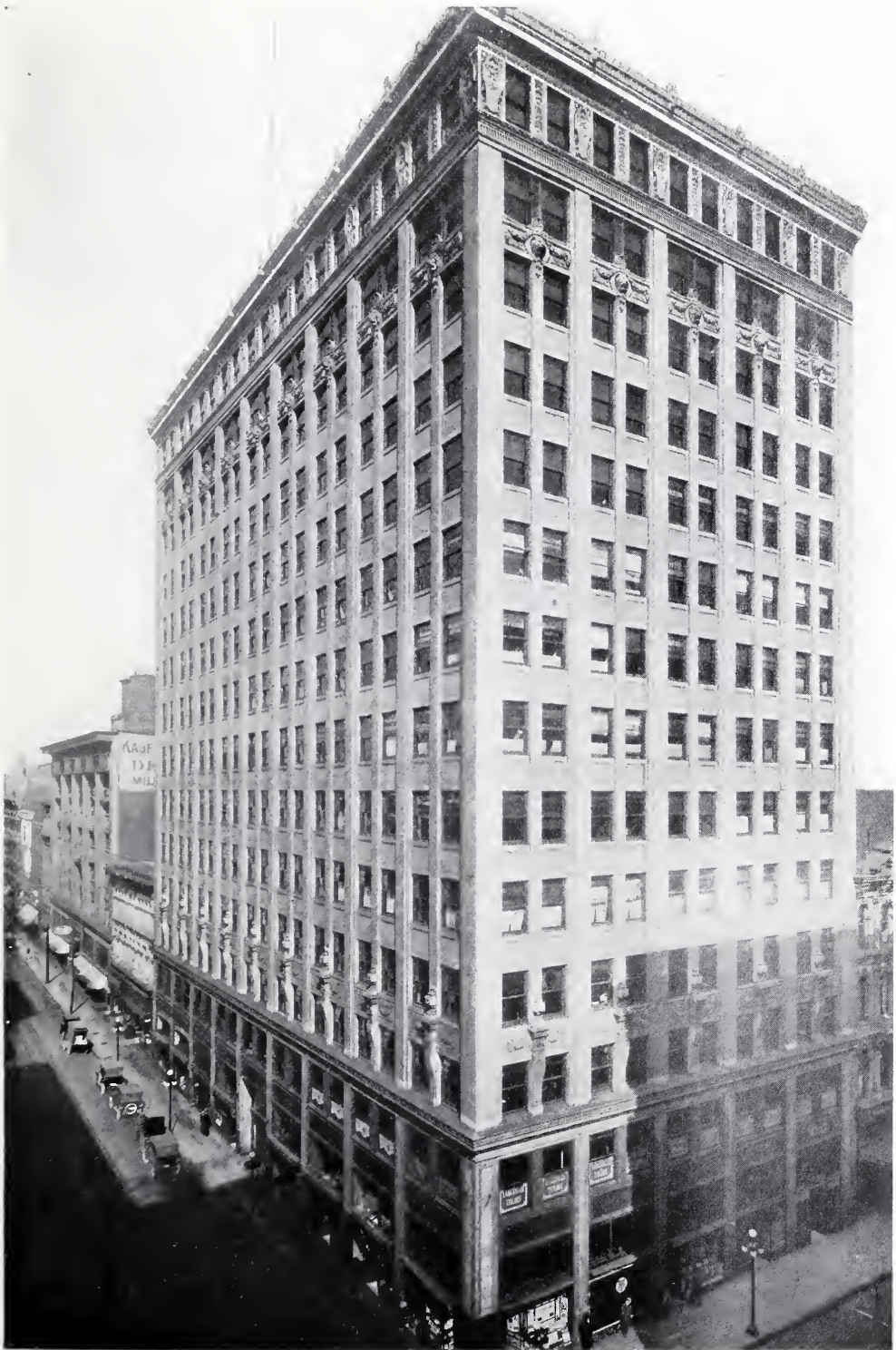
STARKS BUILDING, LOUISVILLE, KY., 1913. D. H. BURNHAM & CO., AND GRAHAM, BURNHAM & CO., ARCHITECTS.
