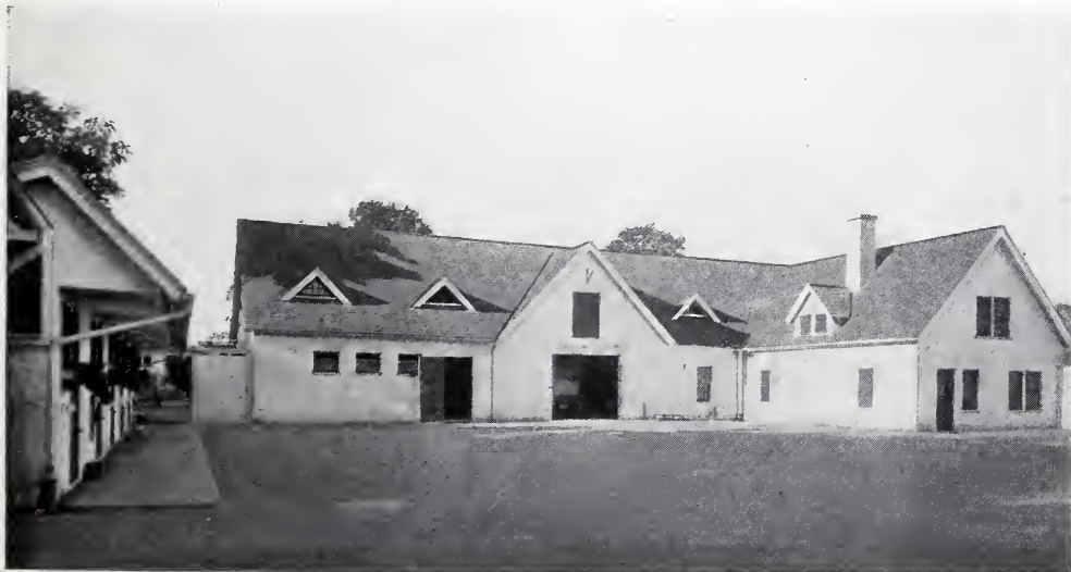
STABLES—HOUSE OF ARTHUR A. FOWLER, ESQ., PEAPACK, N. J. Hewitt & Bottomley, Architects.
