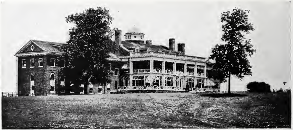
SOUTHWEST FRONT—BELLE REVE COUNTRY CLUB, ST. LOUIS. E. G. Garden, Architect.
