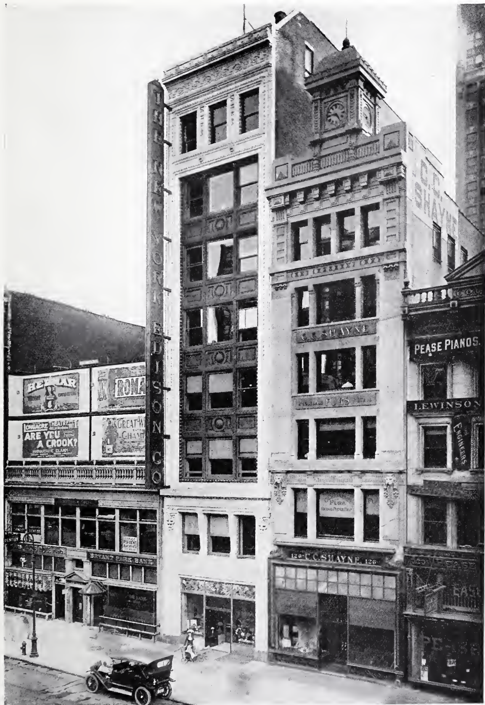
EDISON BUILDING, NEW YORK, 1912. D. H. BURNHAM & CO., ARCHITECTS.
