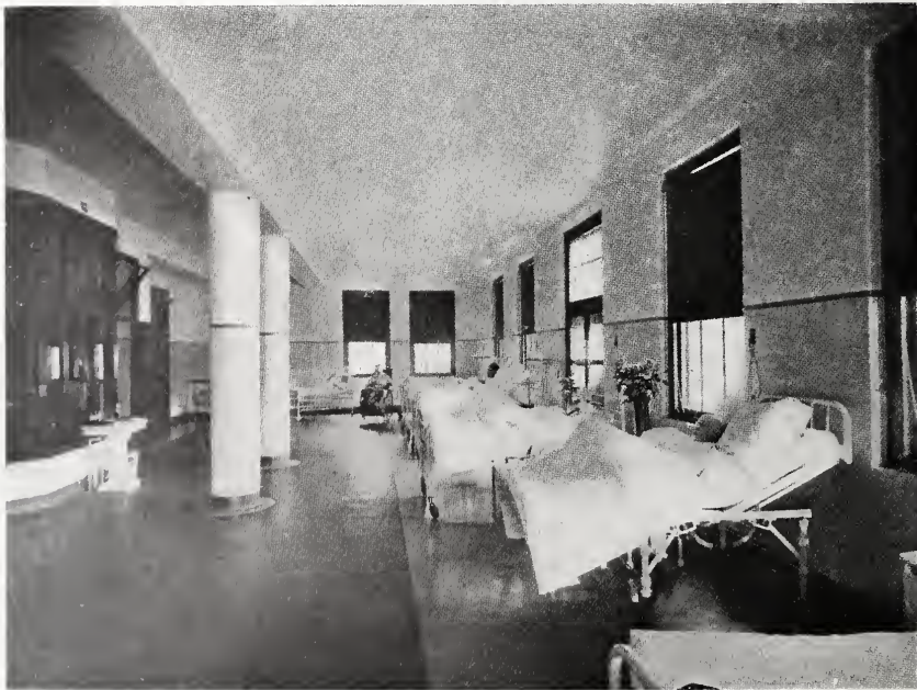
FIG. 20. INTERIOR OF WARD, PAVILION "C," PETER BENT BRIGHAM HOSPITAL, BOSTON, MASS. Codman & Despradelle, Architects.
