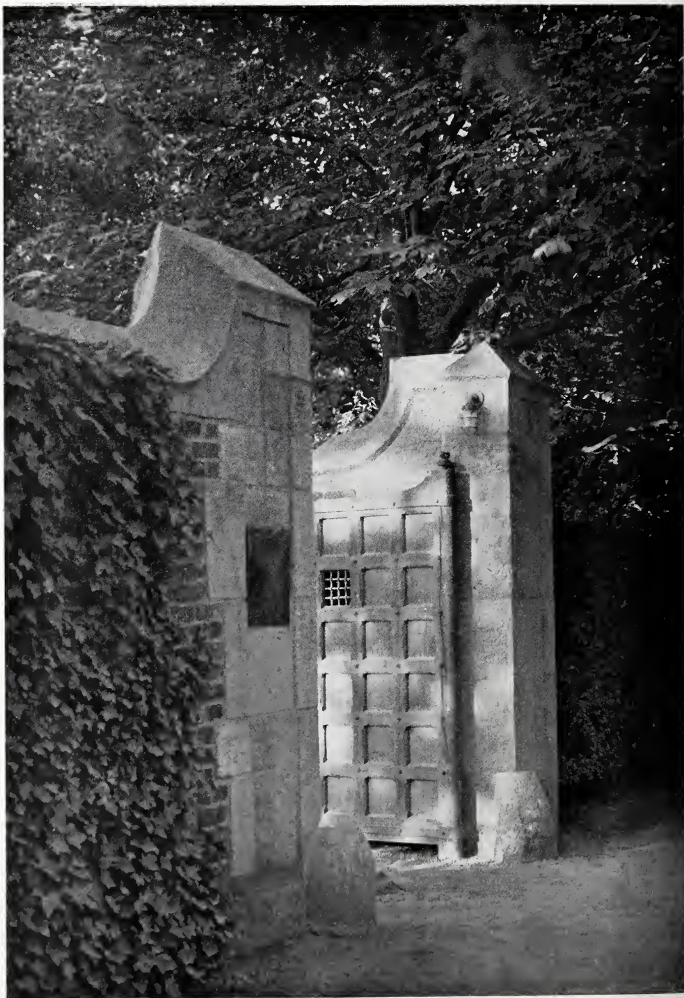
SERVICE GATE—RESIDENCE OF STUART DUNCAN, ESQ., NEWPORT, R. I. JOHN RUSSELL POPE, ARCHITECT.
