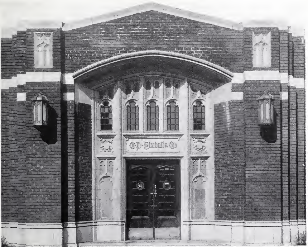
MAIN ENTRANCE—BUILDING OF C. P. KIMBALL & CO., CHICAGO. George C. Nimmons, Architect.
