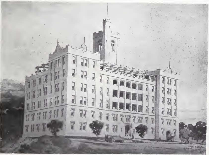
FIG. 22. GENERAL VIEW, OHIO VALLEY GENERAL HOSPITAL, WHEELING, WEST VIRGINIA. Edward F. Stevens, Architect.
