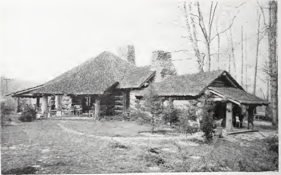
LOG CABIN—ESTATE OF CHARLES S. WALTON, ESQ., ST. DAVIDS, PA. D. Knickerbacker Boyd, Architect.
