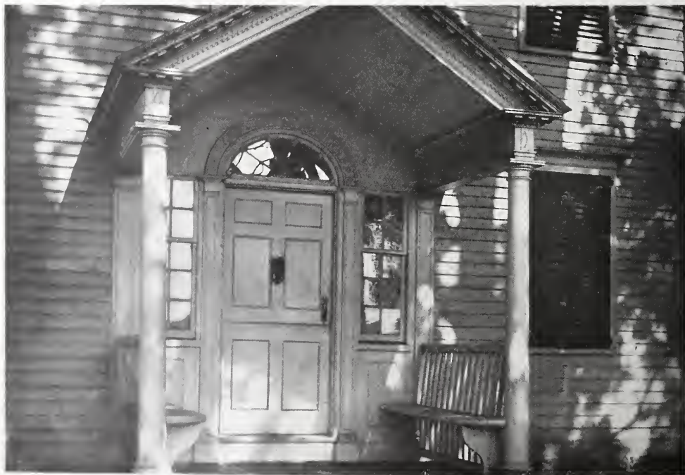
DOORWAY OF THE STILES HOUSE, SOUTHBURY, CONN.
