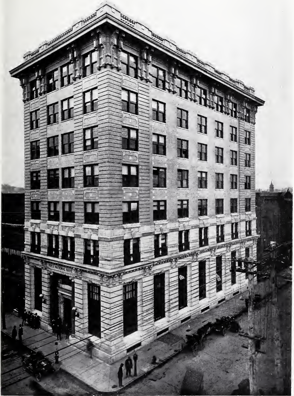
FIRST NATIONAL BANK, ROANOKE, VA. JOHN KEVAN PEBBLES, ARCHITECT.
