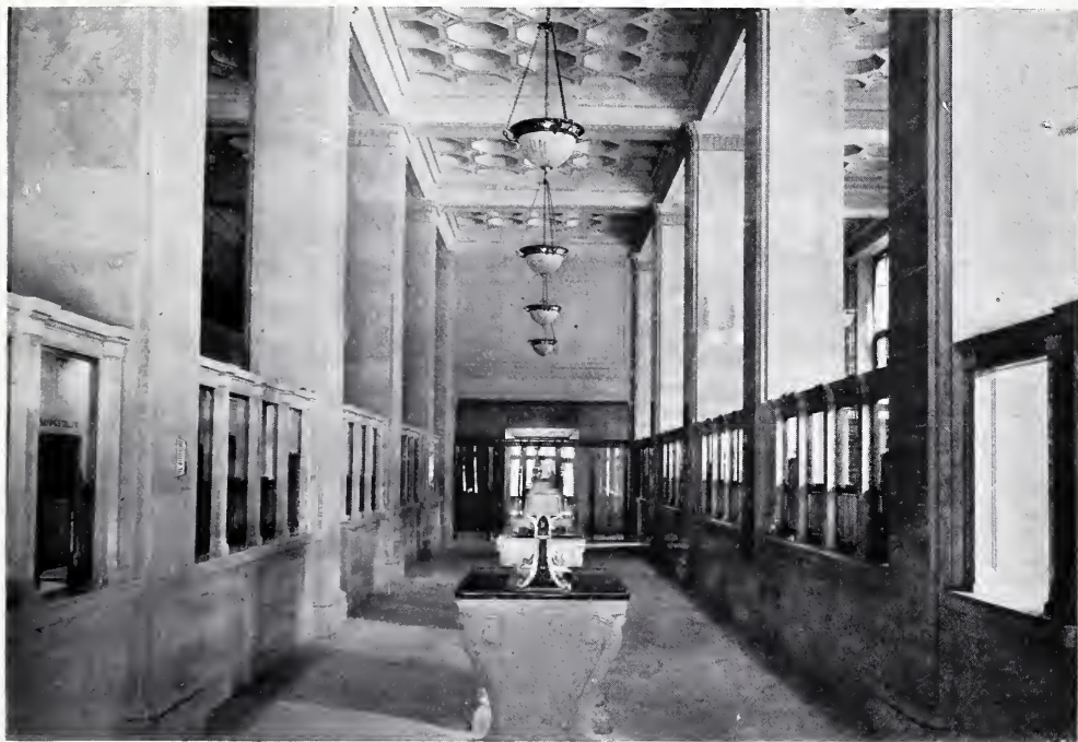
BANKING ROOM—MINERS' BANK, WILKESBARRE, PA. D. H. Burnham & Co. and Graham, Burnham & Co., Architects.
