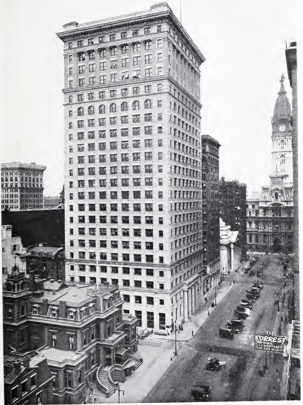
LAND TITLE BUILDING, PHILADELPHIA, 1897, 1904. D. H. BURNHAM & CO., ARCHITECTS.
