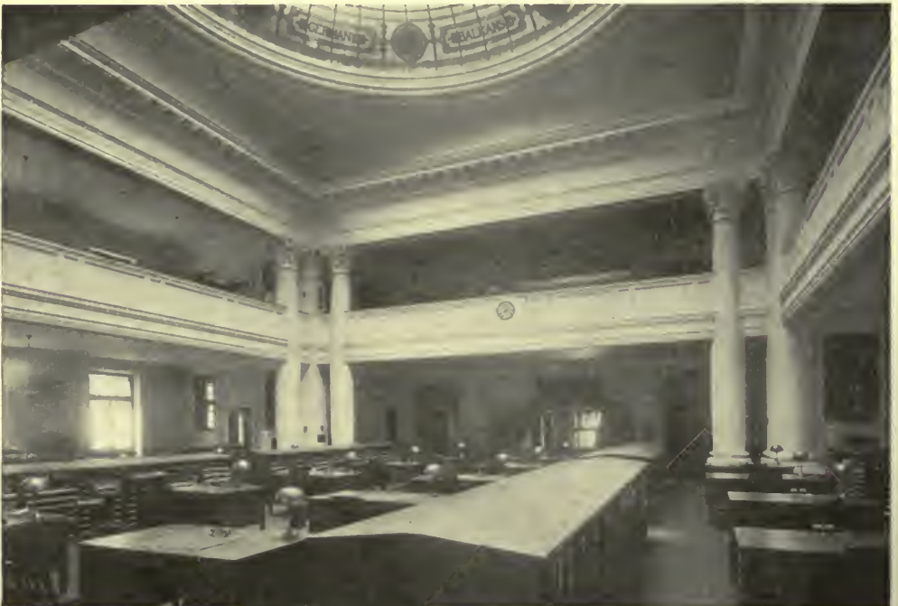
MAIN ROOM—ROSSIA INSURANCE COMPANY'S BUILDING, HARTFORD, CONN. Edward T. Hapgood, Architect.
