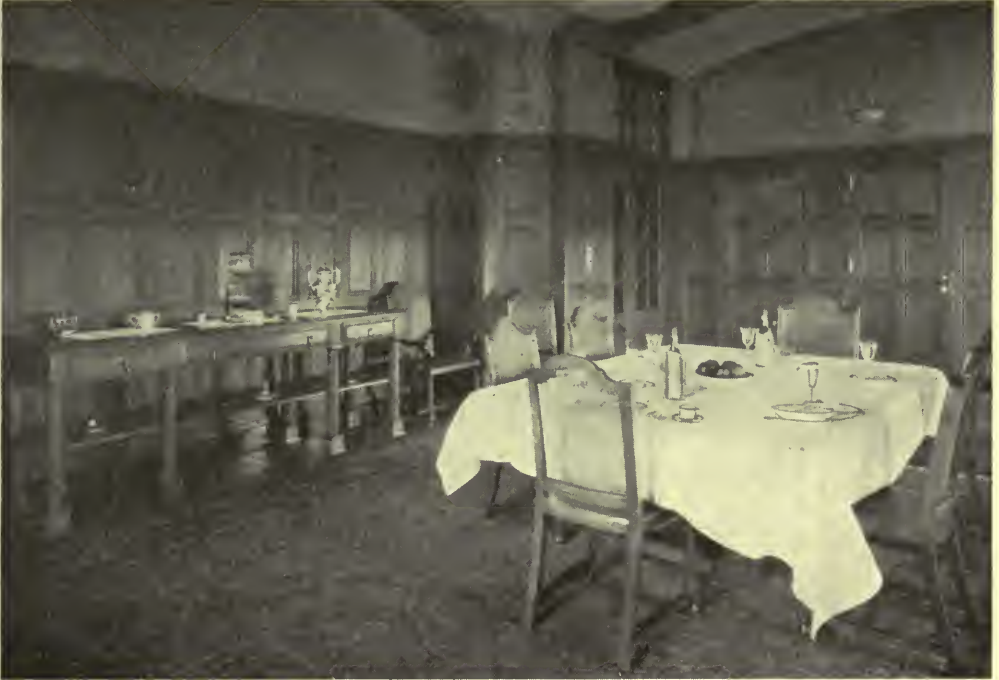
FIRST OFFICERS' DINING ROOM—PENN MUTUAL BUILDING, PHILADELPHIA. Edgar V. Seeler, Architect.
