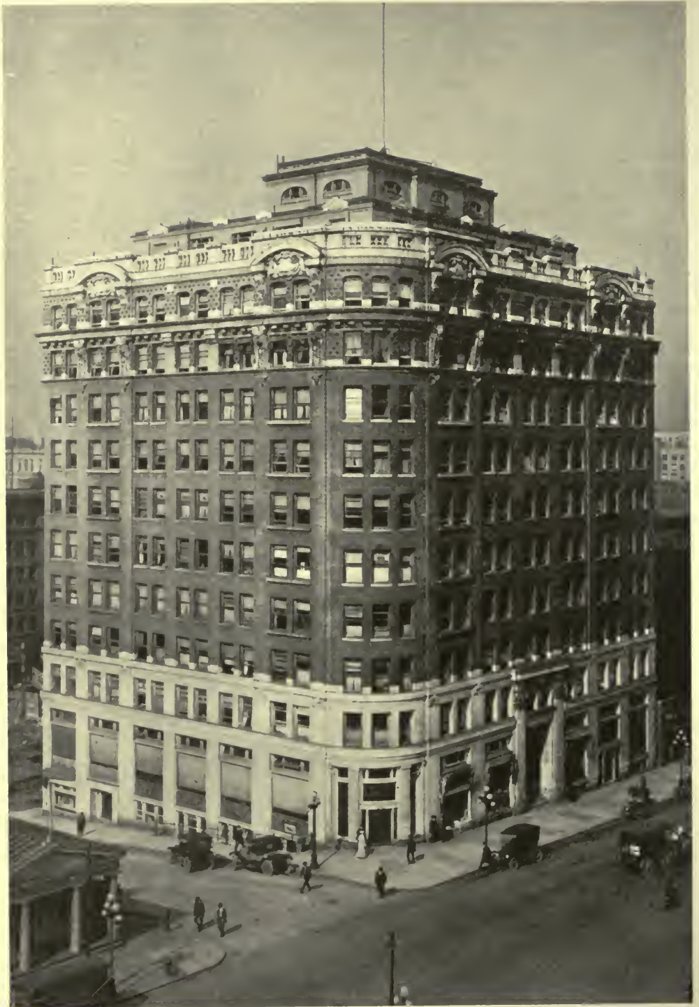
COBB BUILDING, SEATTLE, WASH. HOWELLS & STOKES, ARCHITECTS.
