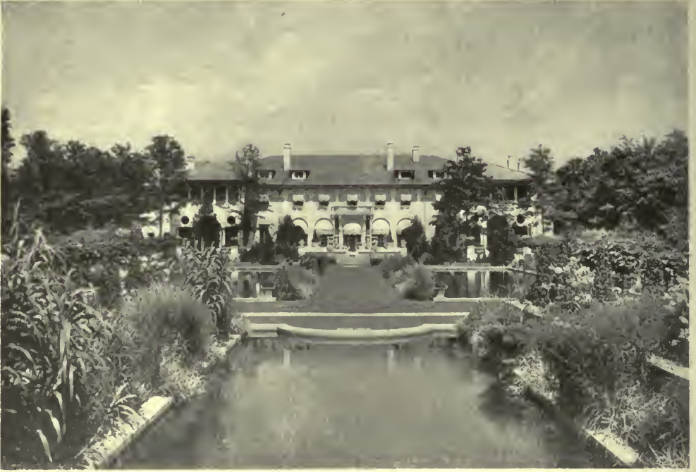
FIG. 17. WEST FRONT, FROM THE CASINO ACROSS THE WATER GARDEN—MELODY FARM, LAKE FOREST, ILL.
