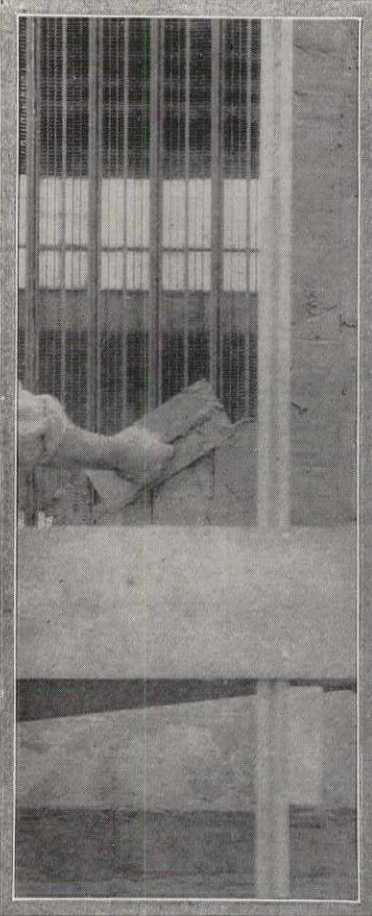
Applying scratch coat. In this exterior wall no studding was used. Ribplex, back-plastered, made a smooth wall inside and out.
