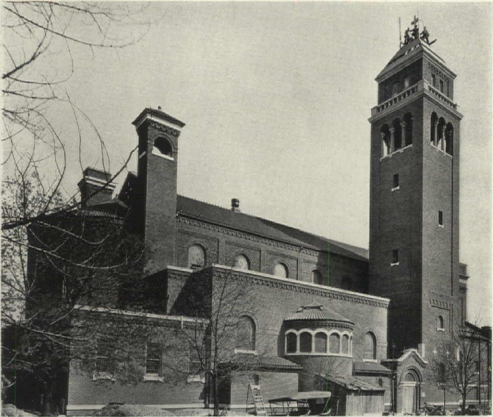
DETAIL OF WEST AISLE—HOLY ROSARY CHURCH, DAYTON, OHIO. W. L. Jaekle, Architect.
