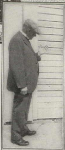
This man has just rubbed his hand over the boards of a house painted with pure white lead and oil. His fingers are all white from the chalking off of the paint. The paint was pure. But the paint is poor. Lowe's paint does not chalk off.
