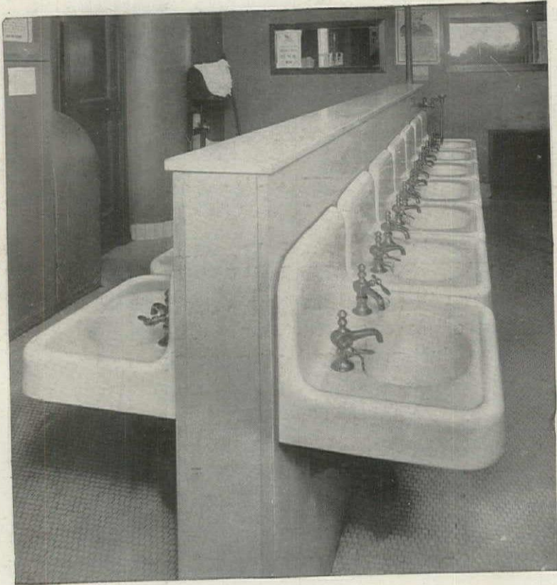
Wolff Lavatories in Reid, Murdock & Co. Building, Chicago. George C. Nimmons, Architect C. J. Stein, Plumbing Contractor
