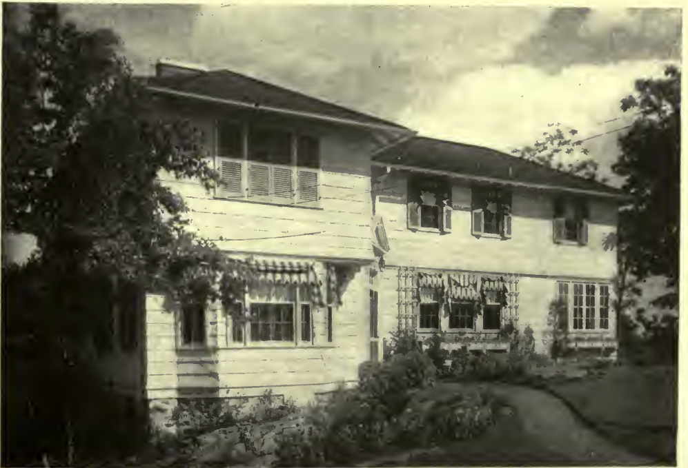
RESIDENCE OF FRED LAVIS, ESQ., HARTSDALE, N. Y. Parker Morse Hooper, Architect.
