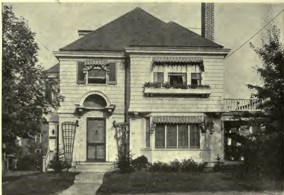
RESIDENCE OF DR. EDMUND F. CURRY, FALL RIVER, MASS. Parker Morse Hooper, Architect.
