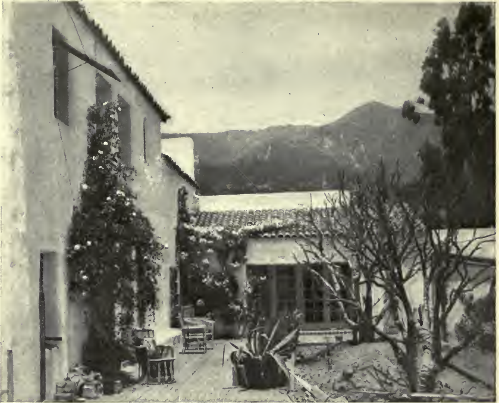
GARDEN FAÇADE, LOOKING TOWARD DINING ROOM—"CASA DRACAENA," RESIDENCE AT SANTA BARBARA, CAL., OF GEORGE WASHINGTON SMITH, ARCHITECT.
