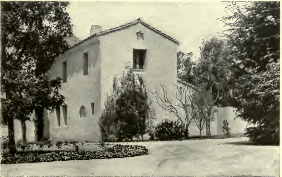
RESIDENCE OF WILLARD P. LINDLEY, ESQ., SANTA BARBARA, CAL. George Washington Smith, Architect.
