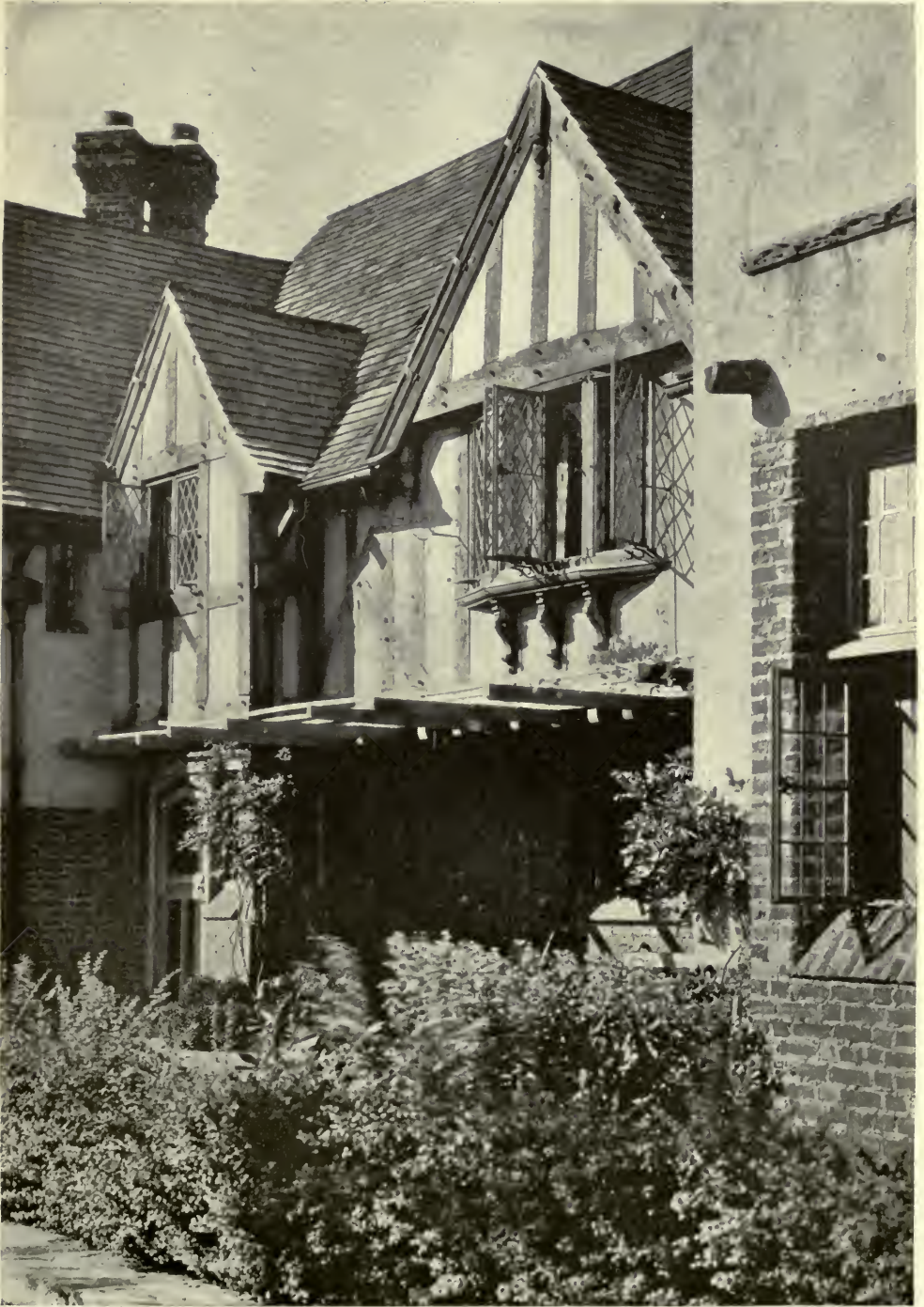
SOUTH ENTRANCE—RESIDENCE OF CAS- PAR W. MORRIS, ESQ., HAVERFORD, PA. MELLOR, MEIGS & HOWE, ARCHITECTS.
