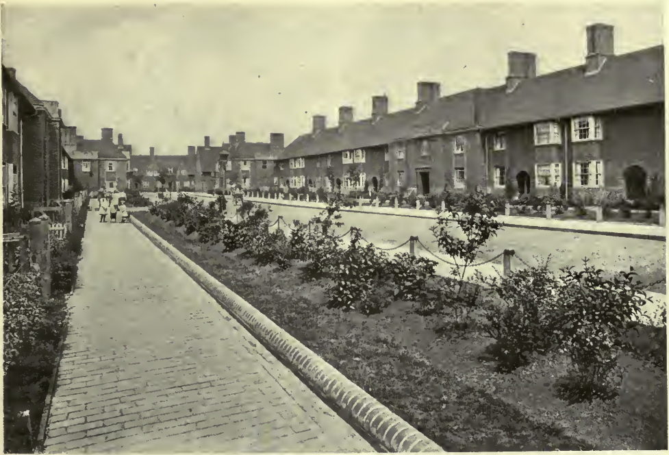
LONDON COUNTY COUNCIL COTTAGES AT HAMMERSMITH. Row houses that are not monotonous.
