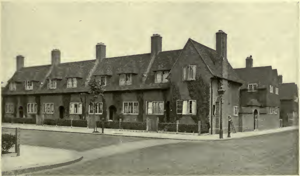
LONDON COUNTY COUNCIL COTTAGES AT HAMMERSMITH. Containing five rooms and bath. In 1911 each house cost £300, as against £1,125 today.
