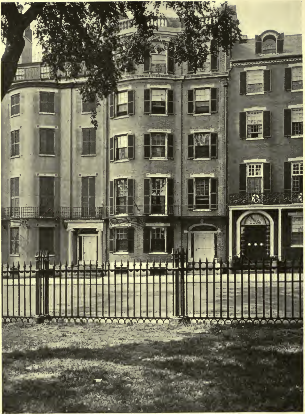
FIG. 25. APARTMENT HOUSE AT 62 BEACON ST., BOSTON. RICHARD ARNOLD FISHER, ARCHITECT.
