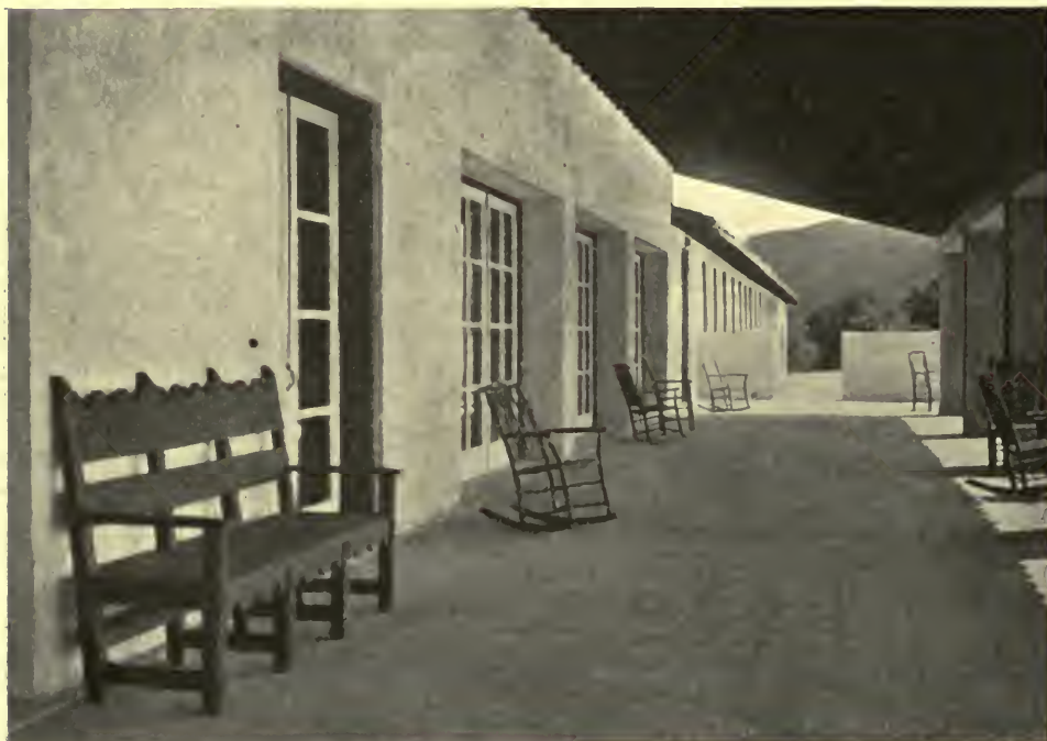
LOOKING SOUTH ON PORCH—FLINTRIDGE COUNTRY CLUB, FLINTRIDGE, NEAR PASADENA, CAL. Myron Hunt, Architect
