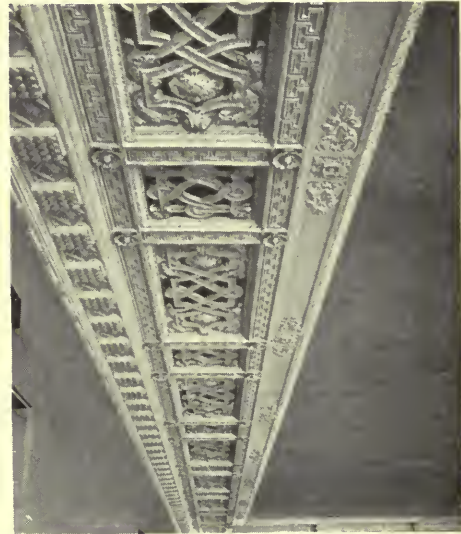
DETAIL OF SIDE OF CEILING
