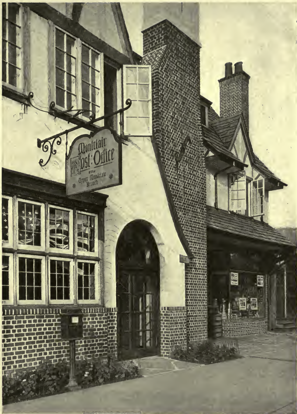
DETAIL OF POST OFFICE, UPPER MONTCLAIR, N. J. FRANCIS A. NELSON, ARCHITECT.
