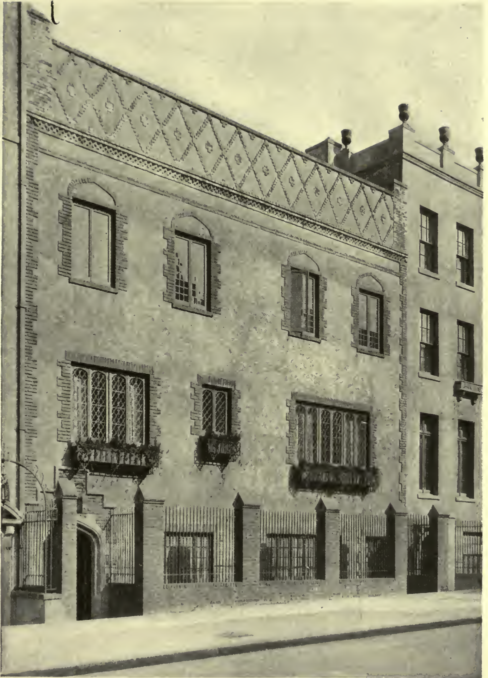
HOUSE ON EAST SIXTY-THIRD STREET, NEW YORK CITY. FREDERICK STERNER, ARCHITECT.
