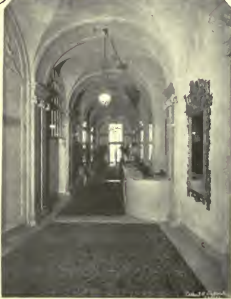
Corridor in the Hotel Ambassador. Note the inlet valve in the baseboard at the right.
