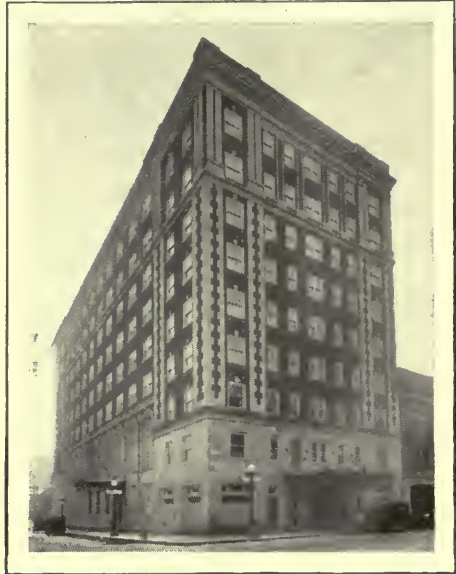
The Fort Steuben Hotel, Steubenville, Ohio: Frederic Webber, Phila., Architect; J. D. Johnson Co., Inc., Phila., Jobbers; Modern Plumbing & Heating Co., Phila., Plumbers
