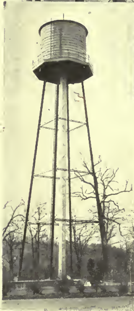
A 30,000 gallon water tank of 3" Redwood. Installed at the Pittsburgh Field Club for club house water system, watering the greens and supplying water for swimming pool.
