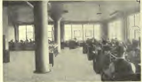
Parker Pen Co., Janesville, Wis., Frank Carpenter, Arch.
