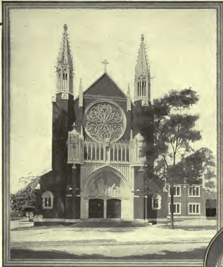
Grace Evangelical Lutheran Church, Wadsworth, Ohio. Mr. Reynold H. Hinsdale, Cleveland, Architect; Artstone furnished by The George Rackle & Sons Co., Cleveland, using Medusa Stainless White Cement. Waterproofed.
