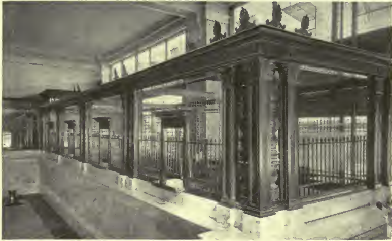
AMBRAC EXTRUDED BRONZE COUNTERSCREEN OF THE BANK OF COMMERCE, SPRINGFIELD, MO. Opel & Torbett, Architects. Fabricated by the Michaels Art Bronze Company, Cincinnati, Ohio, from AMBRAC extruded bronze shapes and mouldings manufactured by The American Brass Company.
