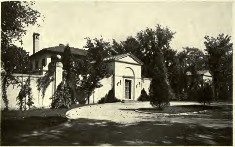
RESIDENCE OF CHARLES B. PIKE, ESQ., LAKE FOREST, ILL. David Adler and Robert Work, Architects.
