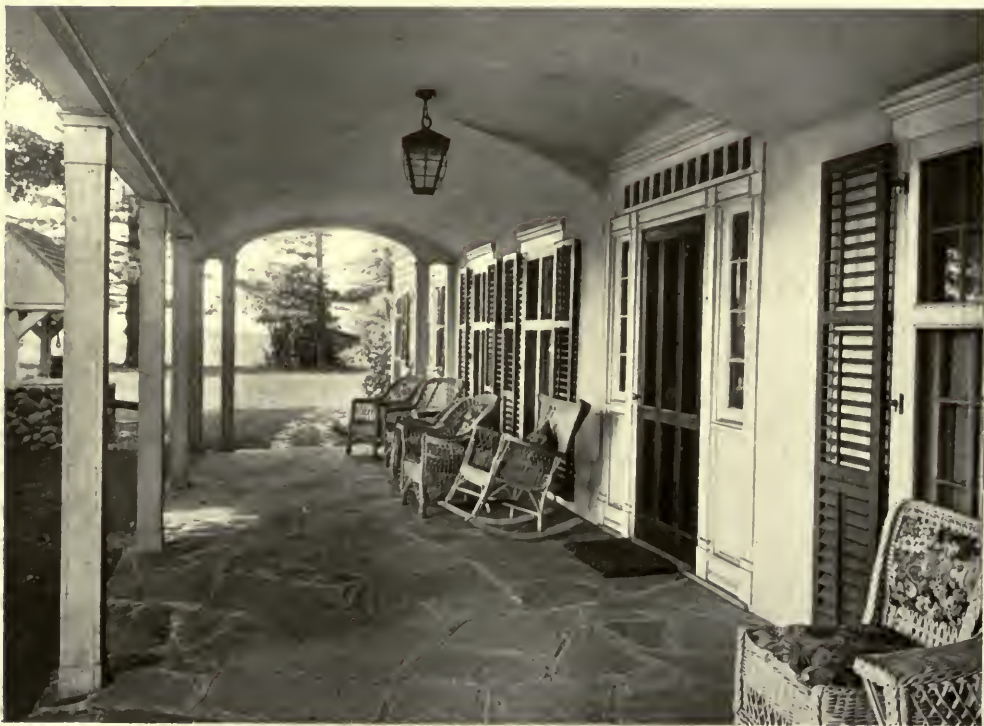
PORCH—RESIDENCE OF HERBERT E. GUNNISON, ESQ., PURCHASE, N. Y. Wesley Sherwood Bessell, Architect.
