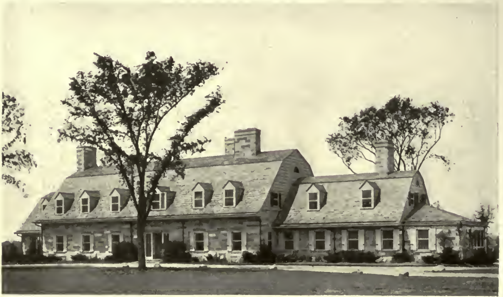
RESIDENCE OF MALCOLM McKAY, ESQ., TENAFLY, N. J. Frank J. Forster, Architect.
