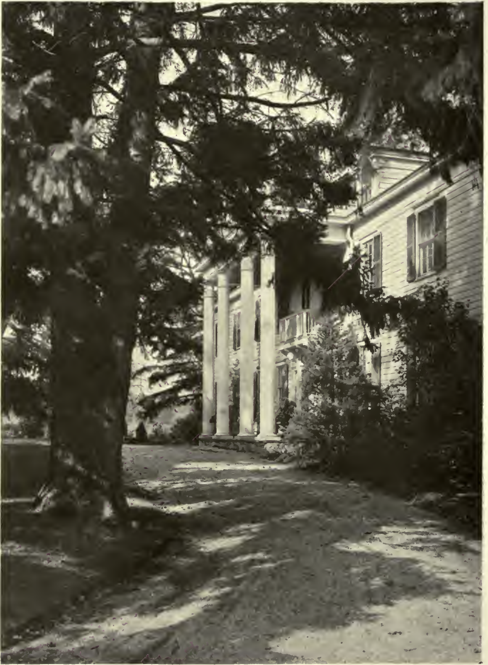
RESIDENCE OF WINCHESTER FITCH, ESQ., GREENWICH, CONN. GODLEY AND SEDGWICK, ARCHITECTS.
