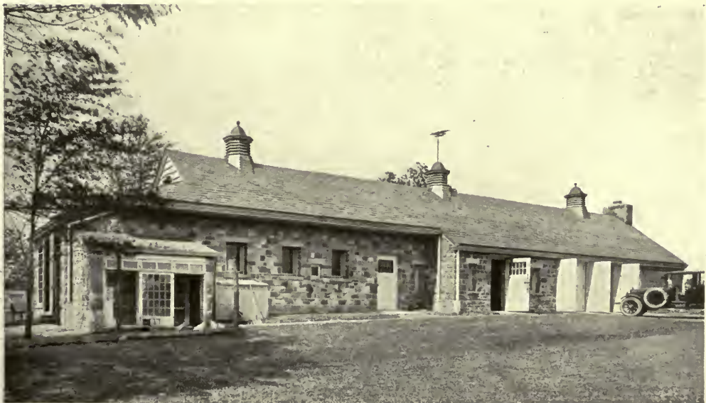
GARAGE FOR MALCOLM McKAY, ESQ., TENAFLY, N. J. Frank J. Forster, Architect.
