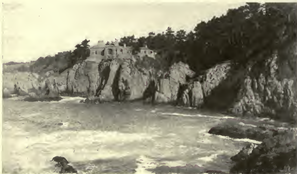
RESIDENCE OF D. L. JAMES, ESQ., CARMEL HIGHLANDS, CAL. Charles Sumner Greene, Architect.
