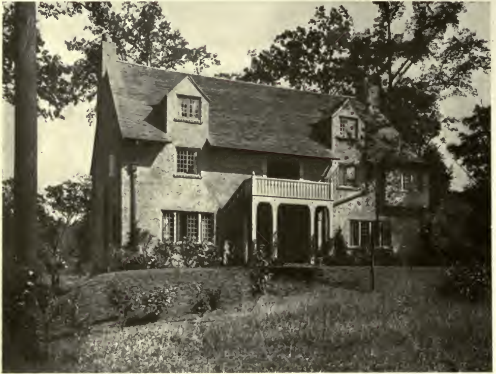
RESIDENCE OF MRS. MARY McKELVEY, SPUYTEN DUYVIL, NEW YORK CITY. Julius Gregory, Architect.
