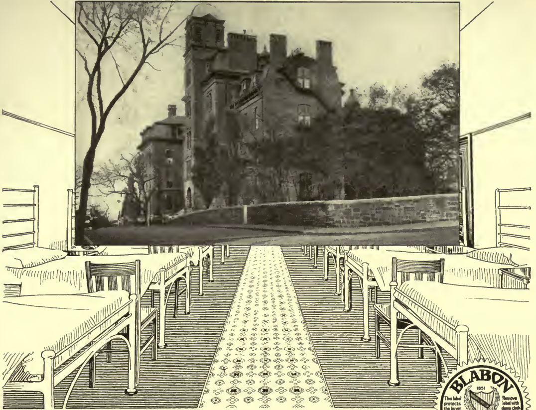
Blabon floors of linoleum in the Carney Hospital, Boston, Mass., are a sanitary aid and a promoter of quietness.
