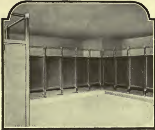
Sanymetal in St. Joseph's School, Cleveland. Chas. R. Greco, Arch.
