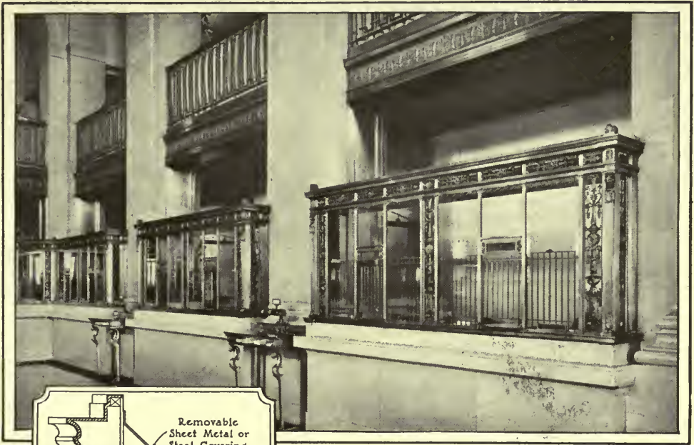
Counter Screen of the Astor Trust Company, New York. Charles E. Birge, Architect. Fabricated by the Gorham Company from Anaconda extruded architectural bronze.
