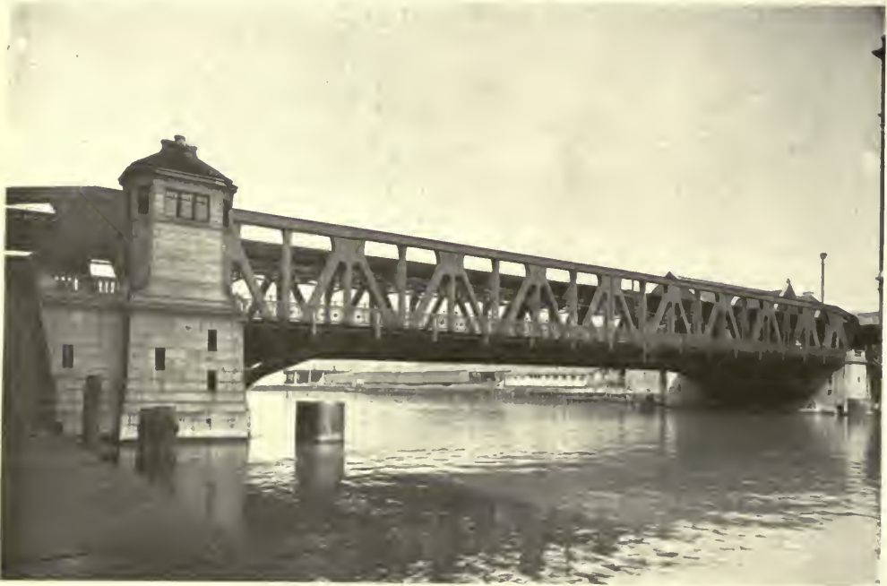
WELLS STREET DOUBLE DECK BRIDGE, CHICAGO, ILLINOIS.
