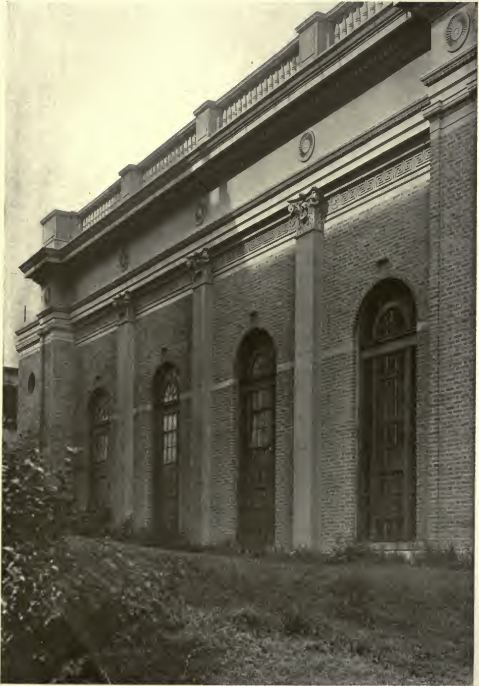
SIDE DETAIL—SECOND CHURCH OF CHRIST SCIENTIST, BAY RIDGE, NEW YORK CITY. BERNHARDT E. MULLER, ARCHITECT.
