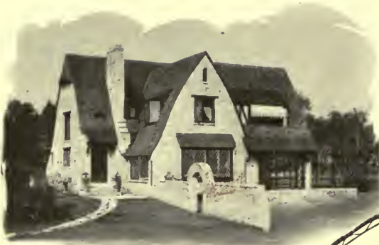
Residence of S. S. Bemman, Winnetka, Ill. Celotex used for insulation on all walls and roof under exterior finish.
