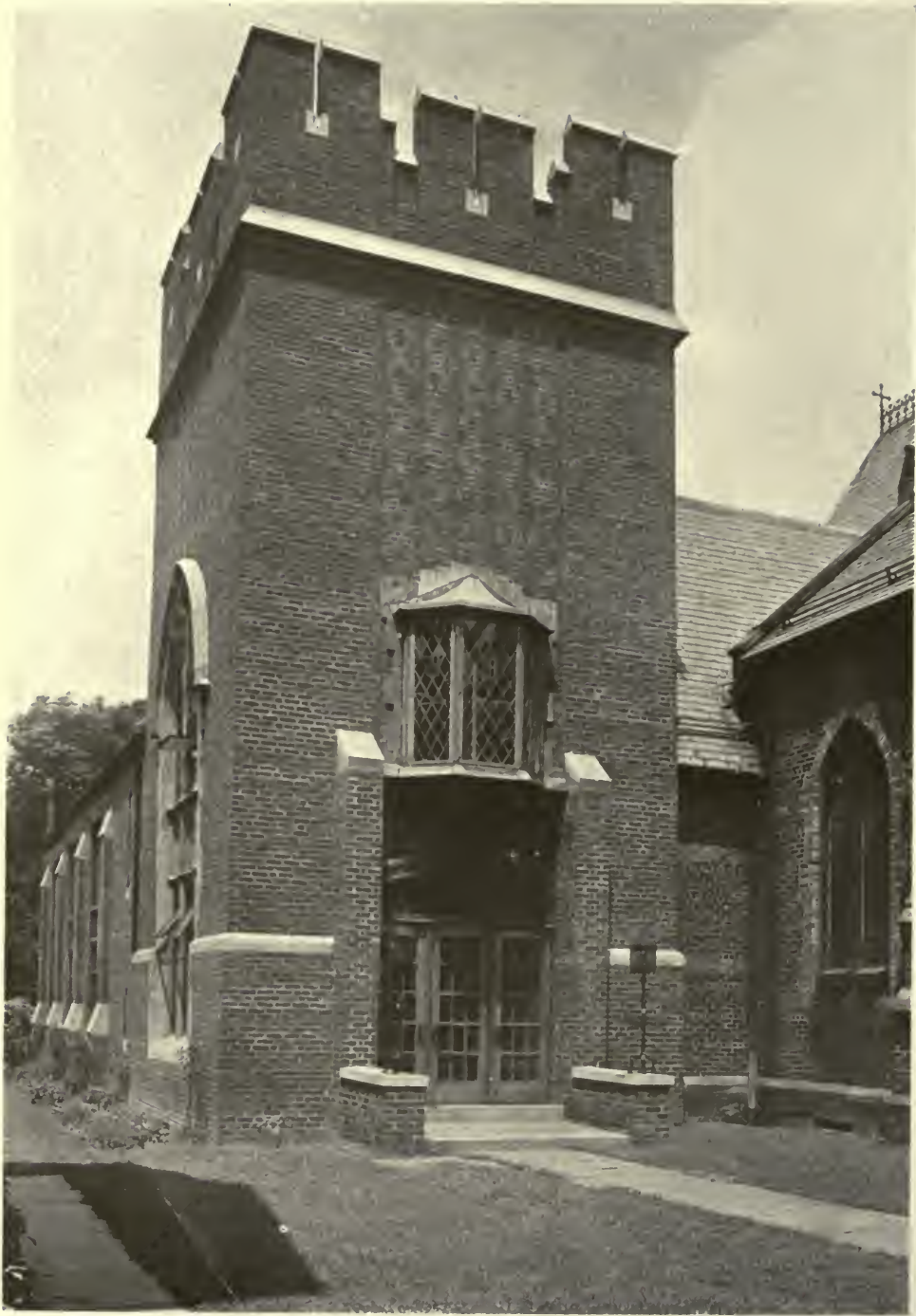
TOWER—CHRIST CHURCH PARISH HOUSE, HACKENSACK, N. J. WESLEY SHERWOOD BESSELL, ARCHITECT.
