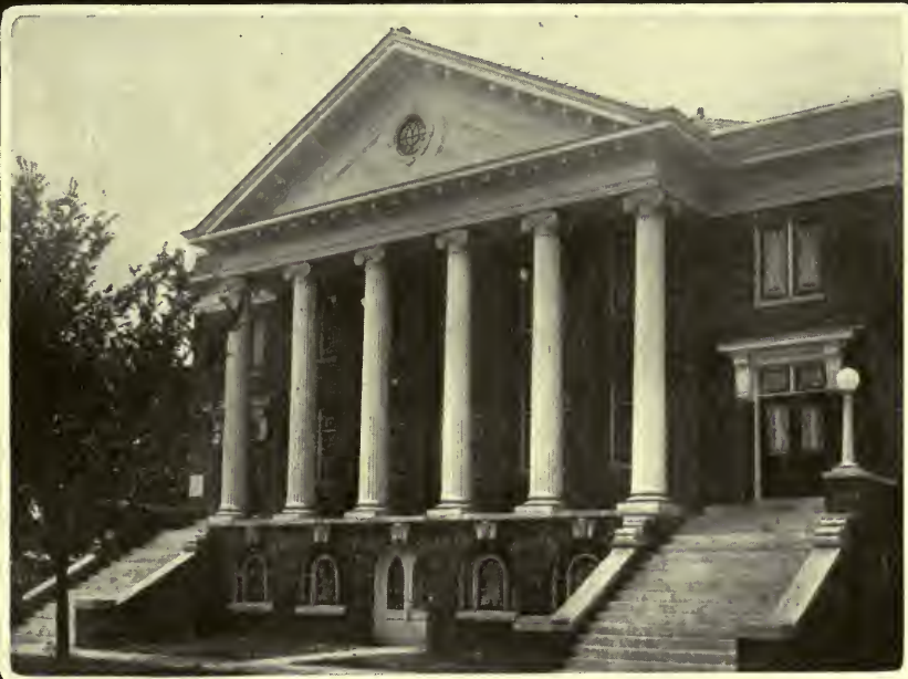
Fairfield Baptist Church, Fairfield, Ala. J. E. Greene, Architect, Birmingham, Ala. 6 Union Metal Greek Ionic Columns, 28" Diameter, 21' high.
