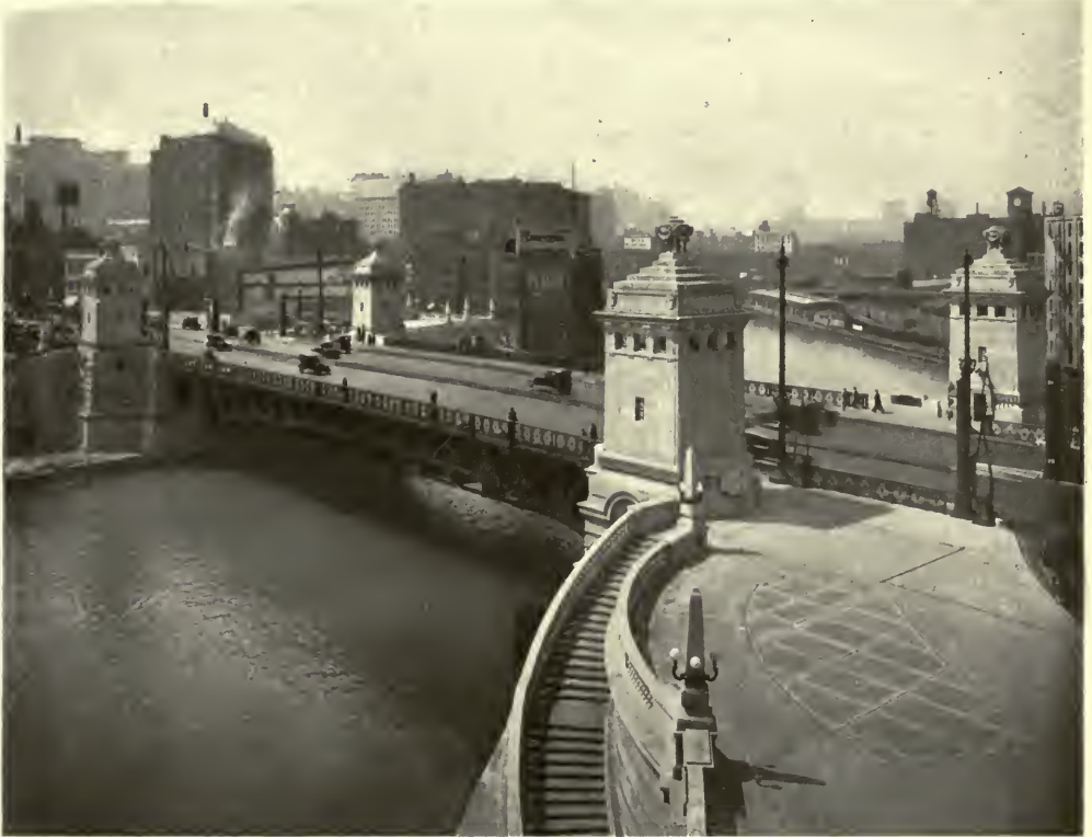
MICHIGAN AVENUE DOUBLE DECK BRIDGE AND APPROACHES.
