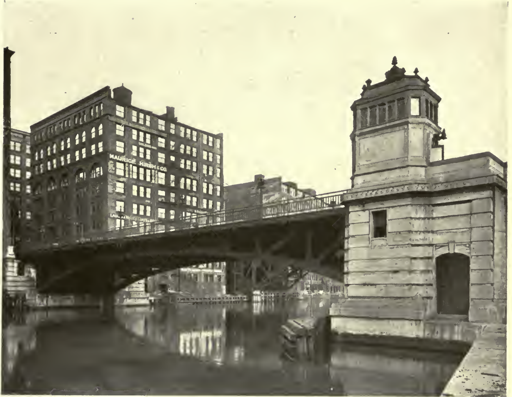
JACKSON BOULEVARD BRIDGE OVER THE CHICAGO RIVER, CHICAGO, ILL.
