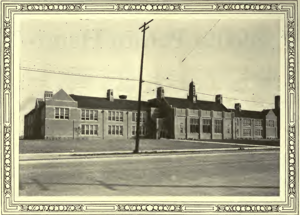
Southwestern High School, Fort Street, Detroit, Michigan Architects, Malcomson, Higginbotham and Palmer, Detroit
