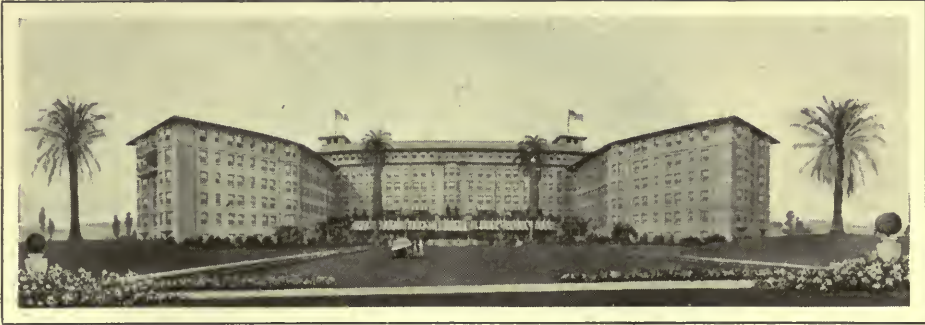
The HOTEL AMBASSADOR, Los Angeles: Myron Hunt, Architect; N. O. Nelson, Mfg. Co., Jobber; Arthur Hess, Plumber
