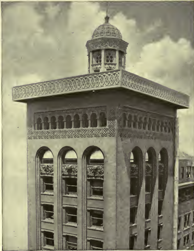
Garrick Theatre (formerly Schiller Theatre) Building, Chicago, Illinois. Adler & Sullivan, Architects. Gray unglazed Terra Cotta throughout. Erected 1891. Photograph taken 1922.
