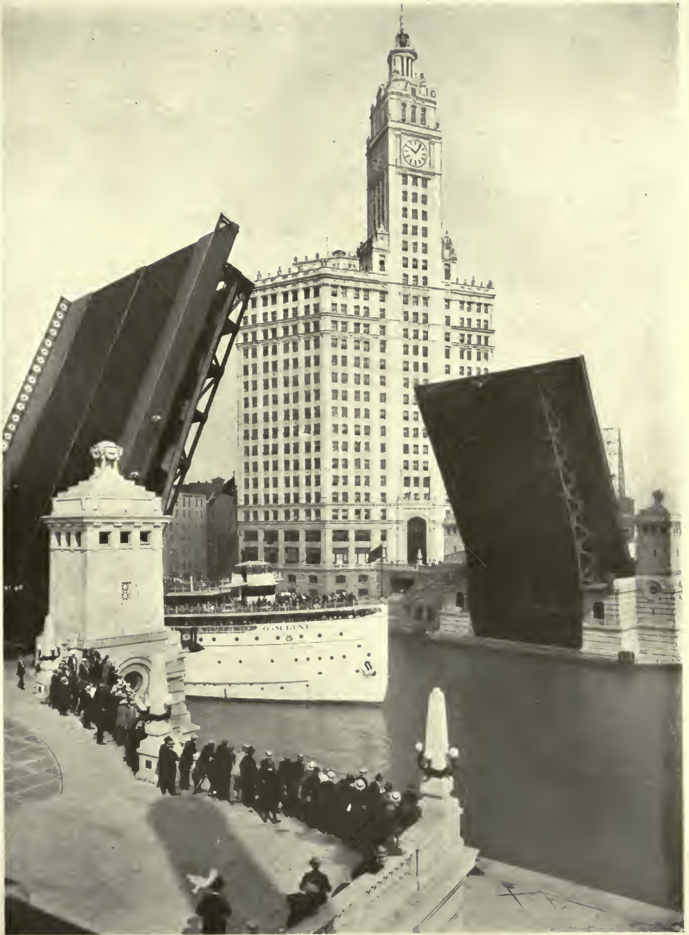
THE MICHIGAN AVENUE BRIDGE SHOWING THE TRUNNION BASCULE TYPE IN OPERATION—IMPROVEMENT OF MICHIGAN AVENUE, CHICAGO, ILLINOIS.
