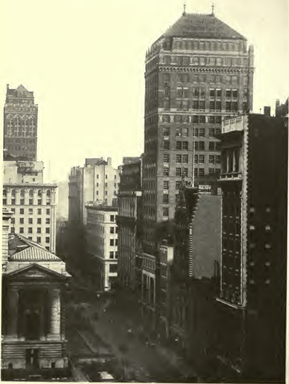
NO 8 WEST FORTIETH STREET, NEW YORK CITY. STARRETT & VAN VLECK, ARCHITECTS.
