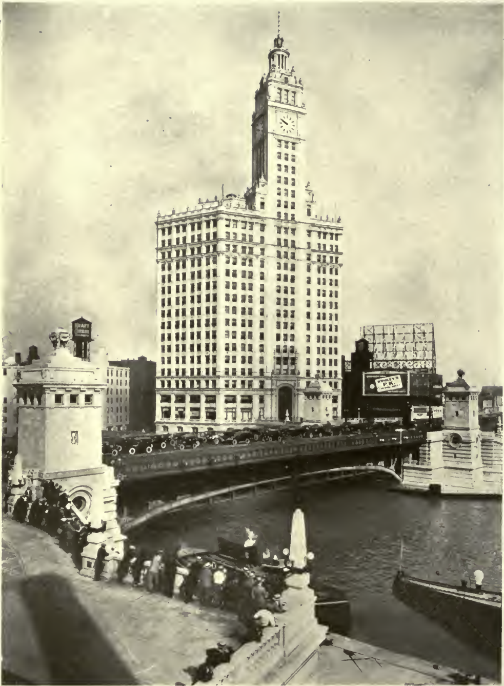
THE MICHIGAN AVENUE BRIDGE—IMPROVEMENT OF MICHIGAN AVENUE AND PINE STREET, CHICAGO, ILLINOIS. The Wrigley Building in the background.
