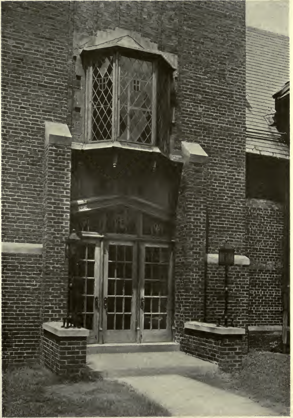
ENTRANCE DETAIL—CHRIST CHURCH PARISH HOUSE, HACKENSACK, N. J. WESLEY SHERWOOD BESSELL, ARCHITECT.
