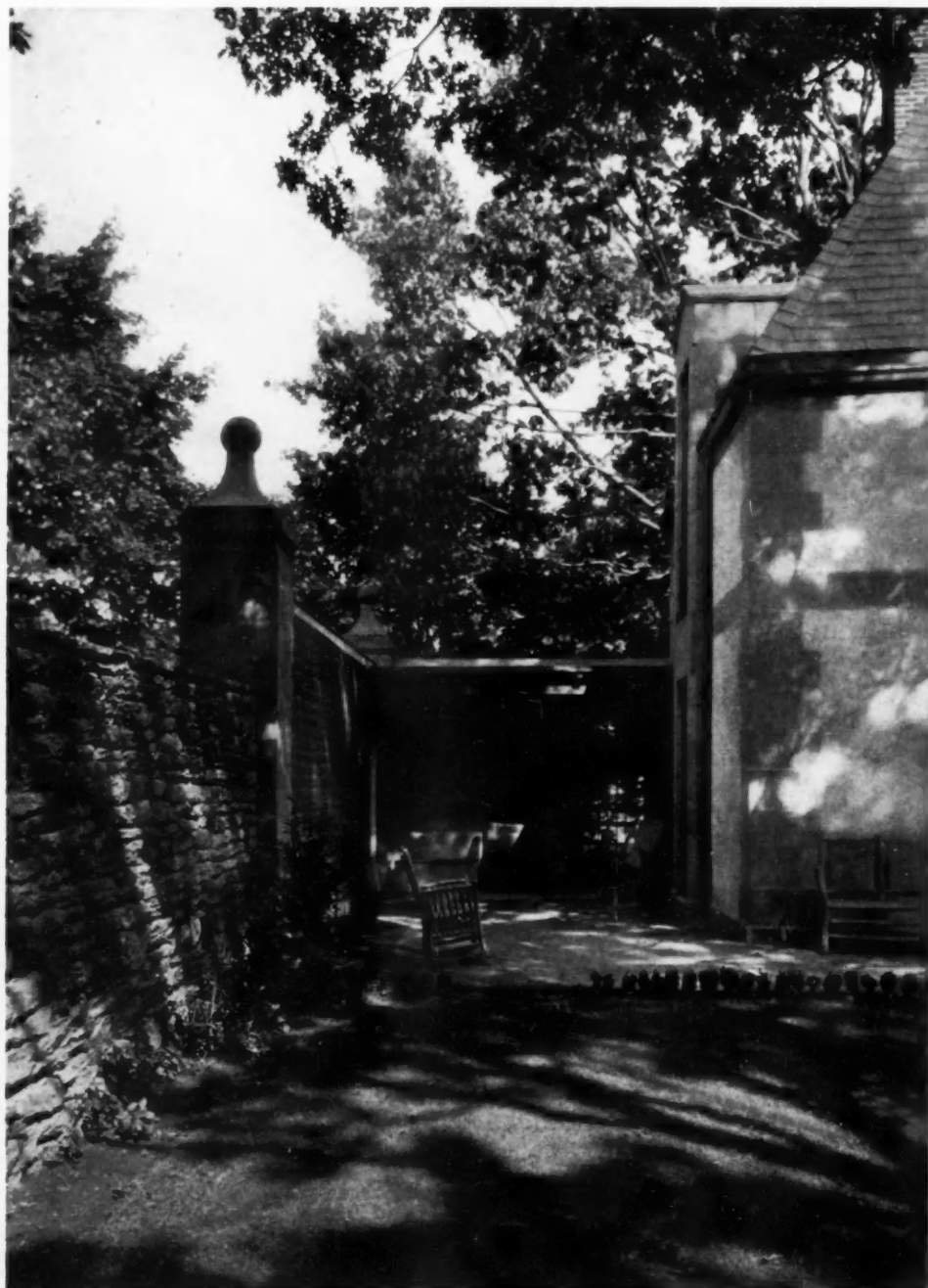
Enclosed Terrace RESIDENCE OF MRS. JOSEPH C. FRALEY, CHESTNUT HILL, PENNSYLVANIA Mellor, Meigs & Howe, Architects [424]
