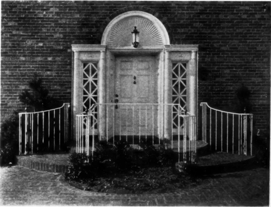
Entrance Detail RESIDENCE OF ROBERT ANDERSON, ESQ., MONTCLAIR, NEW JERSEY Francis A. Nelson, Architect
