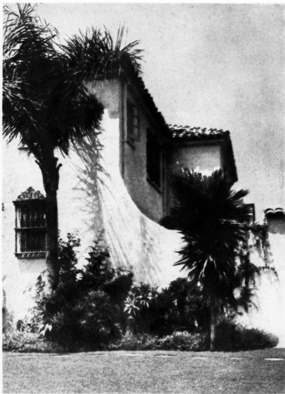
RESIDENCE OF M. H. ADAMSON, ESQ., LOS ANGELES, CALIFORNIA Elmer Grey, Architect
