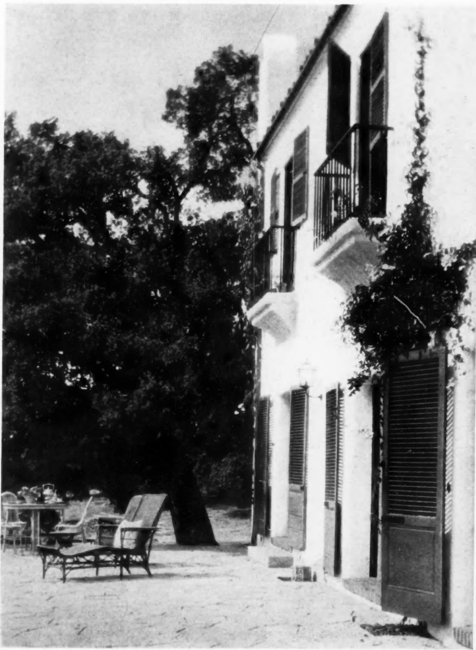
Terrace Detail RESIDENCE OF IRVING WRIGHT, ESQ., SANTA BARBARA, CALIFORNIA George Washington Smith, Architect
