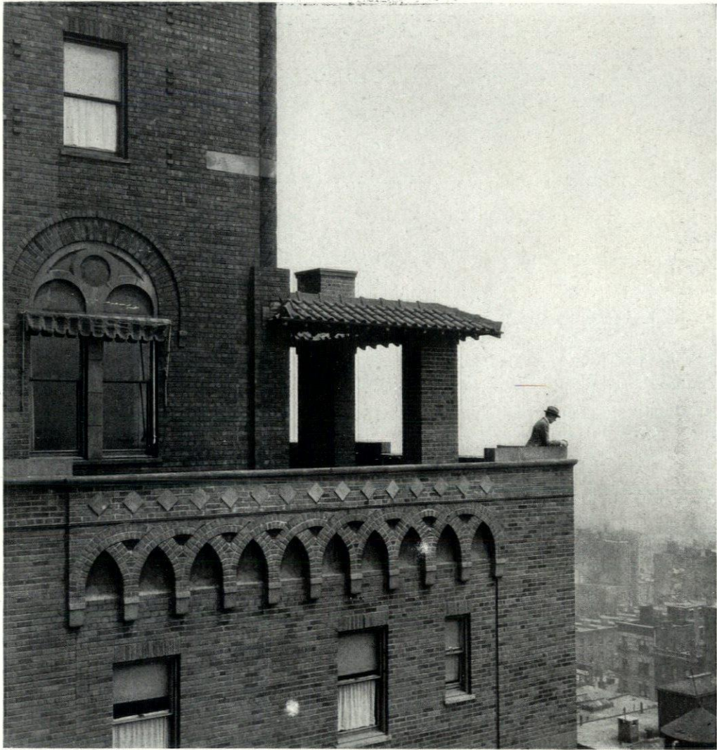
Detail at Setback of Corner Pavilion at Sixteenth Floor THE SHELTON HOTEL, NEW YORK Arthur Loomis Harmon, Architect
