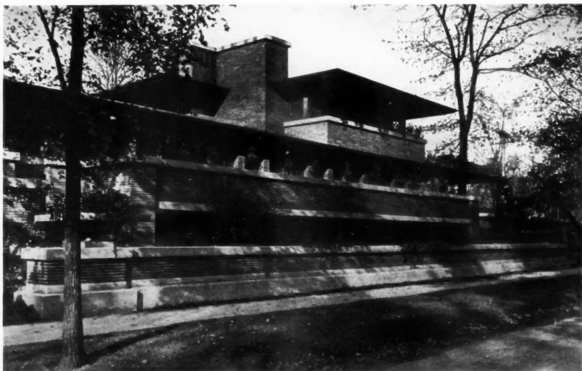
DETAIL OF BRICK WORK THE ROBIE HOME, WOODLAWN AVENUE, CHICAGO FRANK LLOYD WRIGHT, ARCHITECT
