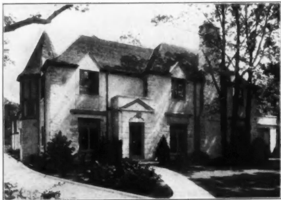
Residence of Harry W. Rubloff, Glencoe, Illinois W. D. Mann, Architect. Cabot's Quilt and Stained Shingles Used.
