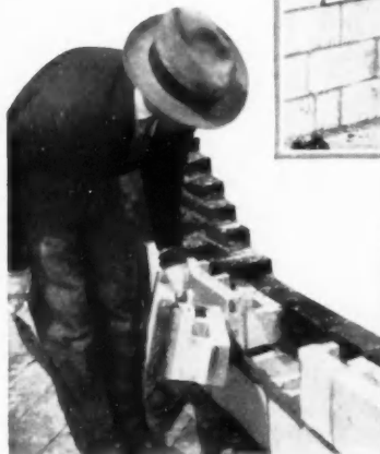
This picture shows how light weight and smooth surface of tile contribute to ease and speed of placing. Wide side walls contribute to ease of placing mortar and materially reduce mortar loss.
