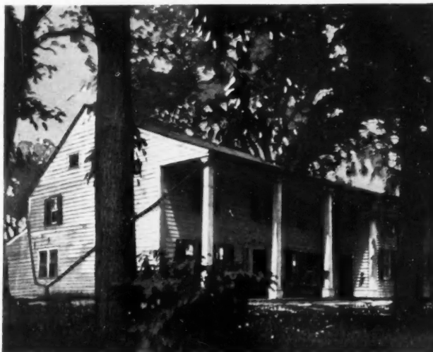
The Henry House at North Bennington, Vt. was built in 1769. The wide Pine clapboards and the porch with its square Pine columns give an atmosphere unique in old homes of the North.
