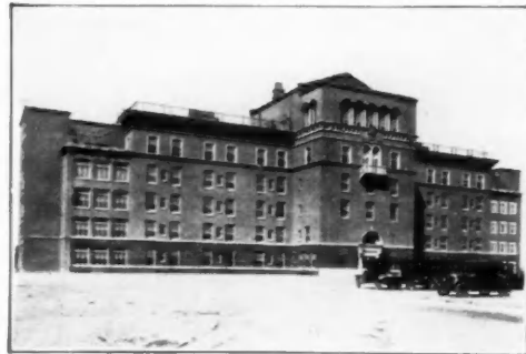
Right—Presbyterian Hospital, Denver, Col.; 8,000 sq. ft. TMB; W. E. and A. A. Fisher, Architects
