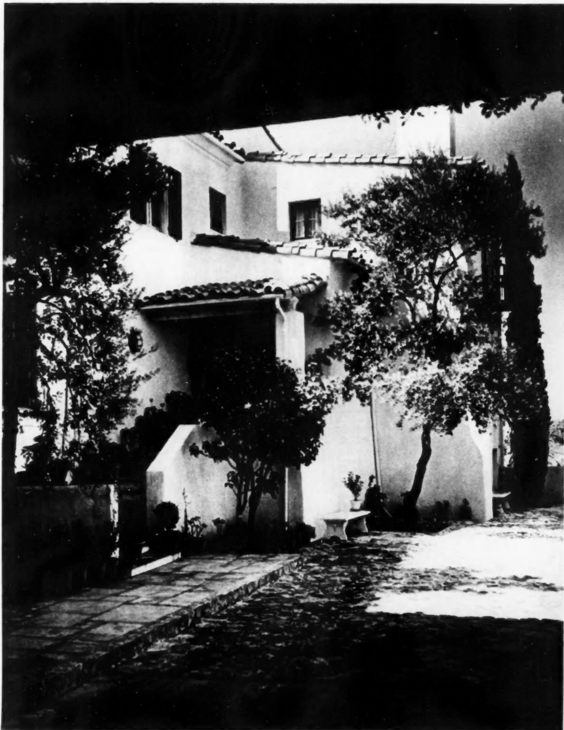
Residence of Mrs. Richard B. Fudger, Los Angeles, Calif. ROLAND E. COATE, ARCHITECT
