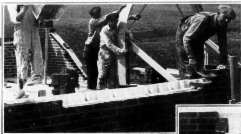
As shown in this picture, header brick bonding is easily accomplished with Structolite Tile. Practically all patterns of bonding are easily adaptable to a simplified construction without requiring continuous brick work clear through the wall.
