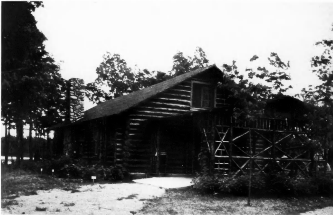
COTTAGE IN WHICH ALL LOGS AND POLES USED WERE TREATED WITH LINSEED OIL Greening's Cottage, Bitely, Michigan
