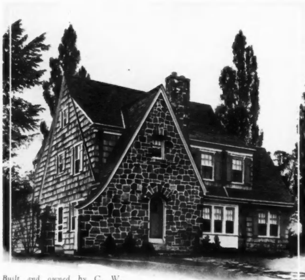
Built and owned by C. W. Hurlbut, West Hartford, Conn., from plans by Architect D. S. Douglass, WEATHERBEST Old Colony Hand Rived Shakes stained gray on Sidewalls and 18-in. dark gray WEATHERBEST Stained Shingles on the Roof.
