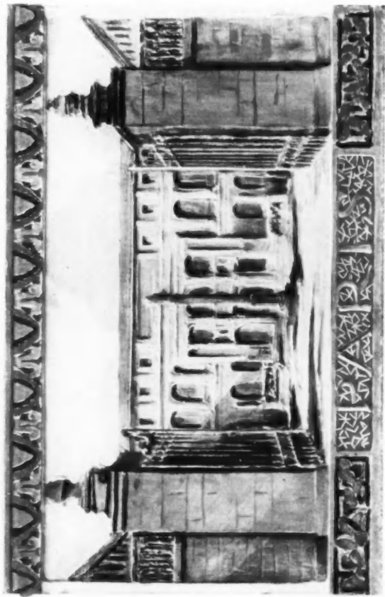
Polychrome Terra Cotta panels for the façade of the new building of the Beaux-Arts Institute of Design, New York City.
