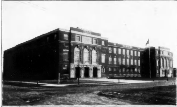
Left—High School, Baldwin, L. I.; 50,000 sq. ft. of TMB; H. T. Blanchard, Architect
