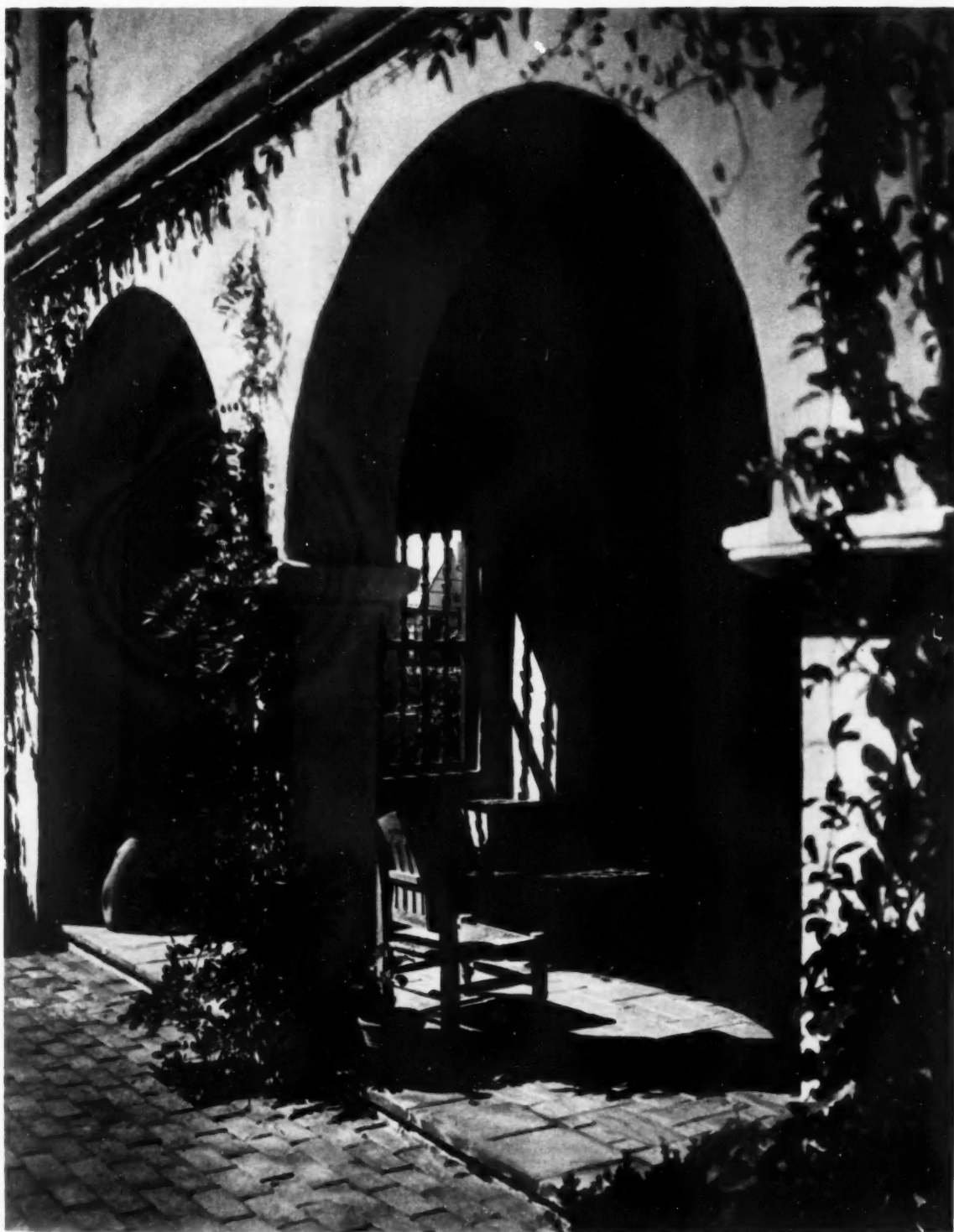
Residence of Mrs. Richard B. Fudger, Los Angeles, Calif. ROLAND E. COATE, ARCHITECT
