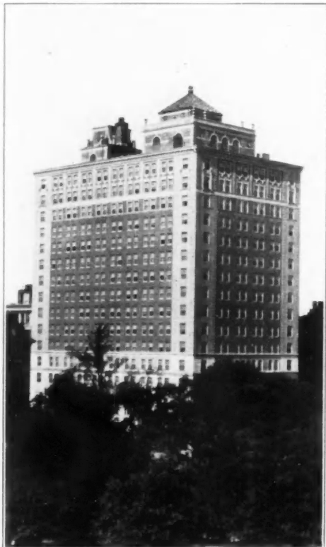
Ritz Carlton Hotel—Boston, Mass.— Chase & Gilbert, Architects
