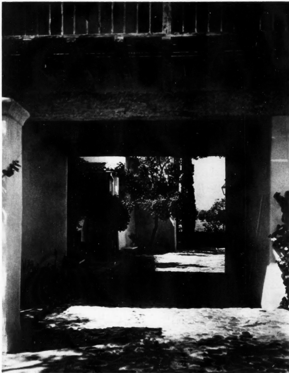
Residence of Mrs. Richard B. Fudger, Los Angeles, Calif. ROLAND E. COATE, ARCHITECT
