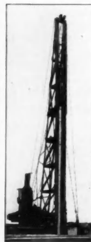
Typical All-Steel Pile Driving Equipment
