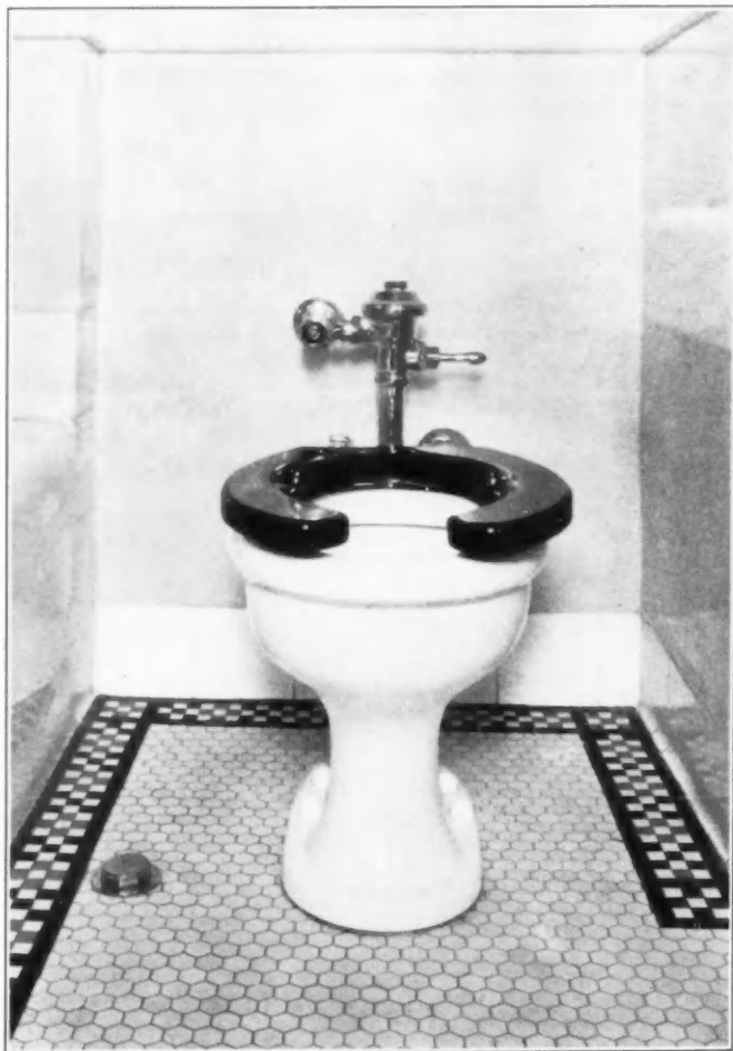
A Church Sani-Black installation in the Northampton Hotel Northampton, Mass.
