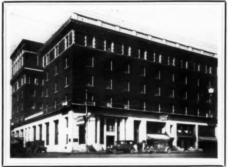
The Hotel Brodhead, Beaver Falls, Pa. Emmett E. Bailey, architect, and Harry Wimer, contractor. Trimmings throughout with RACKLE ARTSTONE, of which some thirty carloads were required. The job illustrates one of our new hand-brushed finishes, applied while the material is still plastic—the result being not only an extremely attractive texture, but enhanced density and weather-proof qualities.
