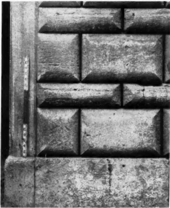
FIG. 102. DETAIL OF WALL, PALACE RONDANINI, ROME
