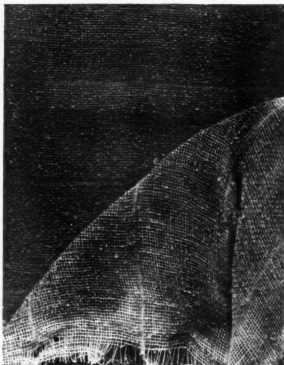
ROUGH CONCRETE SURFACE SUITABLE FOR APPLICATION OF TILE, PRODUCED BY LINING CONCRETE FORMS WITH 1/4" MESH BURLAP
