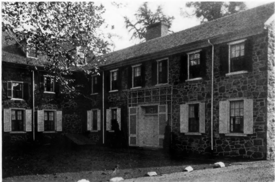
(ABOVE) WEST SIDE, FROM GARDEN. (BELOW) WEST DOORWAY "GOODSTAY", WILMINGTON, DELAWARE EDMUND B. GILCHRIST, ARCHITECT
