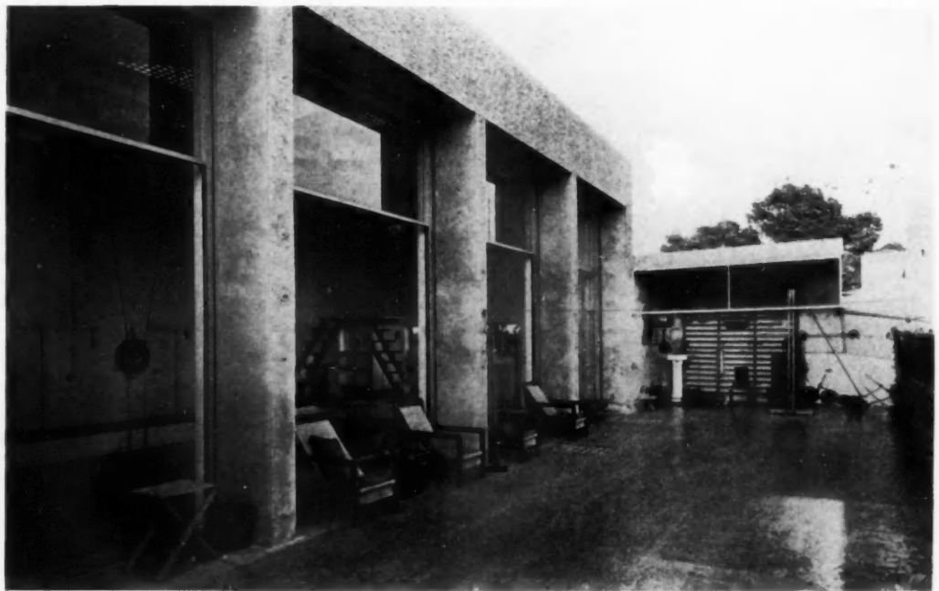
POOL WITH OUTDOOR GYMNASIUM AND BALCONY VILLA OF VICOMTE DE NOAILLES AT HYÈRES, FRANCE ROB MALLET-STEVENS, ARCHITECT
