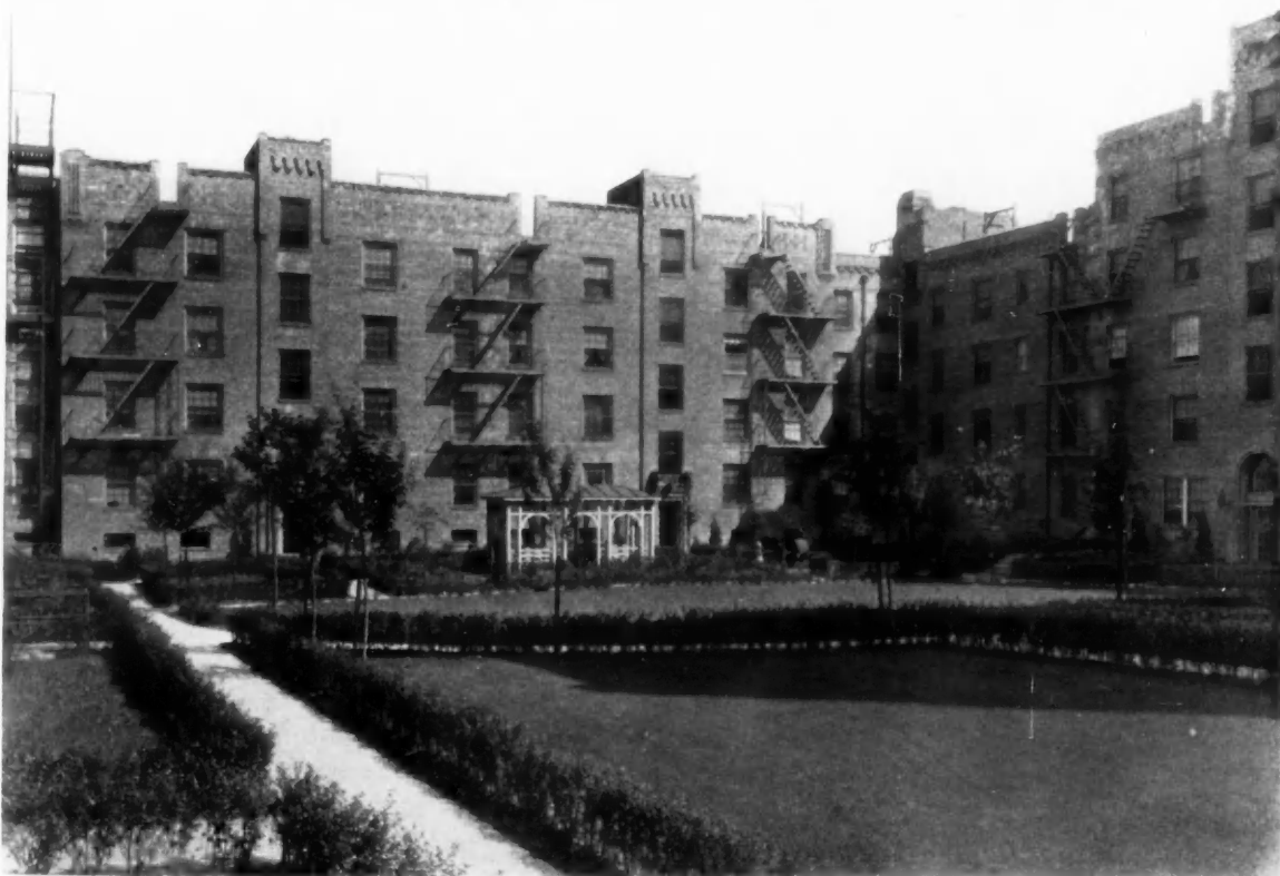
This courtyard is 130 feet square, although the building covers 49 per cent of the plot, which is 190' x 205'. It is an unusual example of simple perimeter planning and also illustrates the fallacy of overcrowding land as shown in the following pages.
