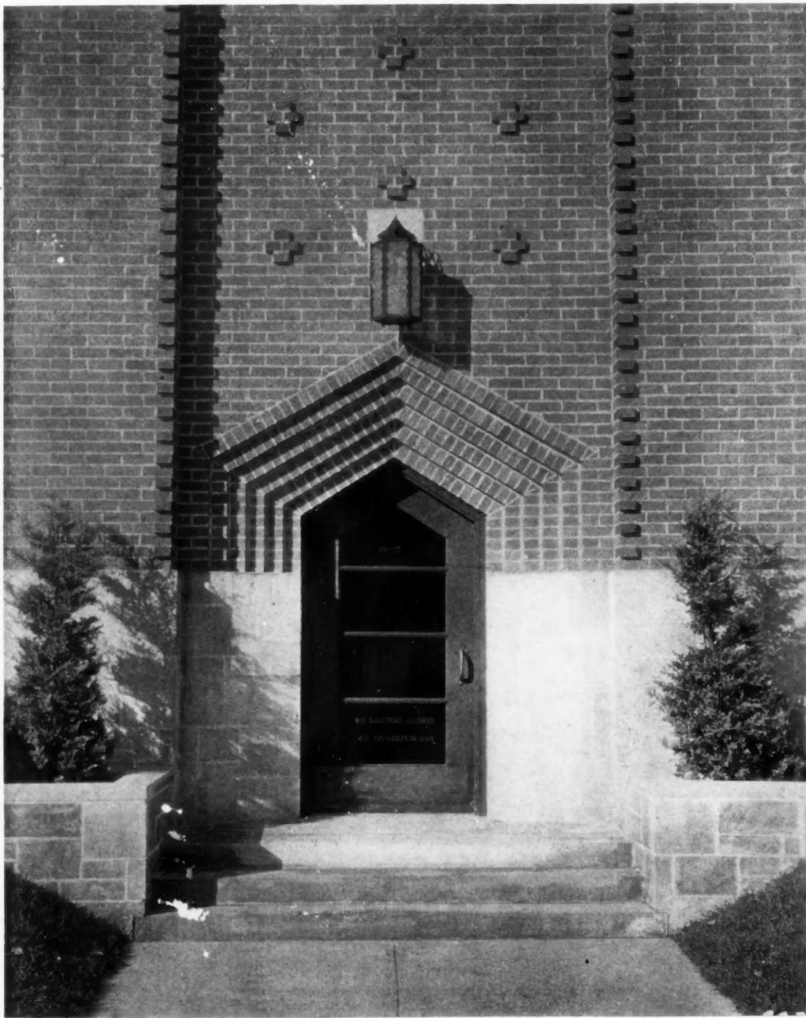
DOORWAY DETAIL APARTMENT HOUSE AT 1111 CEDAR STREET, MICHIGAN CITY, INDIANA JOHN LLOYD WRIGHT, ARCHITECT
