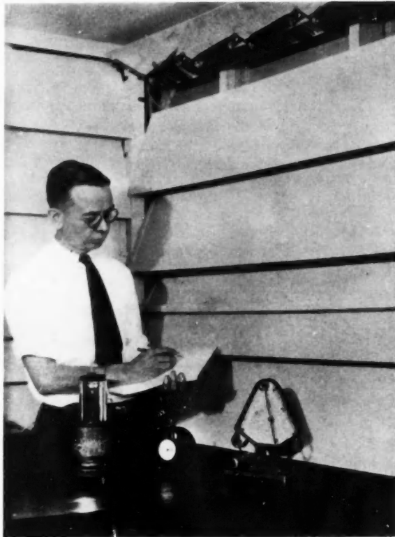
Electrically-heated panels in this windowless room control the wall surface temperature to agree with the body temperature, thus preventing loss of radiated body heat which is usually absorbed by cold walls. (A top panel is turned up to show electric units.) Humidity and air currents are controlled separately. Designed by Westinghouse.
