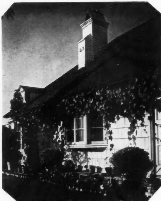
Residence at Los Angeles, California. Leland F. Fuller, A.I.A., Architect and Owner. Cabot's Old Virginia White on side walls, DOUBLE-WHITE on exterior brick, Cabot's Creosote Shingle and Wood Stains (Dark Blue) on roof.
