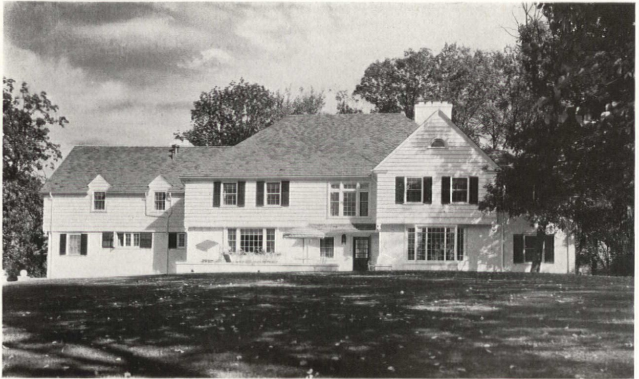
Façade Facing the Lake
