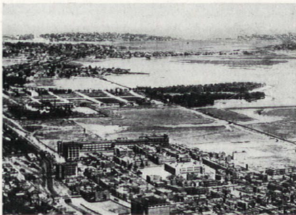
Air view of proposed site for Neptune Gardens housing development.
