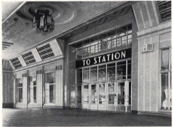
Pedestrians' entrance from incoming vehicular ramp. The entrance, windows, grilles and lighting fixtures are fabricated from light aluminum alloys.
