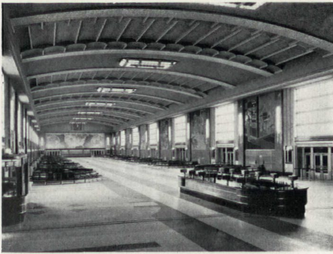
The station concourse: aluminum, mosaics, red verona marble and various shades of terrazzo.
