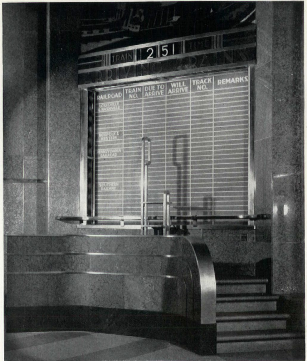
Train announcing board in station concourse: Deplated and highlighted aluminum castings, bar stock, sheet, tubing and extruded sections.
