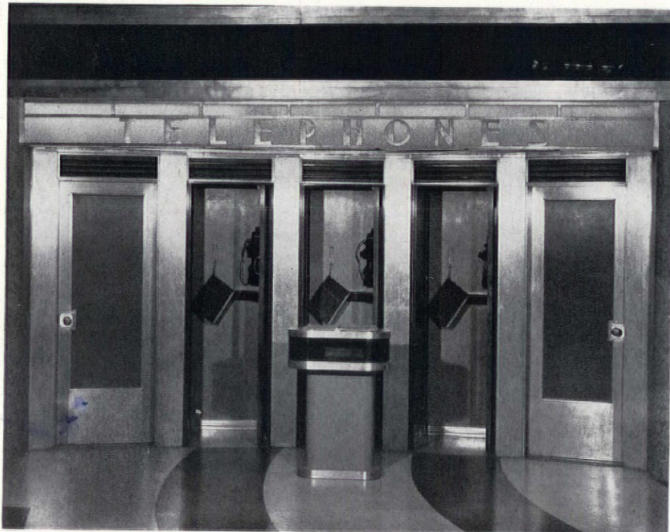
Telephone booths and employees' entrance to lunch counter and storage space at lower end of concourse. The doors are formed from rectangular aluminum tubing; the jambs and casings, from aluminum sheet. Aluminum bar, sheet and angles are employed in the lighting fixture and lettering, while the stand is trimmed with aluminum bar stock.
