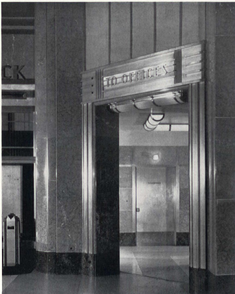
Opening between concourse and lobby to stairs and elevator. The flush panel door is formed from aluminum sheet and channel sections, the lighting fixtures from aluminum sheet.
