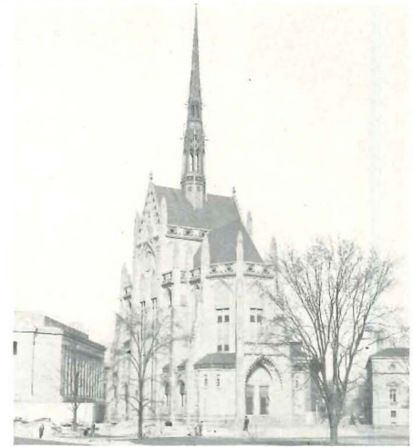
GIVEN BY THE CHILDREN OF THE late "Pickle King," H. J. Heinz, the Heinz Memorial Chapel is reminiscent of the Sainte Chapelle. Interior and exterior are of limestone; the floor is of crab orchard stone except in the chancel where Vermont green slate is used.
