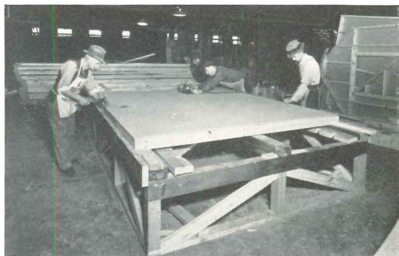
To both sides of units Homasote is fixed by means of special glue, special nails.
