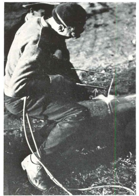
2. EXACTING CONDITIONS SPECIFY USE OF LOCKING DEVICE BEFORE WELDING. NOTE INITIAL TACKING OF PIPE.
