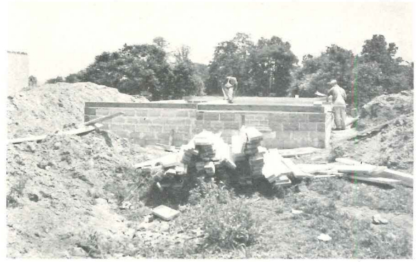
ON THE JOB: Foundations are put in, pre-cut joists set in place.
