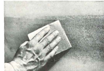
Cement is applied over Perf-A-Tape and sanded evenly, assuring a smooth surface for any decoration.
