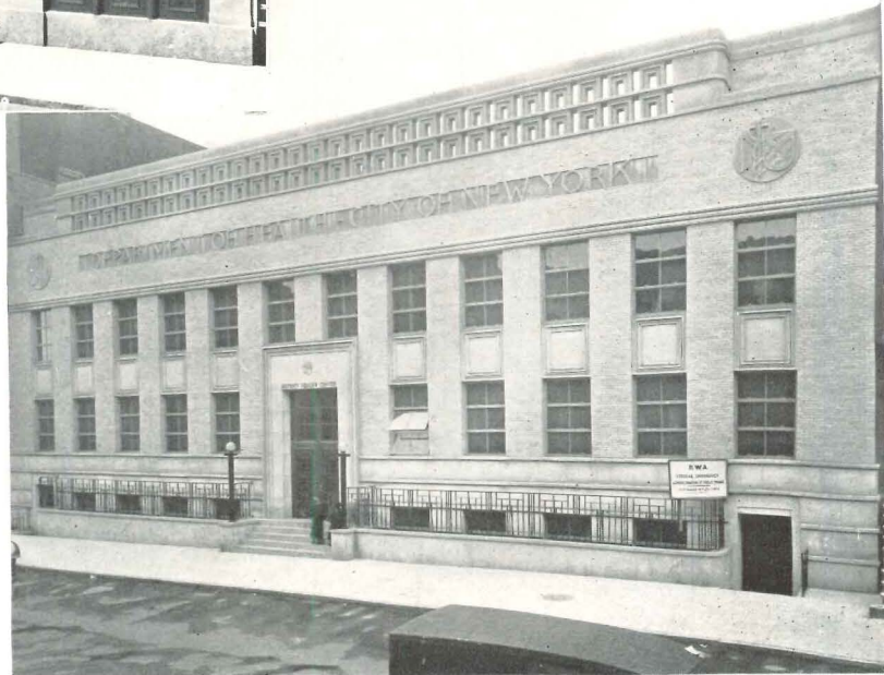
CITY OWNED AND CITY BUILT, East Harlem Health and Teaching Center replaces the first general health center built in 1921.
