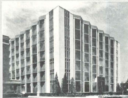
A. O. Smith Building, Milwaukee—Holabird and Root, Architects
