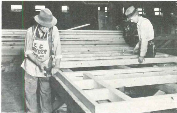
Fabrication of wall and partition units are framed from working drawings, doors and windows integral.
