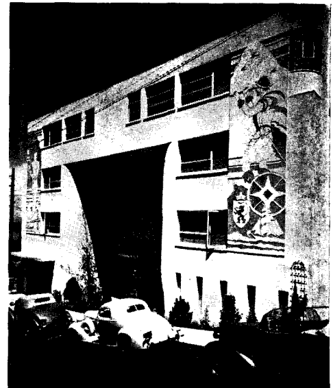
This front elevation view shows the 40-ft. sgraffito carvings, in two colors, which flank the entrance; garage entrance is at lower left.
