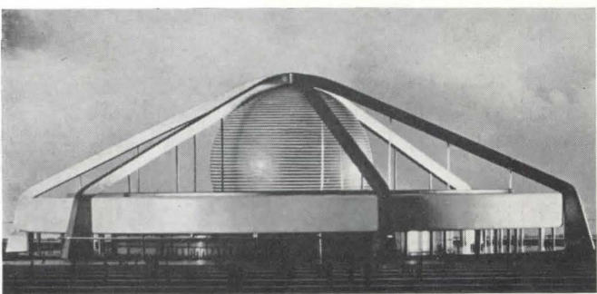
The circular form used on the proposed U. S. Government Exhibit building was determined only partially by the shape of the lot assigned to it; need for centralization and good circulation also dictated a circle.
