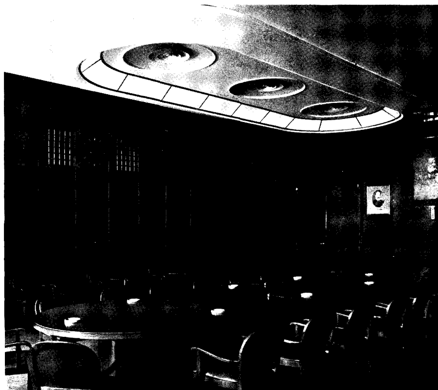
Figure 27. Installation producing a low-velocity blanket of air through use of a number of anemostats.
