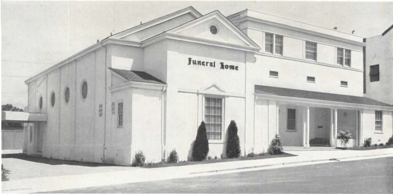
Building after alteration
