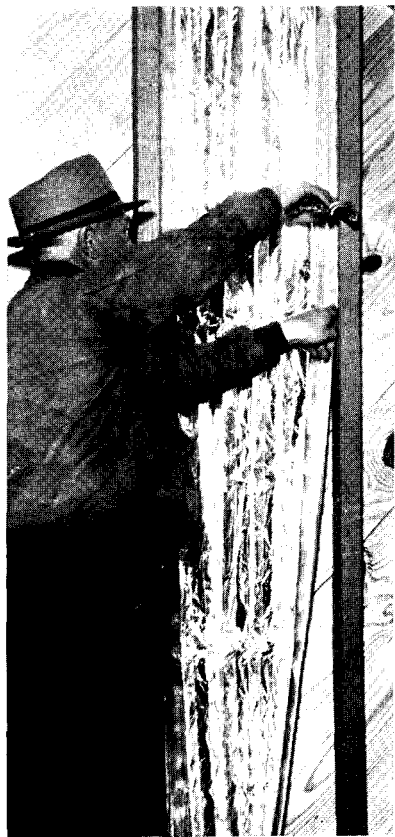
Typical installation showing relation of air space to foil.
