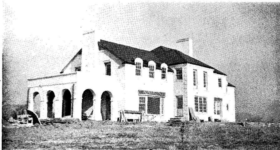
Masked by the brickwork is the welded light-steel frame
