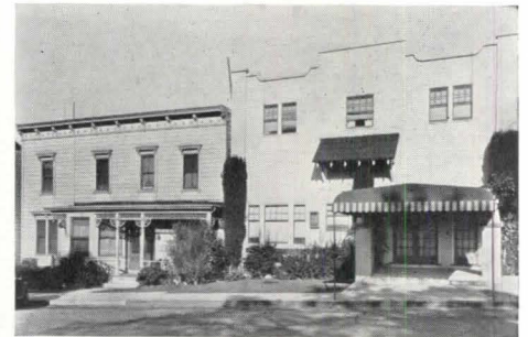
Building before alteration
