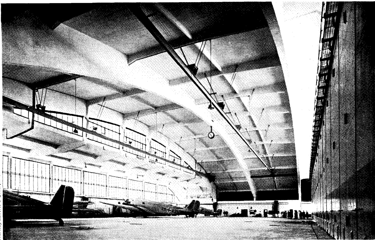
Airplane Hangar, Germany. Construction is monolithic concrete, Z-D system. Concrete shell is 4\frac{3}{4} in. thick. Span is 240 ft.
