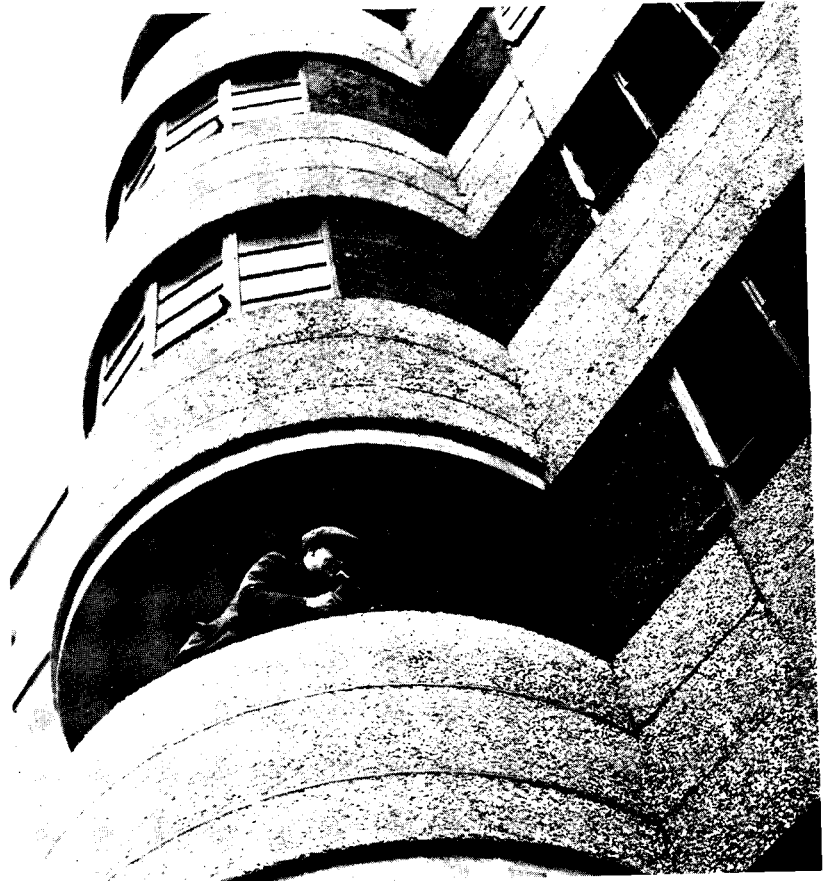
Stage 3: Finishing the exterior
