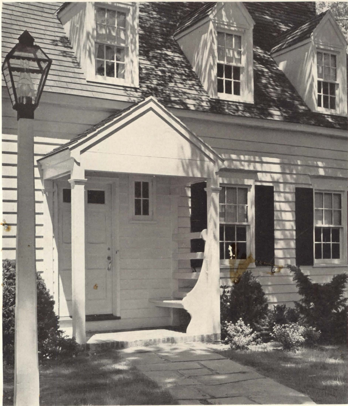
Detail of Front Entrance from the South
