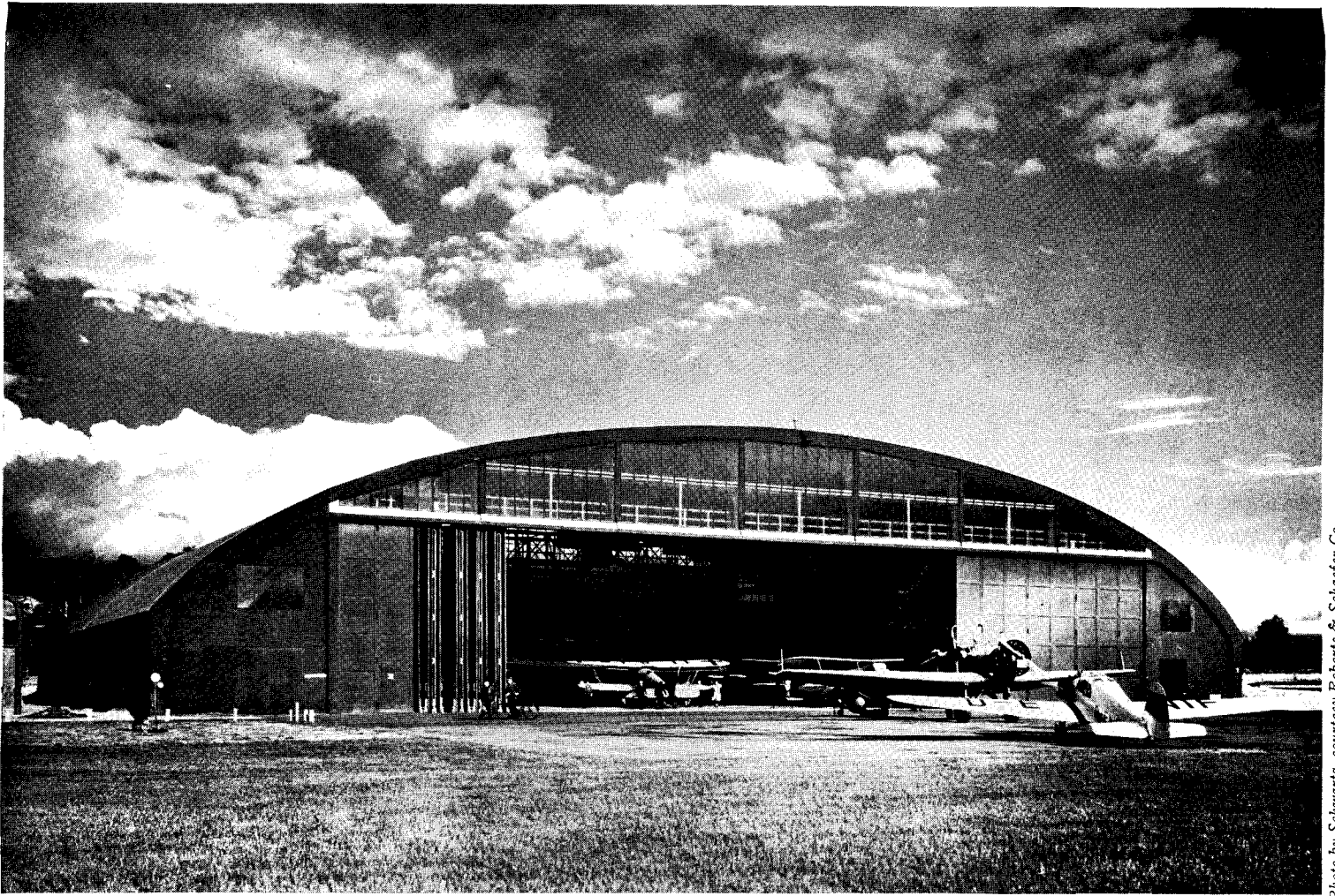
Airplane Hangar, Germany. Construction is monolithic concrete, Z-D system. Concrete shell is 4\frac{3}{4} in. thick. Span is 165 ft.
