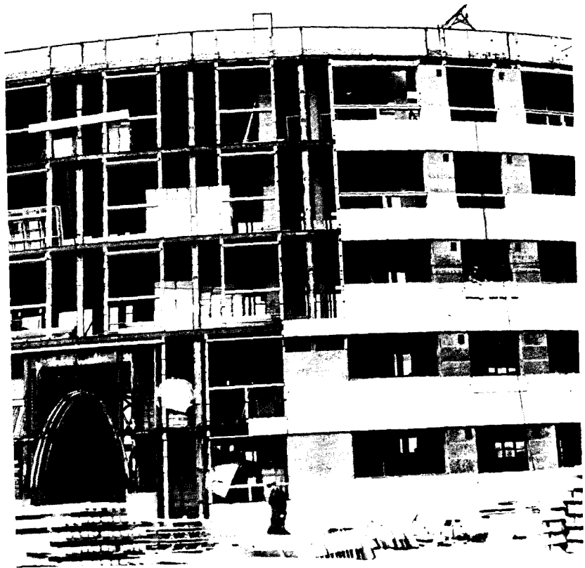
Stage 2: Concrete slabs in place
