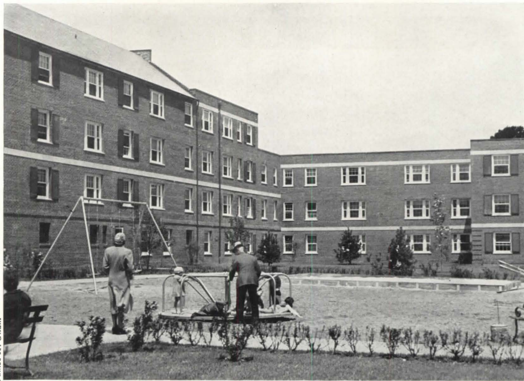
Children's play area, Brentwood Apartments, Washington, D. C.; Raymond Snow, architect. The inclusion of such areas within project sites, while not required by law, is an instance of advanced planning favored by FHA because it helps to defer obsolescence and hence aids in protecting mortgages.
