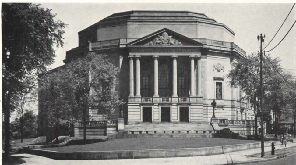
Severance Hall, home of the Cleveland Symphony Orchestra and one of the Wade Park group of cultural buildings
