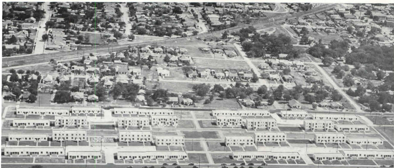
Community and site relationship in a government housing project in Dallas, Texas
