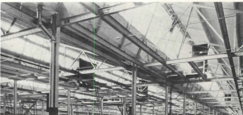
Sawtooth roof design and riveted construction common to many industrial structures
