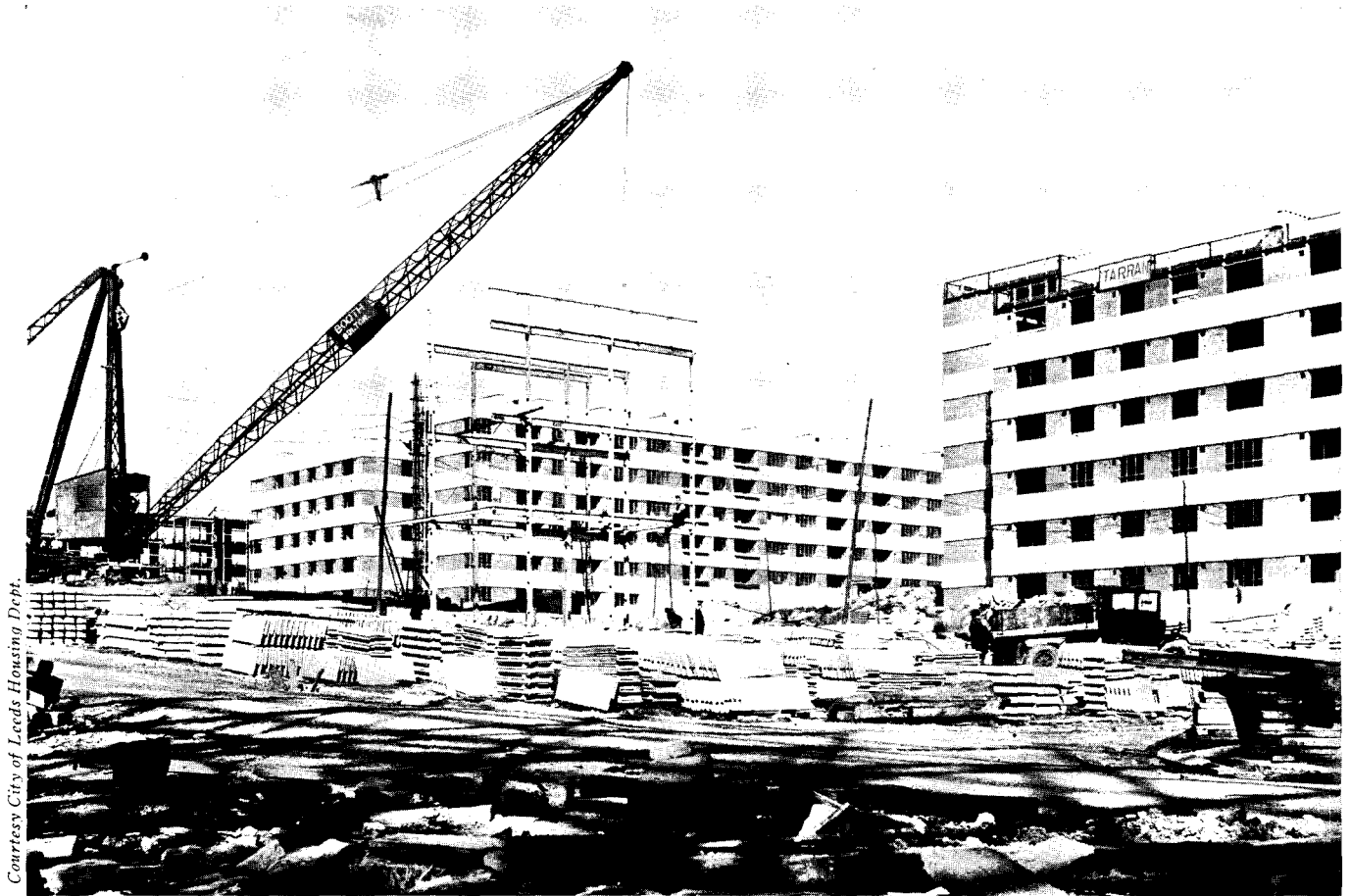
Concrete units ready to be raised to position; the units are supported on vertical posts notched to receive them.
