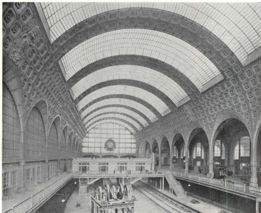
Fig. 2. Architect M. V. Laloux's Orleans Station in Paris, begun in 1898.
