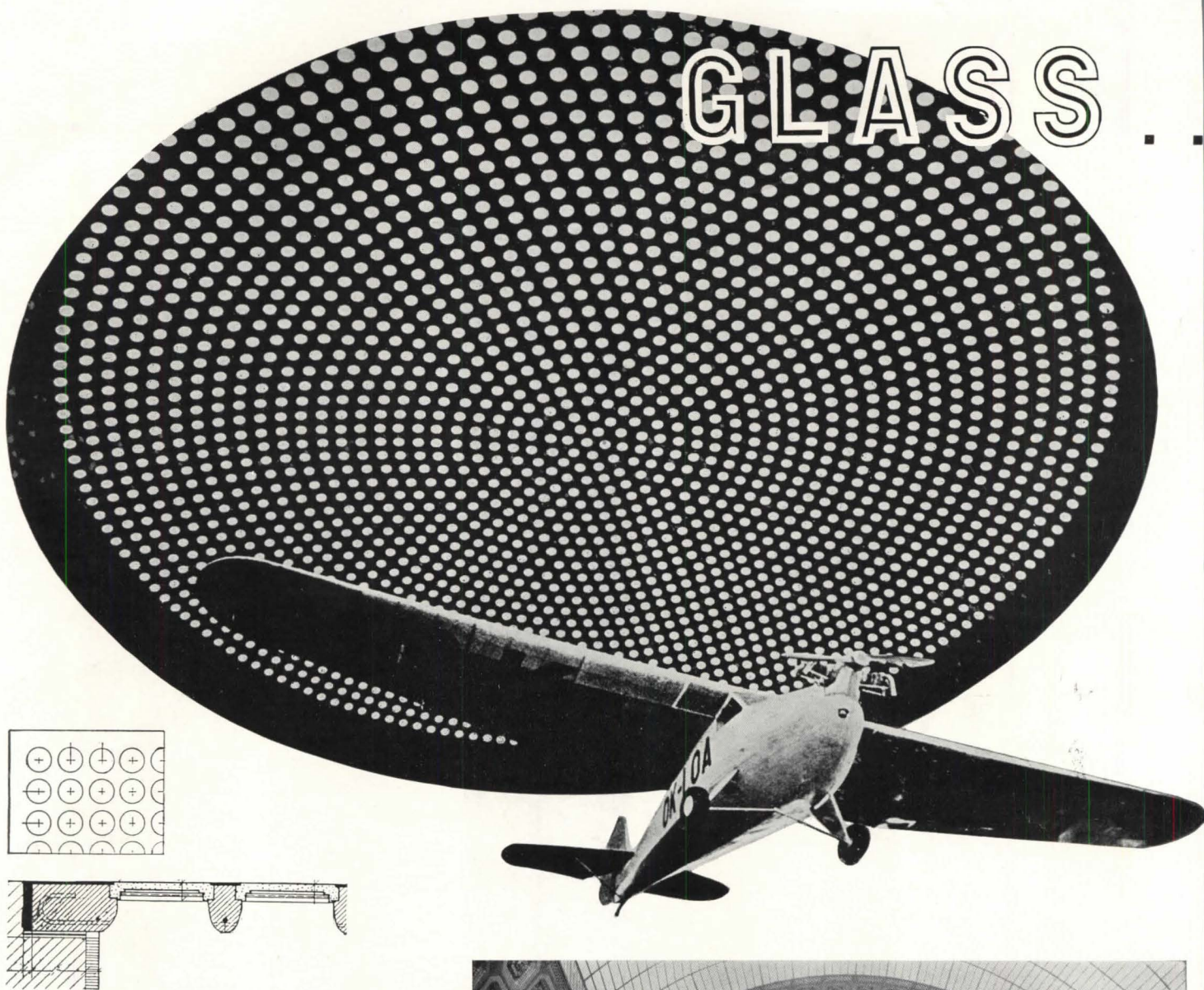
Fig. 1. Interior of Polivka's dome for the Czech Pavilion, Paris, 1937. With a 50-ft. diameter and an over all thickness of only 3 \frac{1}{5} in., this dome was built in place on special forms. Figs. 9 and 10 show similar construction.
