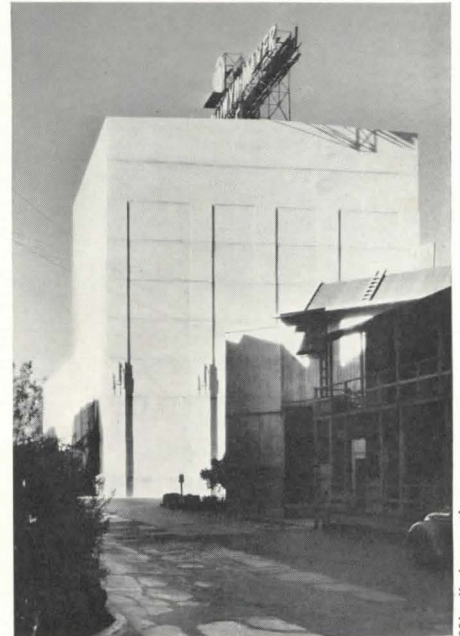
An old-type sound stage; the walls of the structure are solid concrete and insulation is proportional to wall thickness.
