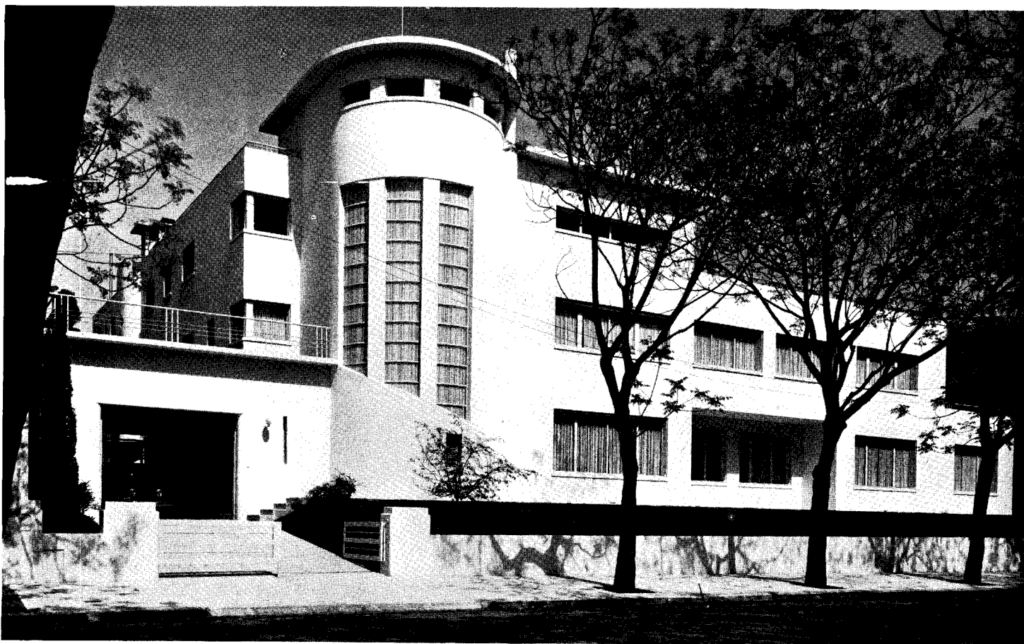
View from the street. Auto entrance at left with direct access to living and dining rooms and stairway to upper floors.
