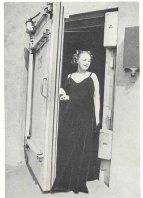
Pedestrian door of one of the new sound stages. No single door can provide insulation value equal to that of stage walls: a pair of doors, with a 5-ft. air space between them, is provided.
