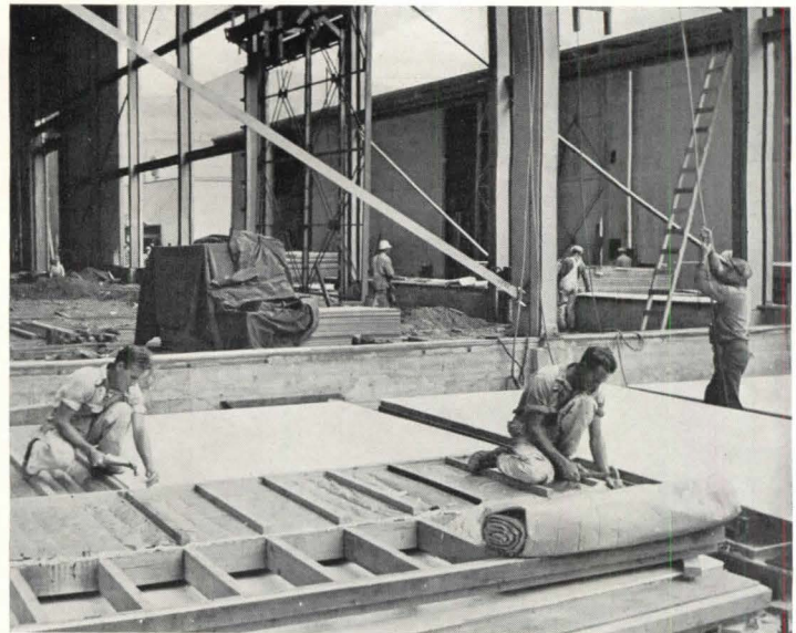
2. Wall panels are prefabricated on the ground. . . . .
