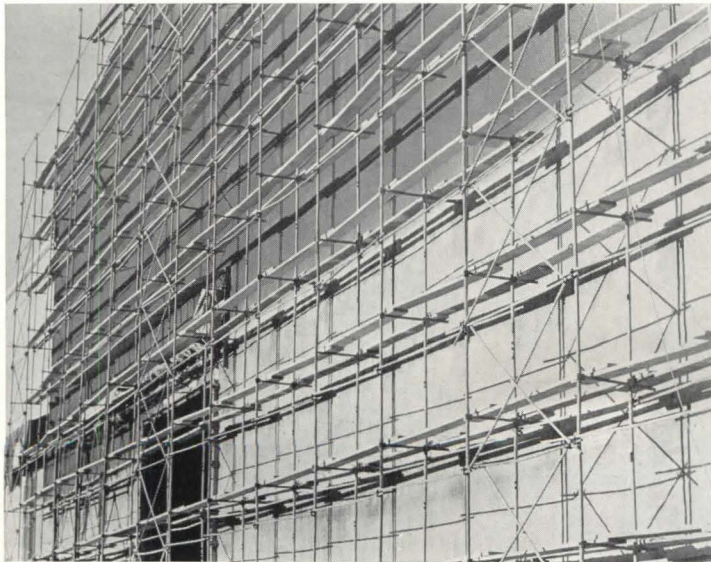
5. From the outside scaffolding, Gunitite plaster is applied. . .
