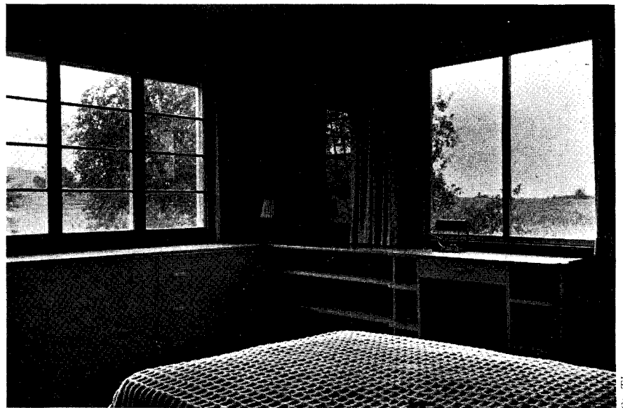
Sash can be slid back, permitting full use of window space for ventilation.
