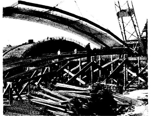
Section of arch reinforcing is picked up by crane for placing on arch centering.
