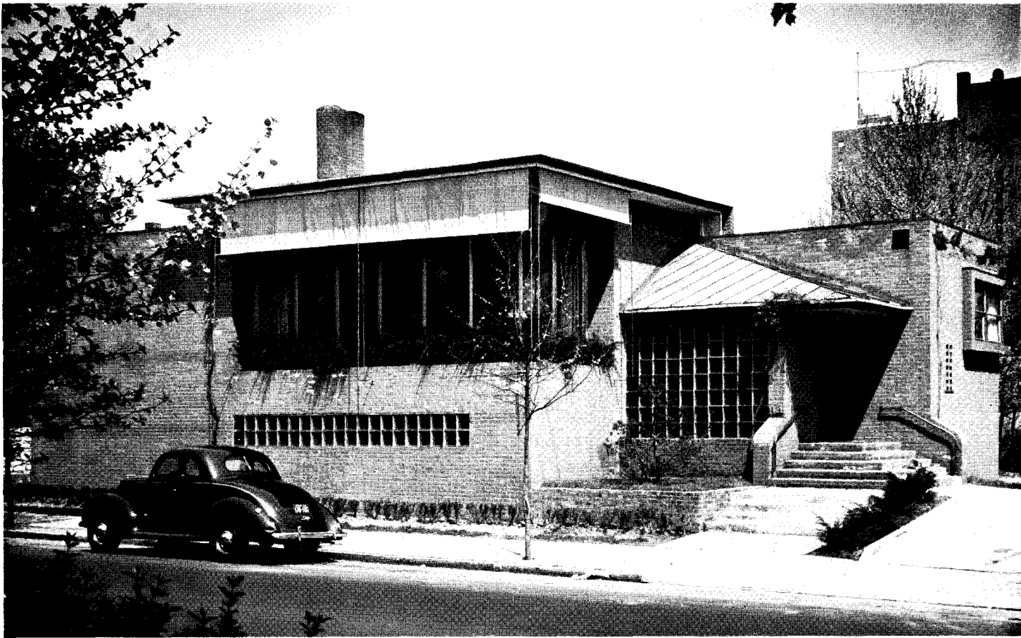
For greater privacy, working areas are elevated above street level. The awnings may be raised or lowered from within.
