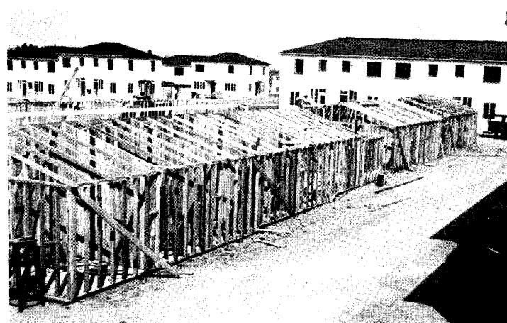
On the monolithic floor, wood-framed garages were built, following construction methods similar to those for dwelling units.
