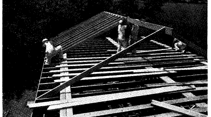
2 p.m. Nailing rafters; sheathing and shingles over.
