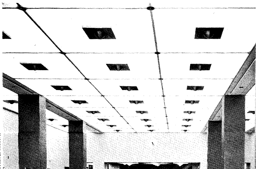
Lamps are concealed in holders in coffers, with sprinkler-heads at corners.
