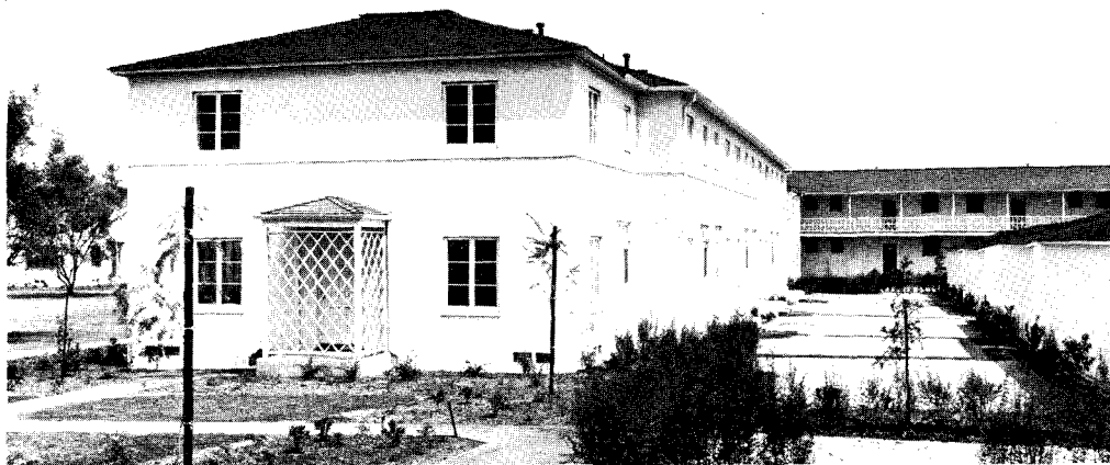
Typical exterior, showing accessibility of garage compounds whose walls form rear boundaries of private yards. Note also balcony for second-floor access.
