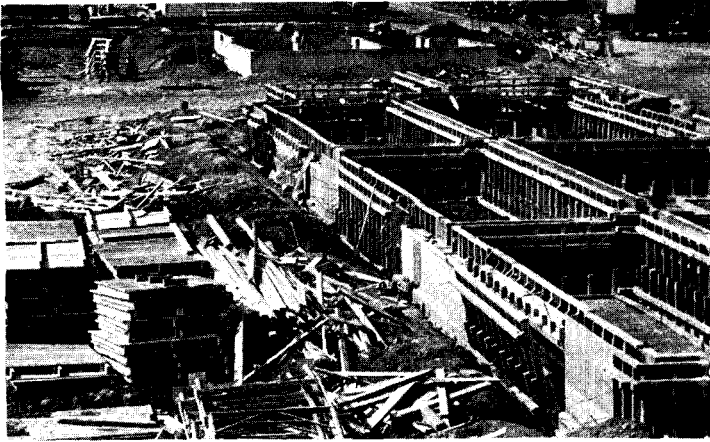
Formwork for concrete foundations was sectional; as fast as sections were stripped from one building they were set up for another.
