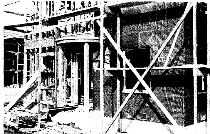
Sisalkraft paper and lath for exterior stucco were applied directly over the stiffened framing, omitting sheathing.
