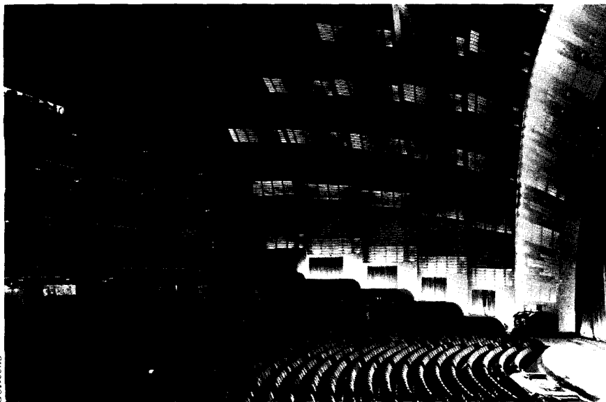
Ceiling arches designed for sound reflection also house concealed lighting.
