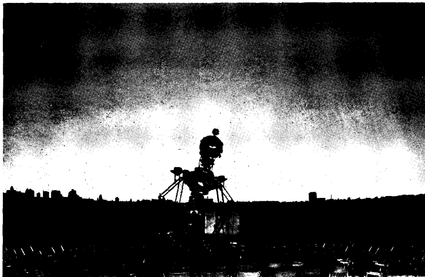
Fels Planetarium: the dome had to be spherical and highly light-reflective, but should reflect sound scarcely at all because of "focusing".
