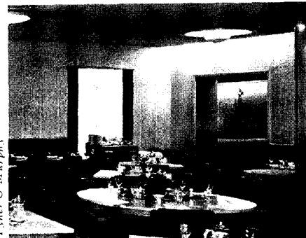
Combined air and lighting sources, Union Station, Kansas City; R. J. Raney-Holabird & Root, architects.
