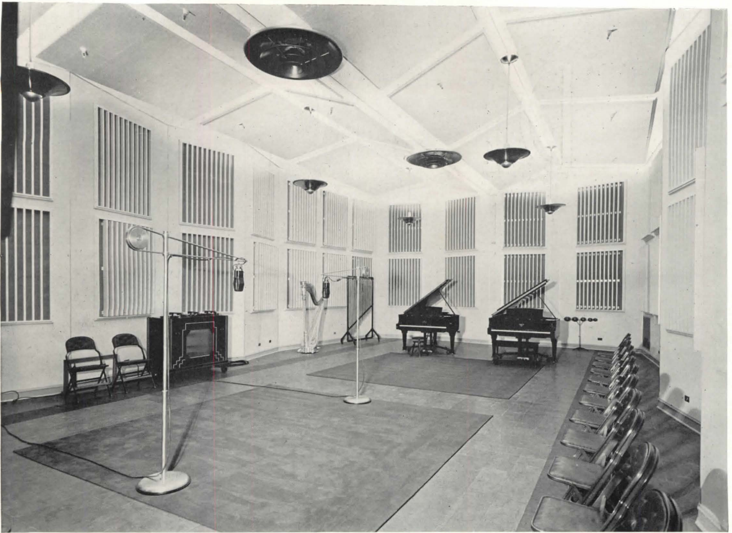
R.C.A. phonograph-recording studio: the reverberation period is controlled by operable louvers with sound-absorbent materials behind them; by opening or closing the louvers it becomes possible to vary reverberation to suit any type of recording.
