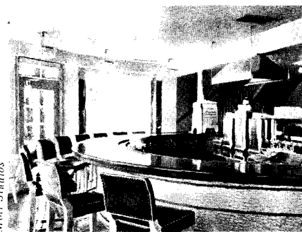
Exhaust over coffee urns, Carl's Viewpark Restaurant, Los Angeles; W. L. Schmolle, architect.
