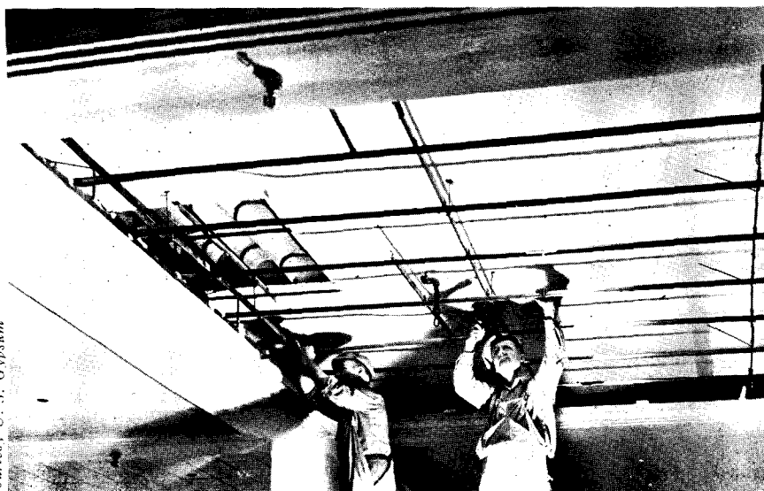
Integration of sound control and air conditioning: space between structural and suspended ceilings is a plenum; air passes through perforated-metal pans.
