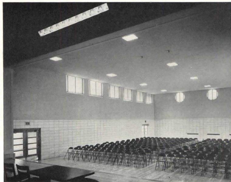
A wainscot of National Fireproofing 8 by 16-in. tile rims the auditorium.
