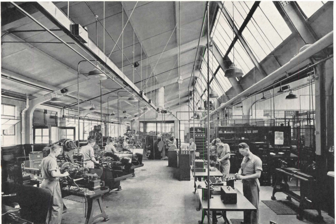
North-light monitors, continuous wall glazing, and structural steel design provide extraordinary daylight conditions.
