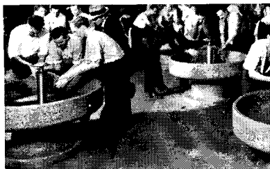
Section of the Norton Co., Worcester, Mass., washroom
