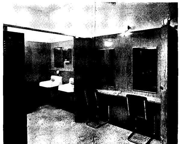
Women's locker room, Monarch Machine Tool Co.; Schenk & Williams, architects.
