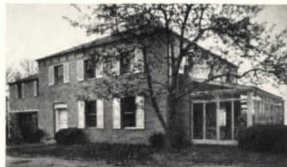
West Dodd also installed the lightning protection system on the Fire Safe House sponsored by the Home Insurance Company and featured at the New York World's Fair.
