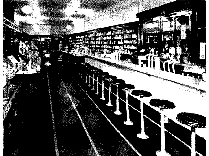
Here's a floor that helps draw trade the length of the store. It's Sloane-Blabon Plain Linoleum with inset borders and directional lines.
