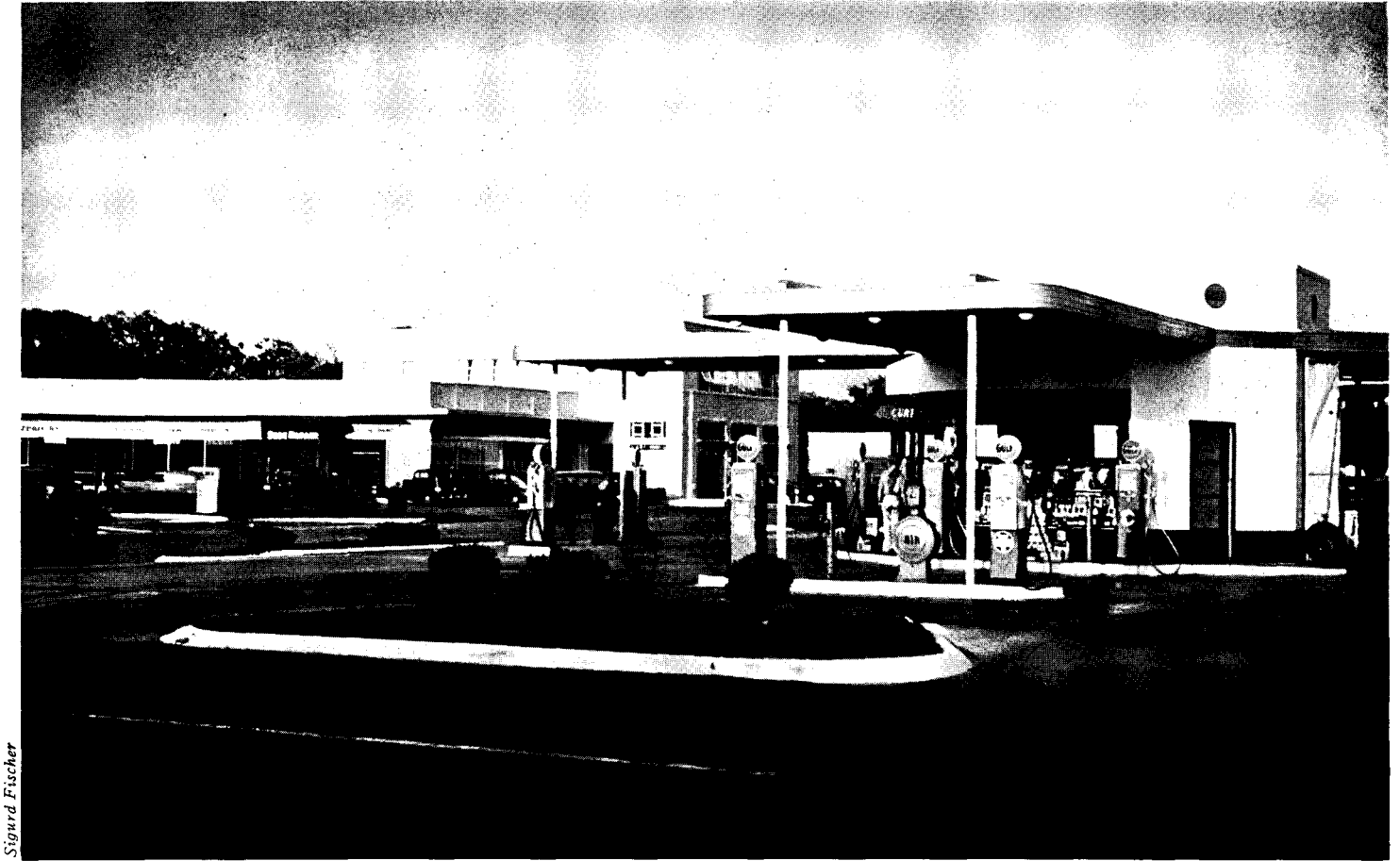
Gasoline stations are designed to offer minimum obstruction to visibility.
