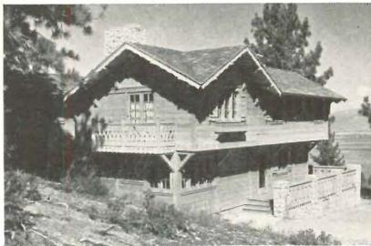
Cabot-Stained house, Minden, Nevada Architect: Russell Mills, Reno, Nev.
