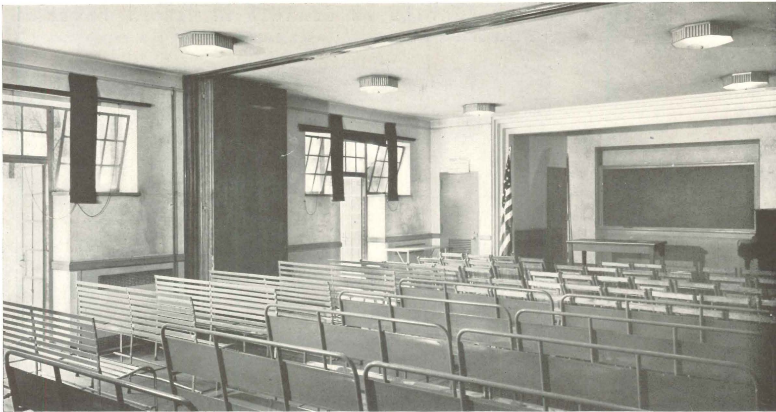
Auditorium of the Red Hook-Gowanus Center has direct access from the street through a separate entrance and courtyard, with elevator service to the first floor. Folding partition is used to subdivide auditorium into smaller rooms for conferences. Glazed doors open into rear yard and provide ample natural lighting.
