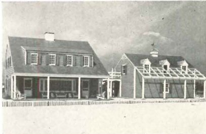
Cabot-Stained house, Beach Haven, N. J. Architects: Savery, Scheetz & Gilmore, Phil.
