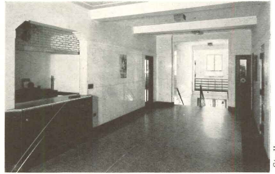
Information desk in main waiting lobby
