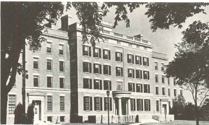
FOURTEEN NOMINATIONS: Munro Hall, College for Women, U. of Rochester; W. G. Kaelber and L. A. Waasdorp, Architects
