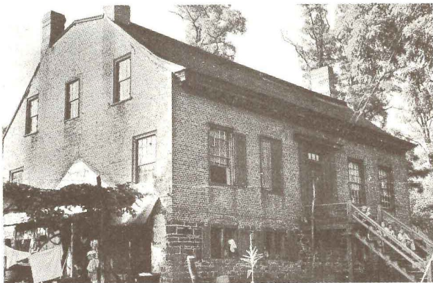
(27) Abraham DePeyster House, Beacon, N. Y., c. 1750. Typical Dutch story-and-a-half in brick on stone basement. Georgian detail
