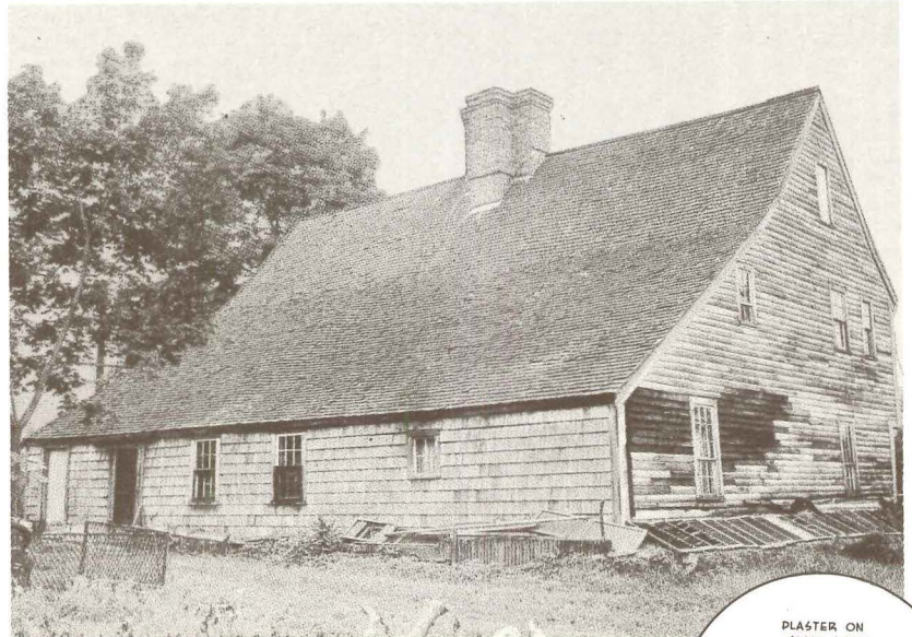
(5) "Scotch" House, Saugus, Mass. Two-story front block built in 1651 for Cromwell's prisoners sent to work bog iron. Typical heavy-timber frame (6), brick-filled and clapboarded; framed overhang; pilastered chimney. Lean-to added later
