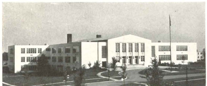
COMMUNITY BUILDING, primarily an elementary school . . .
