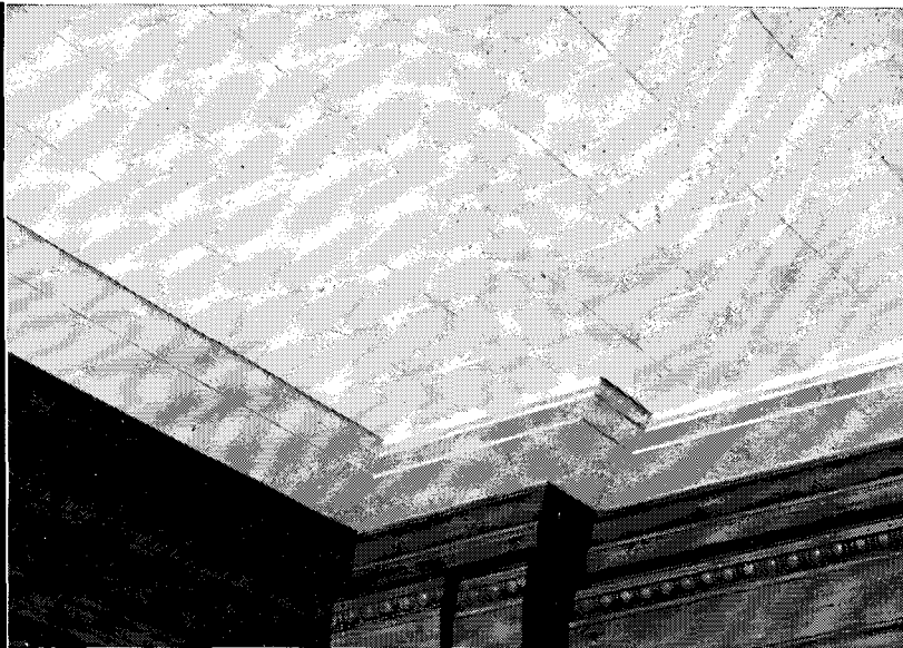
ABOVE: A 12" x 12" Permacoustic unit, white finish. Note its interesting stone-like texture. RIGHT: Close-up of a typical Permacoustic installation.
