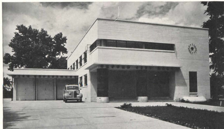
And here is another type of building necessary to "health and safety" of civilians. This is the City Hall and Fire Department, Oxford, Miss. James T. Canizaro, architect
