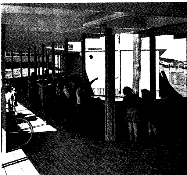
leading from administration building to classroom units
