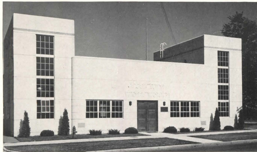
Another recent building done in concrete, this one in precast architectural slabs. It is the Faribault, Minn., water filtration plant. Long and Thorshov, architects
