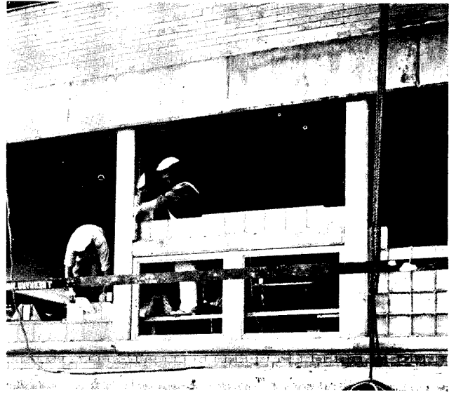
Precast concrete mullions and lintels (details below) were developed to speed the installation of large areas of glass block between stone sills and reinforced concrete spandrel beams
