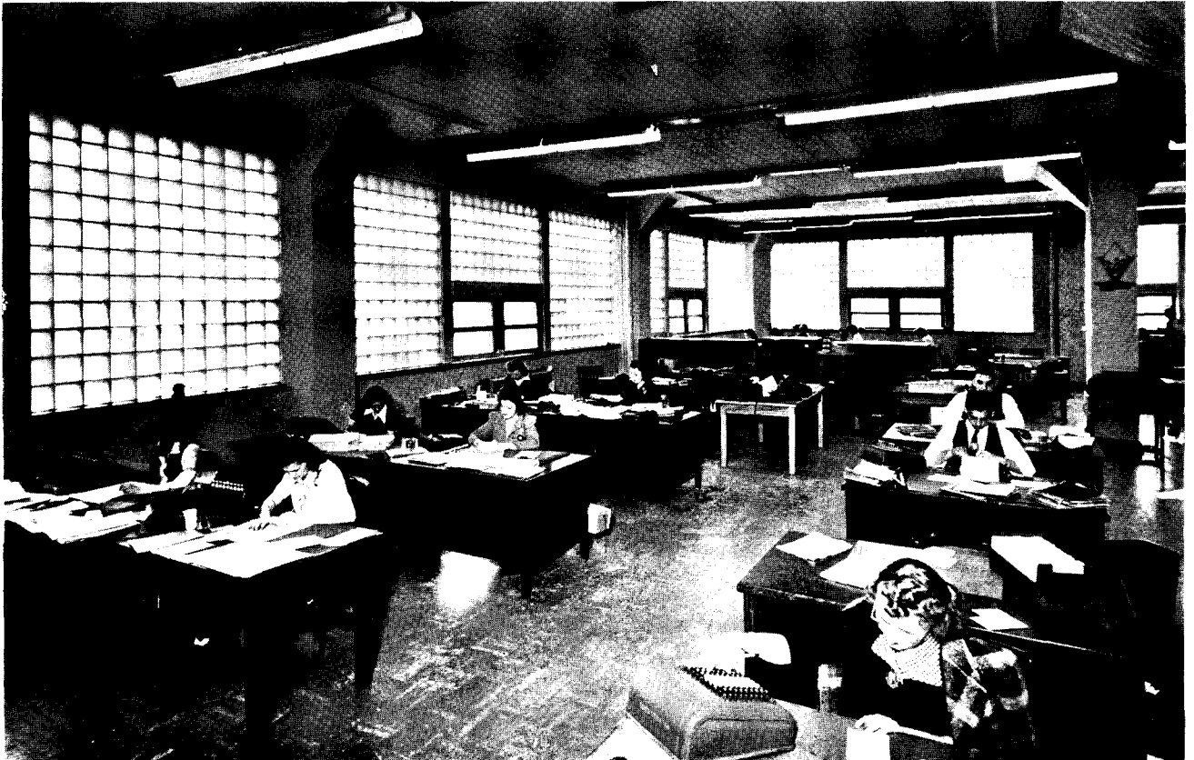
Small panels of clear glass block and small window sections give workers in offices and factory areas a chance to see out
