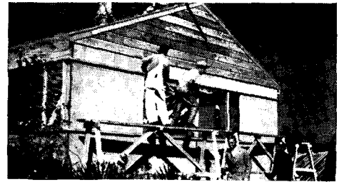
Because Cemesto handles easily, houses go up fast, are ready for occupancy in a hurry.
