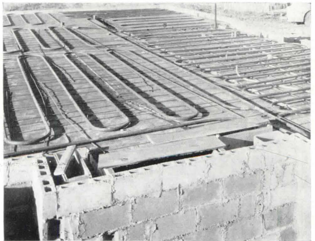
Pipe coils anchored in place above the reinforcing bars and ready for the fill and concrete to be poured
