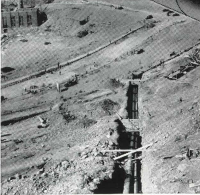
Line of Ric-wiL conduit from anchor to boiler house (top, left). Note shallow, narrow trench. Installing connector band. All necessary accessories are prefabricated and shipped with order.
