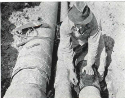
Line of Ric-wiL conduit from anchor to boiler house (top, left). Note shallow, narrow trench. Installing connector band. All necessary accessories are prefabricated and shipped with order.
