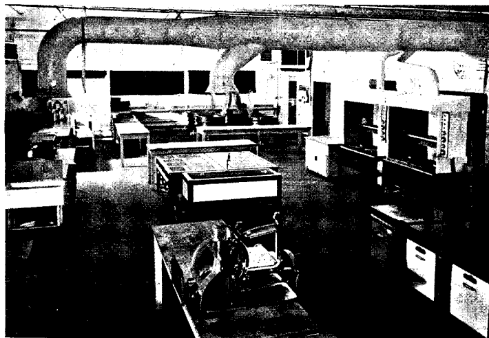
Kitchen is ventilated by exhaust ducts and fans in gable ends
