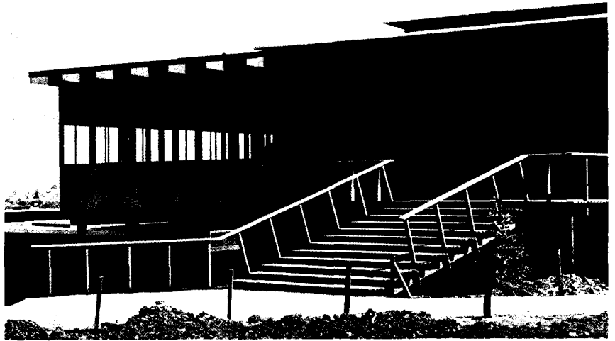
Hillside Dormitories, Vallejo, Calif. Right, entrance to coffee shop; below, dining room. Vernon DeMars, F.S.1 Architect; Norman Fletcher, Associate
