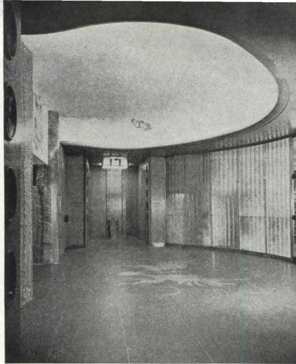
Fifth floor lobby (above) has cast glass screen partitioning in a blue-green tone, clear glass panels in doors to the law library. Floor is of black terrazzo
