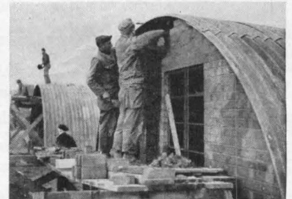
Two GI's bricking in the end of a hut
