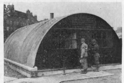
GI finishing touches and GI approval
